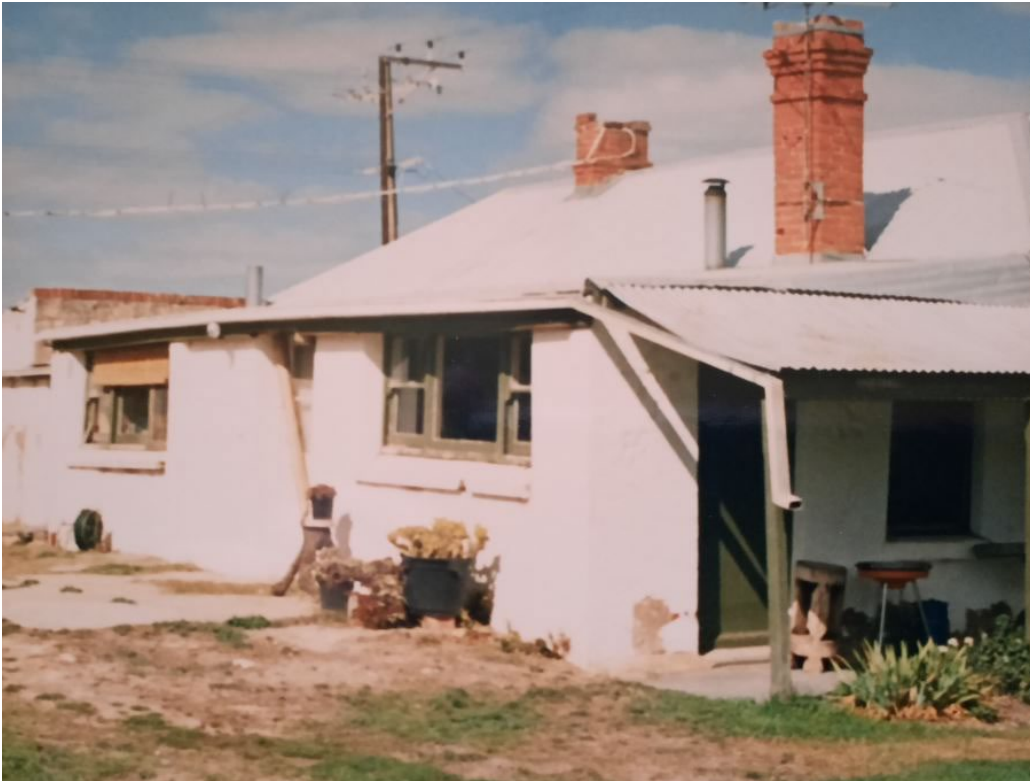
Lean-to additions to 190 Flour Mill Road, Aldinga, now demolished (courtesy of current owner)
