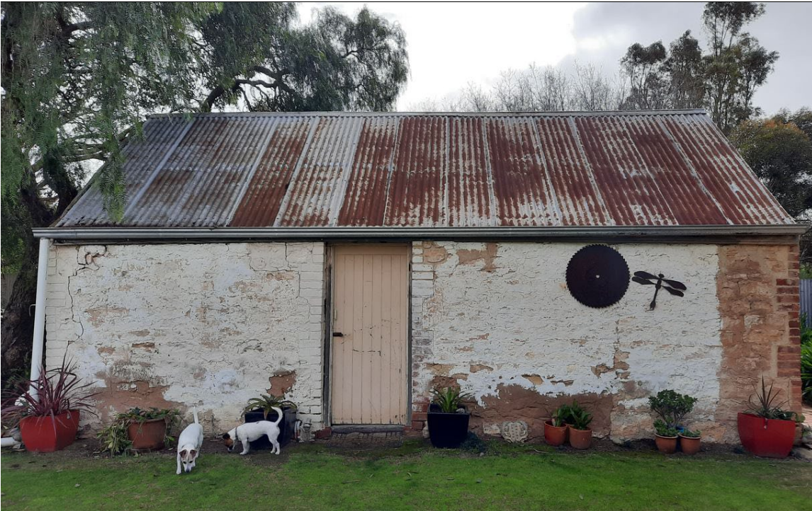
South elevation of early masonry outbuilding at 190 Flour Mill Road, Aldinga (GGA 2021)
