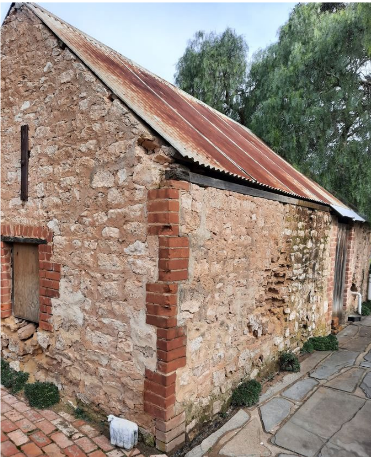
North & east elevations of early masonry outbuilding at 190 Flour Mill Road, Aldinga (GGA 2021)
