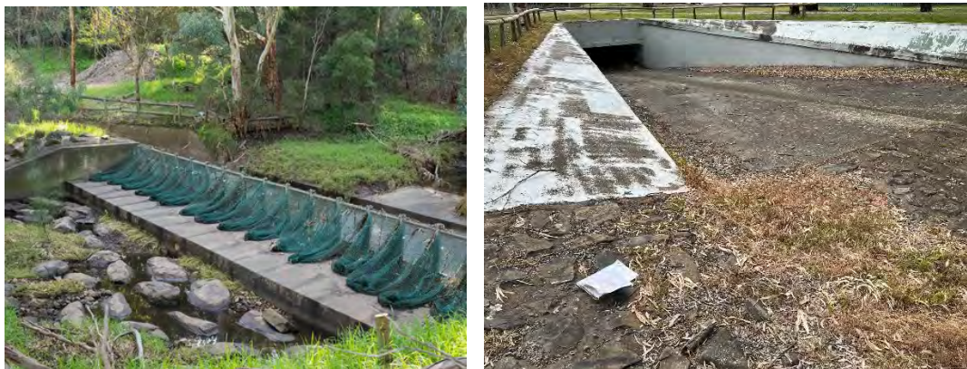
Figure 8 Typical litter net arrangement and the concrete apron at Byards Road
