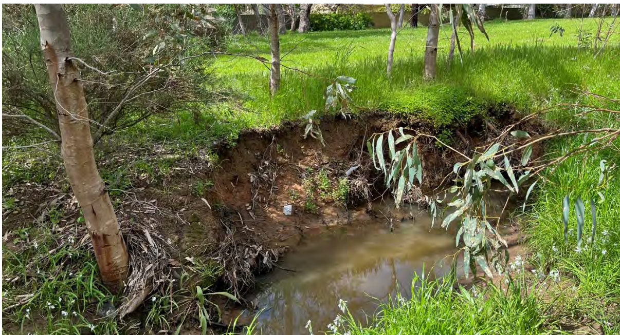
Figure 4 Example of isolated bank erosion (Panalatinga Creek)
