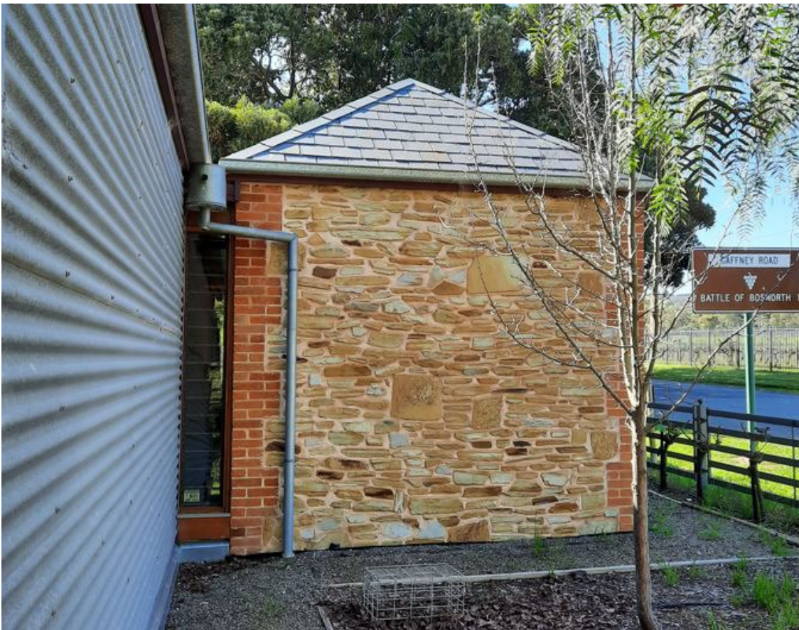
Reconstructed masonry fabric to west elevation with c.2000 additions (GGA, 2021)
