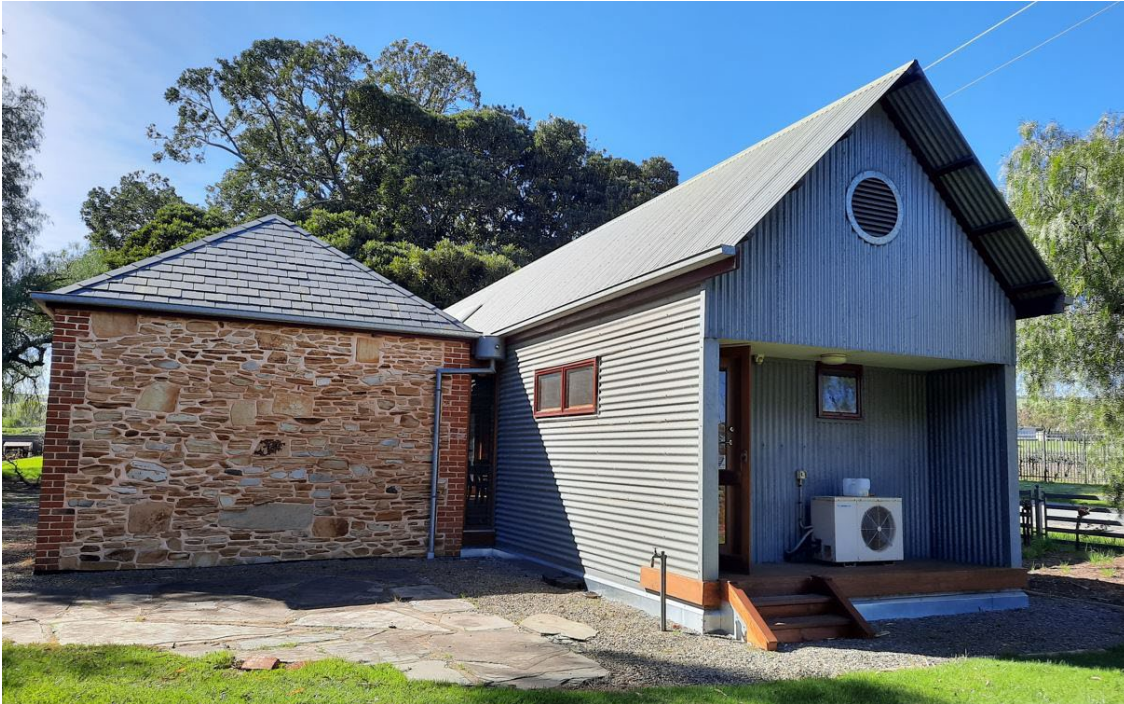
Reconstructed masonry fabric to west elevation with c.2000 additions (GGA, 2021)
