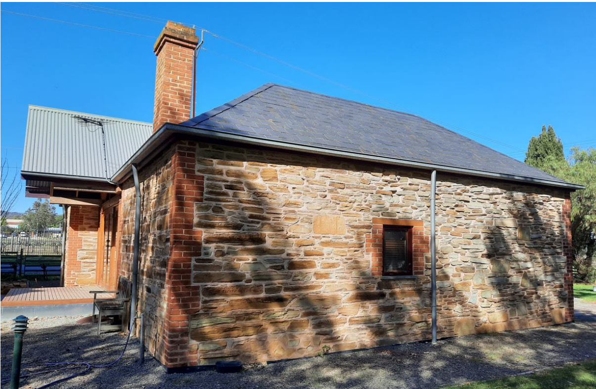
North elevation of former farmhouse, having been extensively reconstructed with additions in c.2000 (GGA, 2021)
