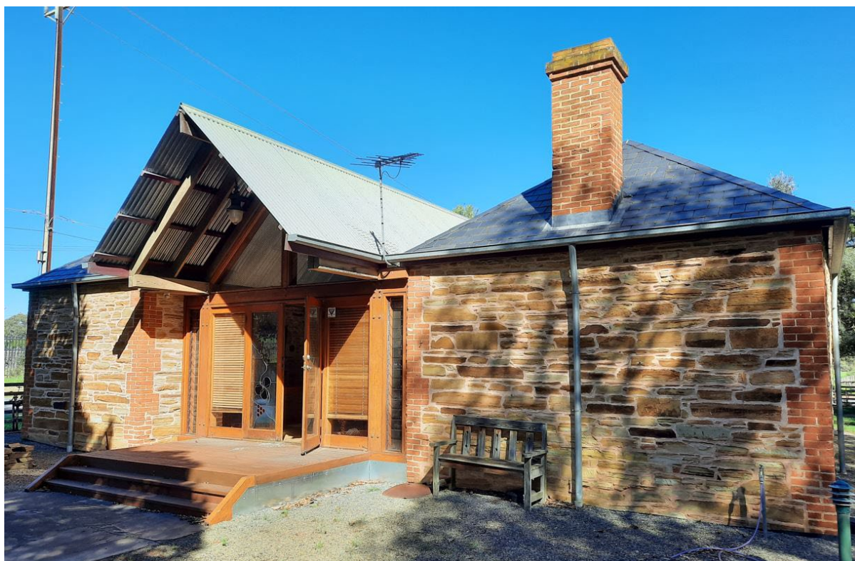
Former cottage ruin (now reconstructed) at 128 Main Road, Willunga (GGA, 2021)
