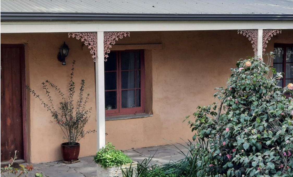
Rendered pug construction and early casement windows at 34 St Andrews Street, Willunga (GGA, 2021).
