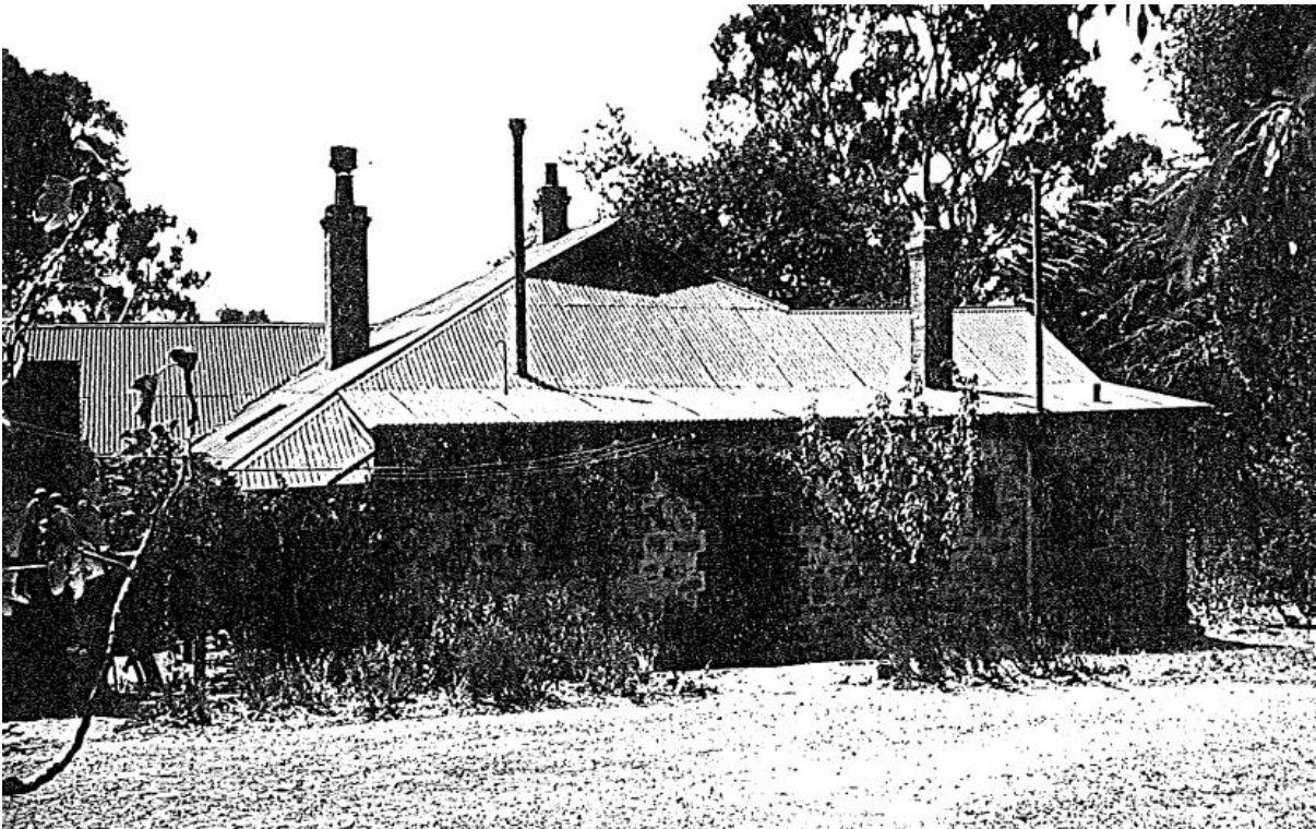
1983 photograph of 'Branden', 25 Shannon Crescent, Coromandel Valley (1983 Happy Valley Heritage Survey)
