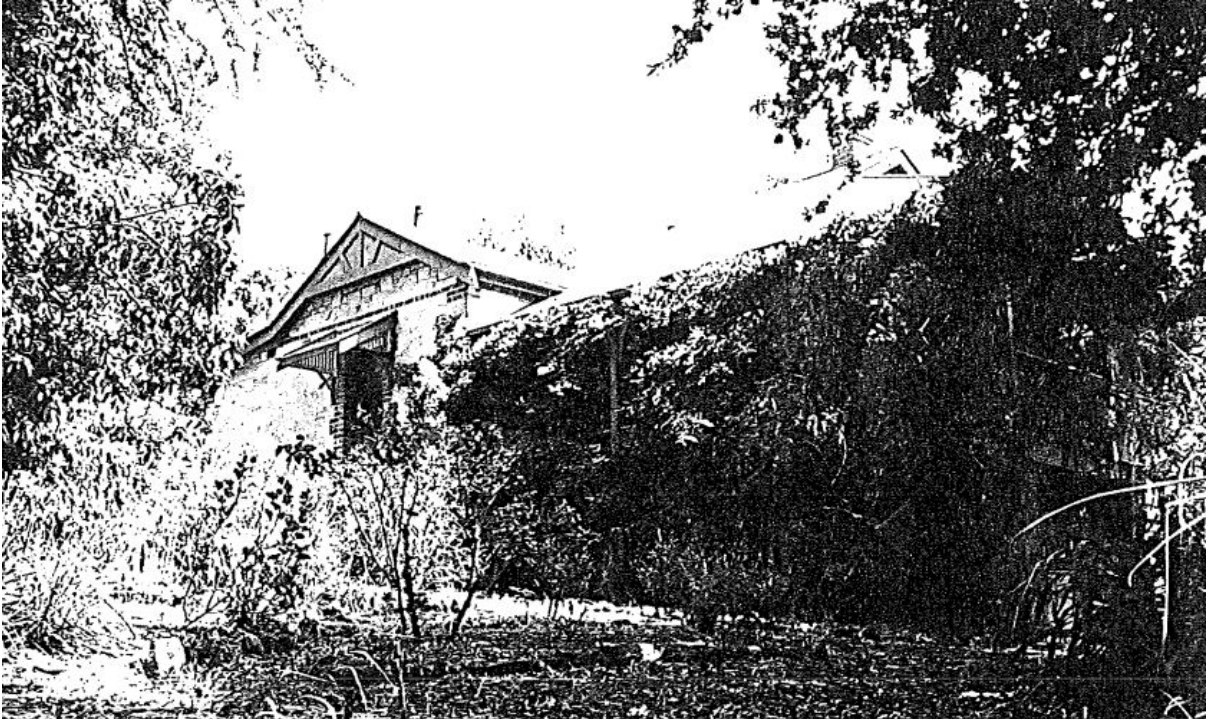
1983 photograph of 'Branden', 25 Shannon Crescent, Coromandel Valley (1983 Happy Valley Heritage Survey)
