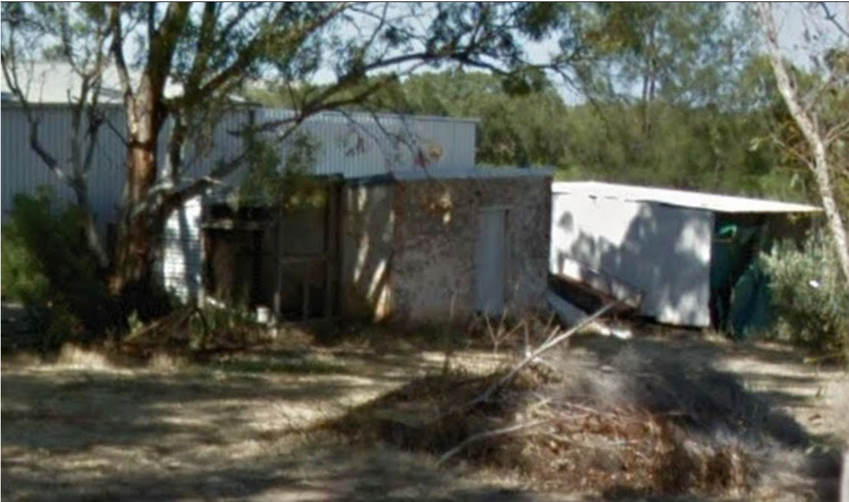
Early sandstone and brick lean-to outbuilding at 418 Plains Road, Sellicks Hill (Google Maps, 2014)
