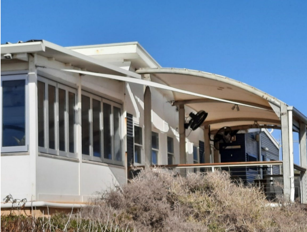
Extensive additions to original 'Star of Greece Café' building (GGA, 2021)
