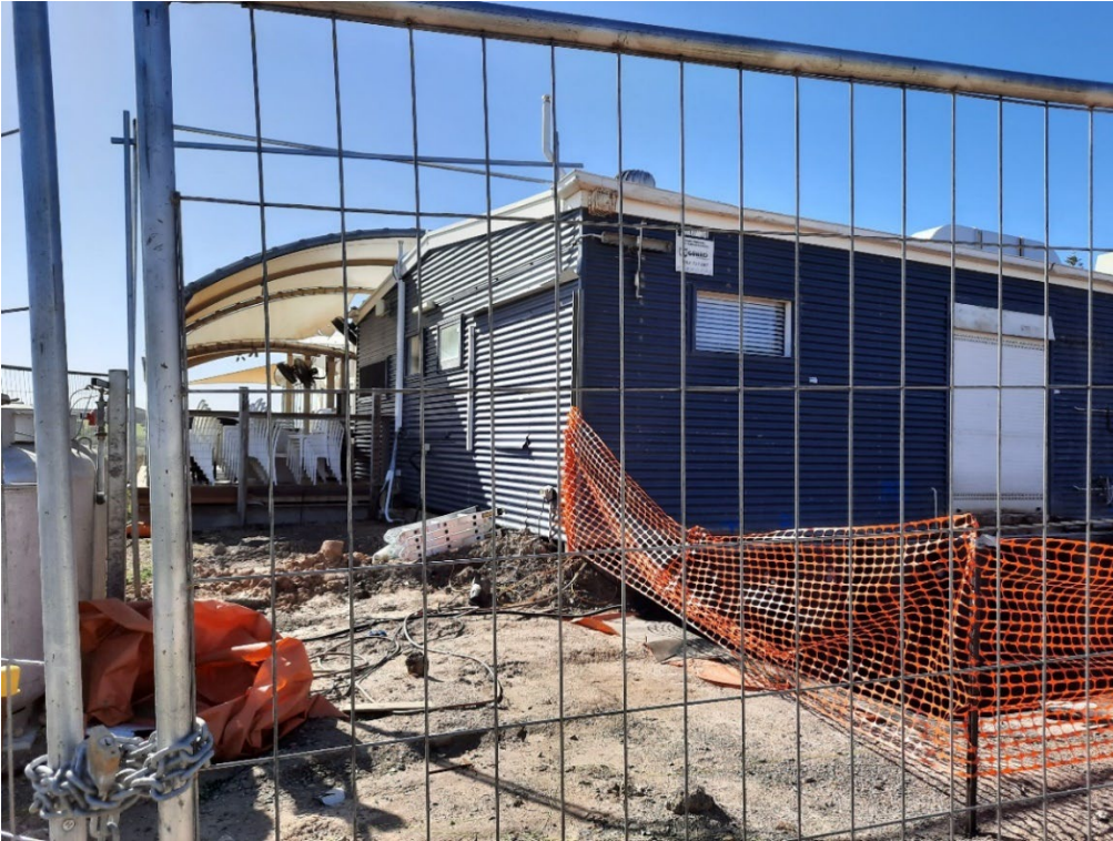
Extensive ongoing additions at 'Star of Greece Café' (GGA, 2021)
