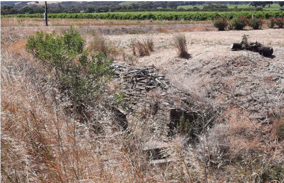
Drain & culvert, south-west corner of Malpas & Main Roads, Willunga (GGA, 2022)
