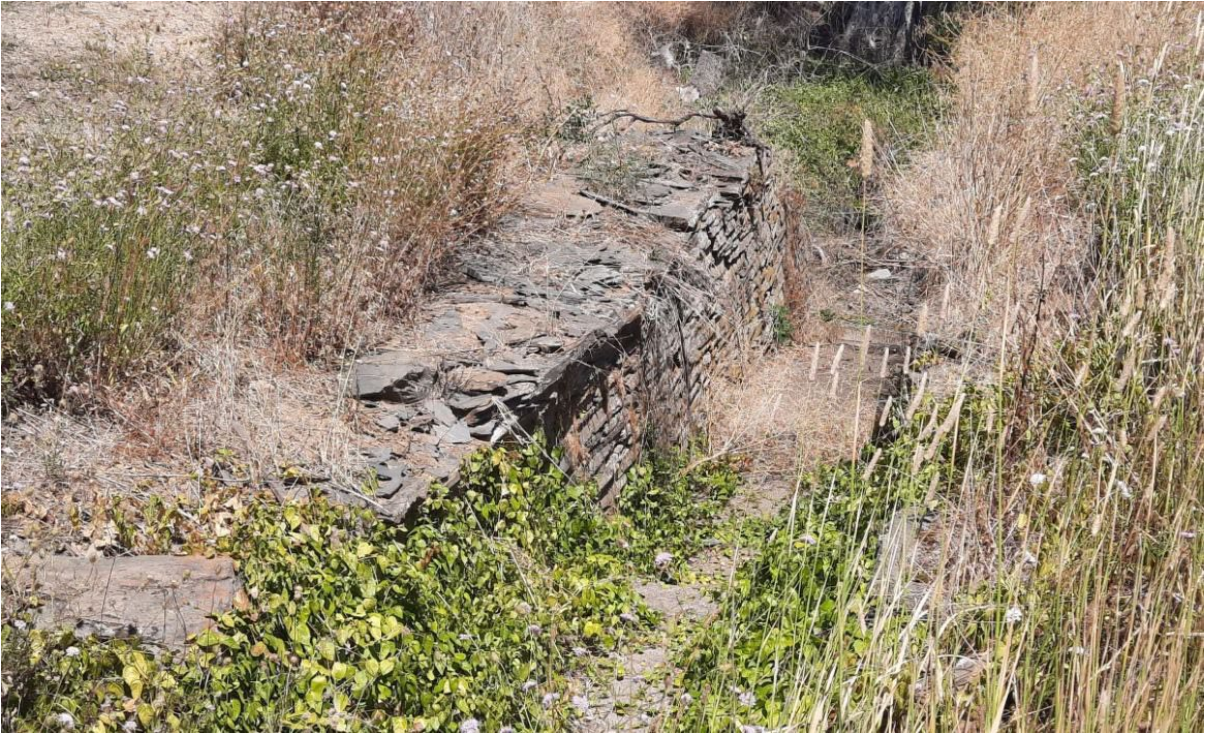
Drain and Culvert, south-west corner of Main and Malpas Roads, Willunga, reaching approximately 1.5 metres in height, looking south-west (GGA, 2022).
