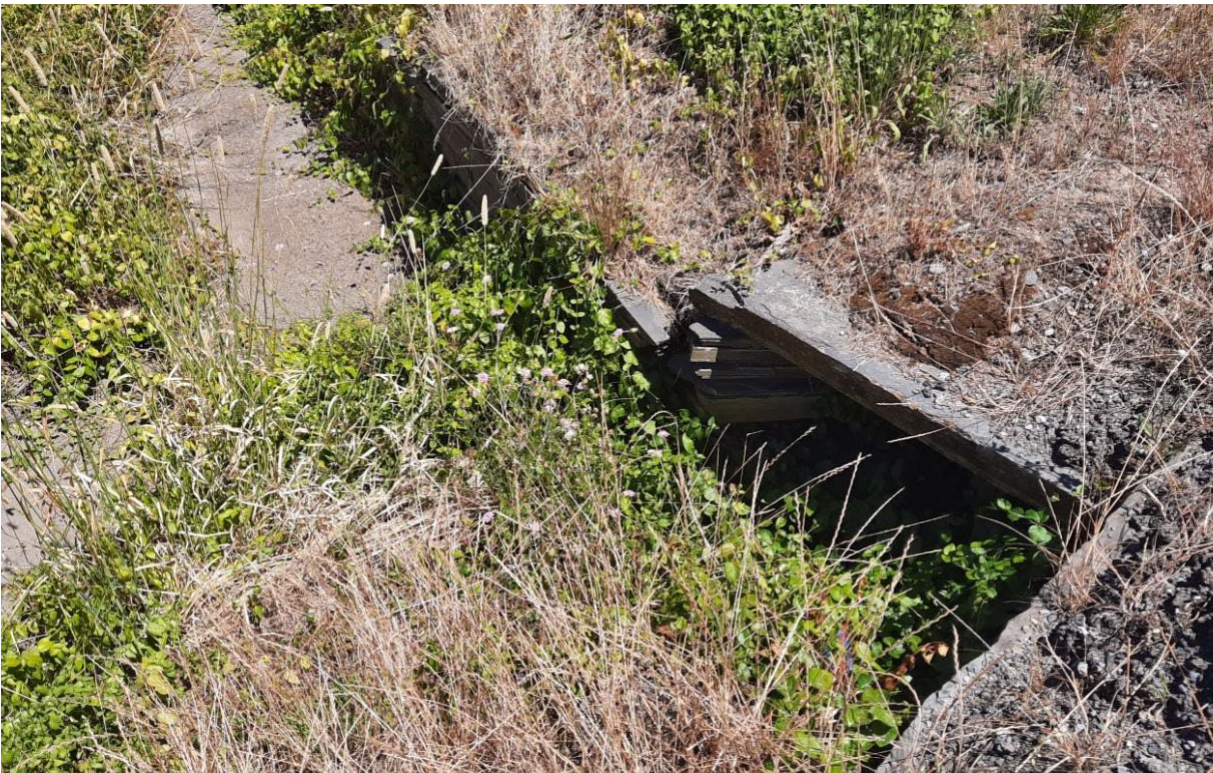
Drain and Culvert, south-west corner of Main and Malpas Roads, Willunga looking north-west, drain continues under Main Road to the east (GGA, 2022).
