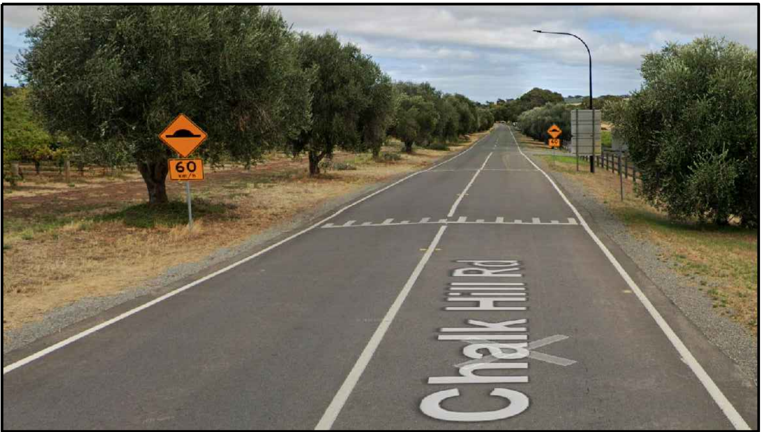
Example of asphalt rural raised safety platform.
