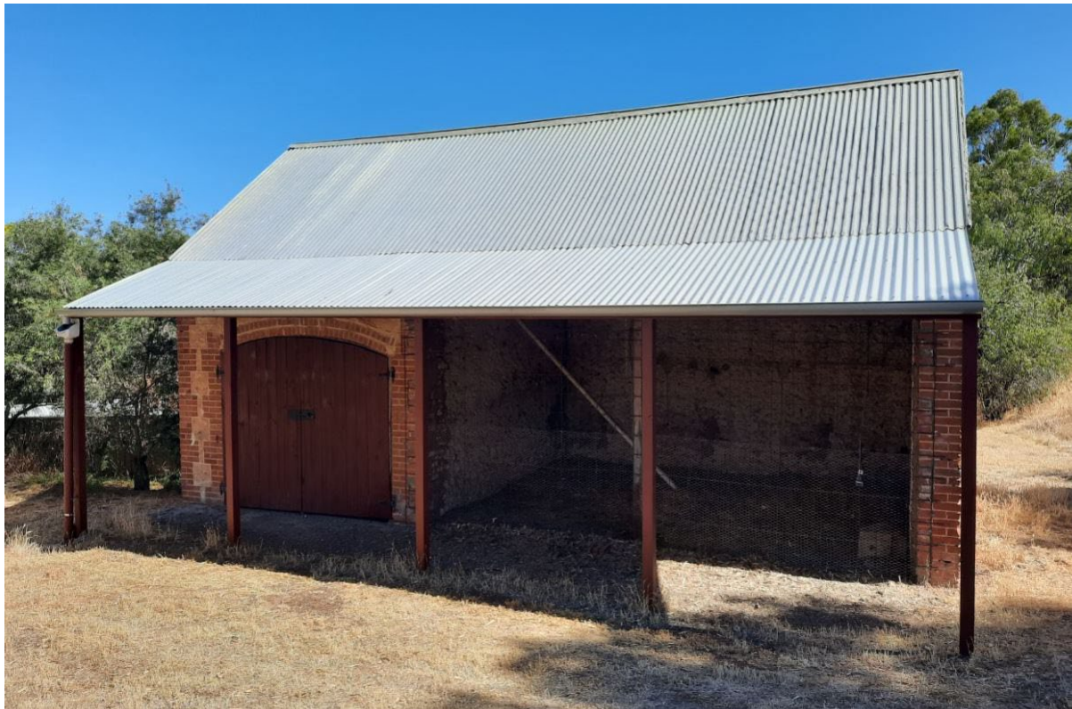
War Memorial Hospital (formerly 'Tsong Gyiaou') stables, 5-9 Aldersey Street, McLaren Vale (GGA, 2021)
