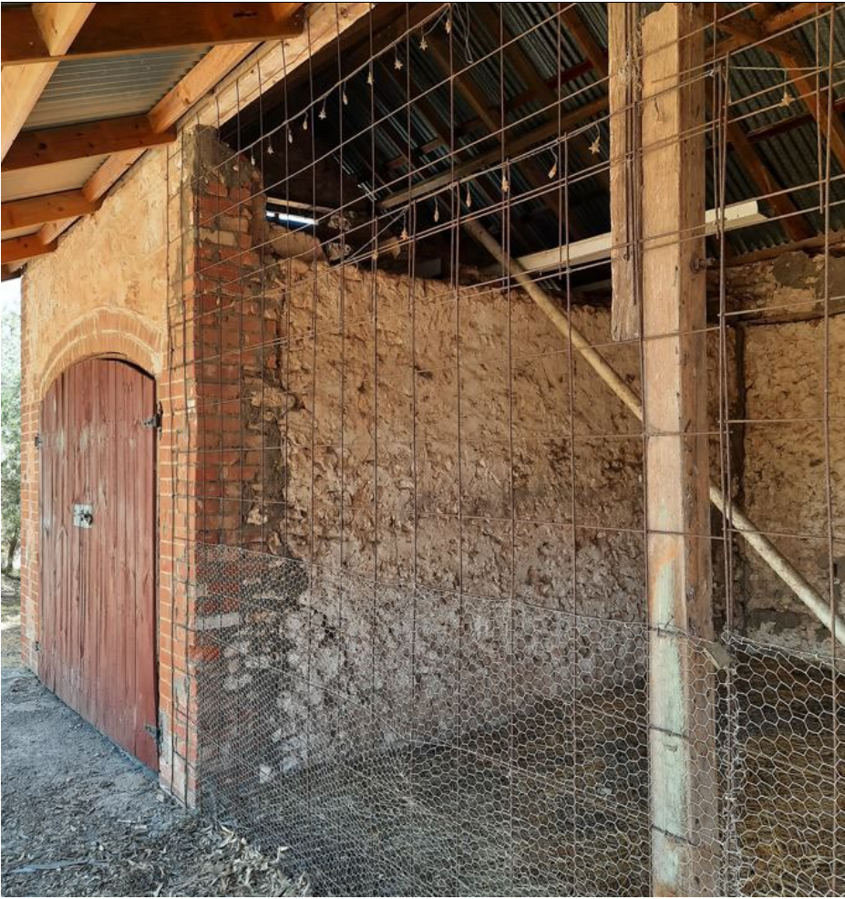
Internal elements of former 'Tsong Gyiaou' stables, looking north-west (GGA, 2021).
