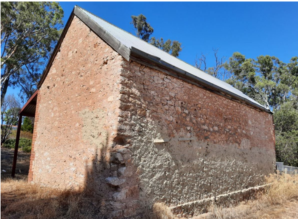
North and east elevations of former 'Tsong Gyiaou' stables, looking west (GGA, 2021).
