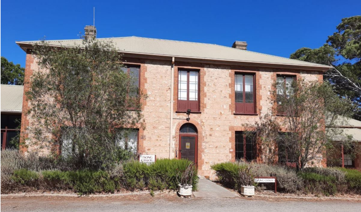
Former 'Tsong Gyiaou' homestead, looking west (GGA, 2021).
