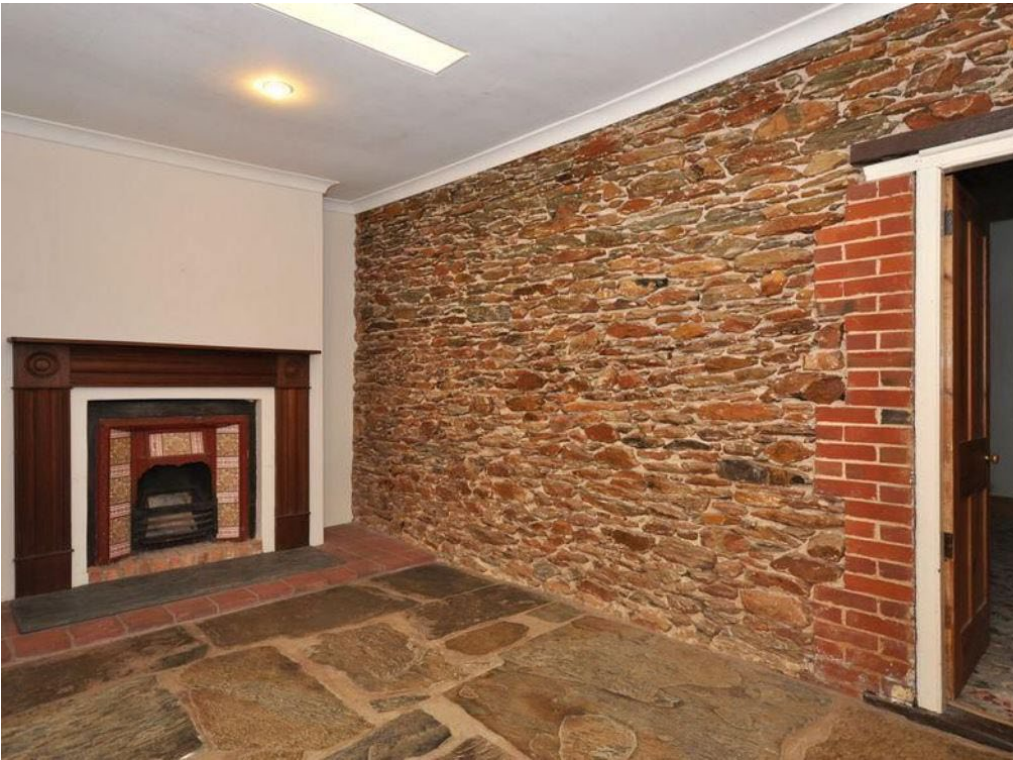
Former external walls to the dining room looking west, ( https://www.domain.com.au/property-profile/2-nicolle-drive-coromandel-valley-sa-5051 , accessed 20/1/2022).
