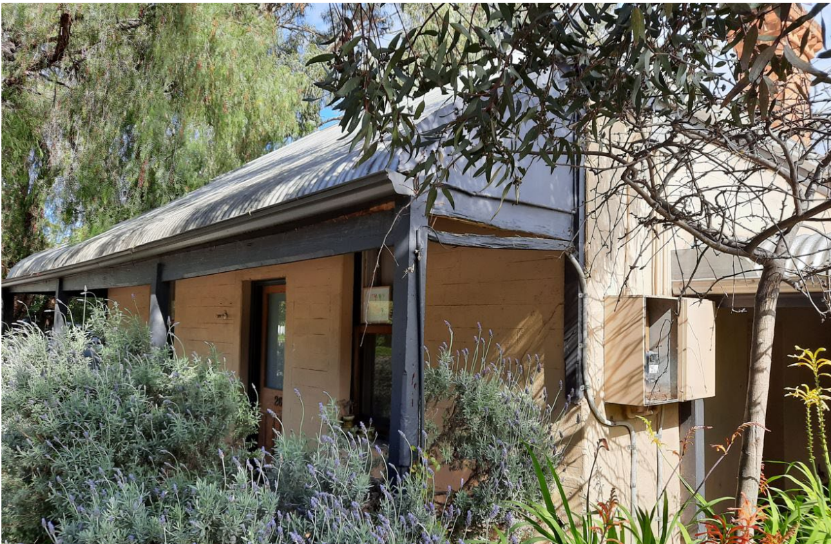
External pise walls to 26 St Andrews Terrace, Willunga now rendered and lined to resemble stonework (GGA, 2021)
