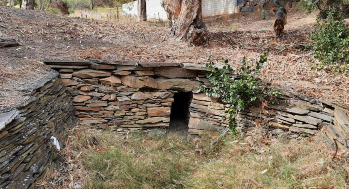
Primary mid-19 th century culvert wall and associated drain, with original subterranean slate slab flooring (GGA, 2022)
