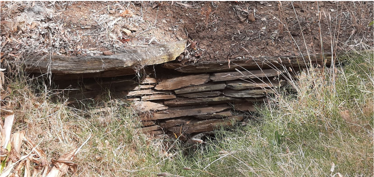
Slate wall construction with slate capping immediately beneath St Georges Street, looking west (GGA, 2022)
