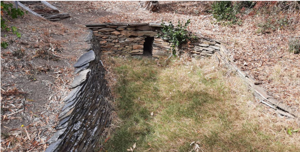
Substantial slate culvert located at Lot 2 (21-25) St Georges Street, Willunga (GGA, 2022)
