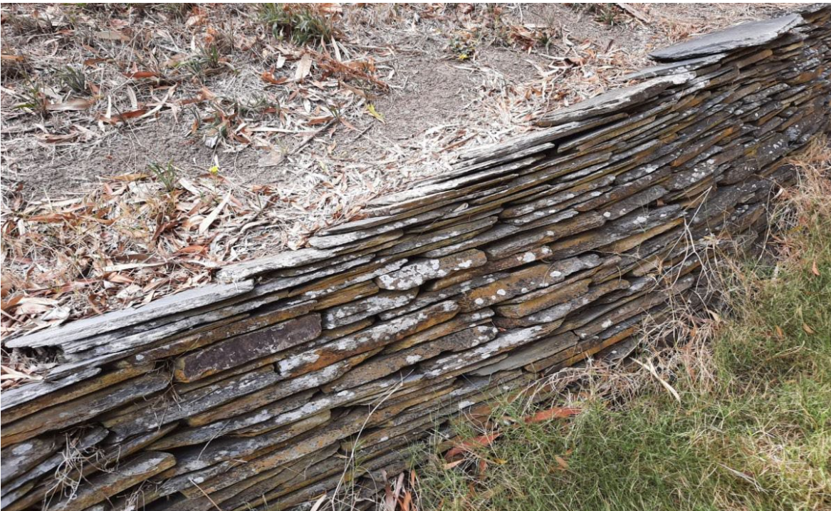
Mid-19 th century 'book leaf' slate construction to culvert, looking east (GGA, 2022).
