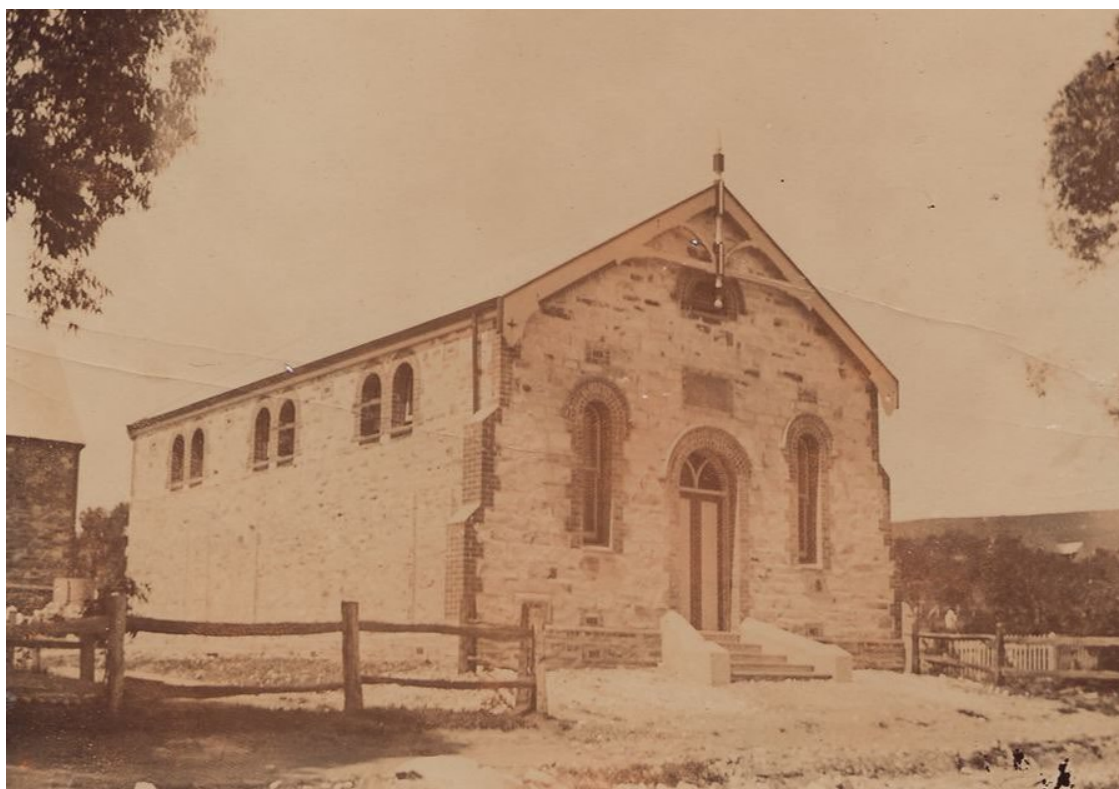
Early photograph of the Willunga Wesleyan Church schoolhouse, likely shortly after completion in c.1906. Note the elaborate timber gable has now been removed, the original stairs have been removed with the installation of a concrete ramp and timber-framed shelter to main entrance. ( https://www.flickr.com/photos/willunganowandthen/11960241934/ , accessed 16/9/2021).
