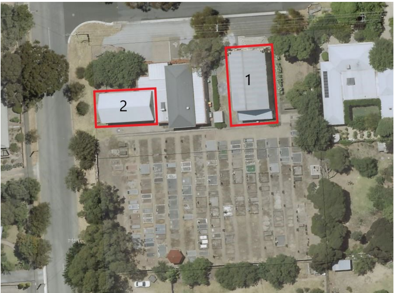
Site of 33 St Andrews Terrace, Willunga; (1) c.1895 church; (2) c.1906 classroom; cemetery located to the immediate south of church and classroom. (Planning SA SAPPa)
