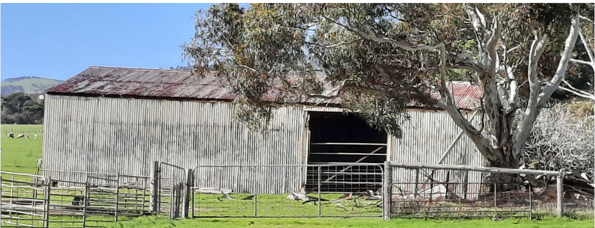
Former shed to immediate east of primary outbuilding (GGA, 2021)
