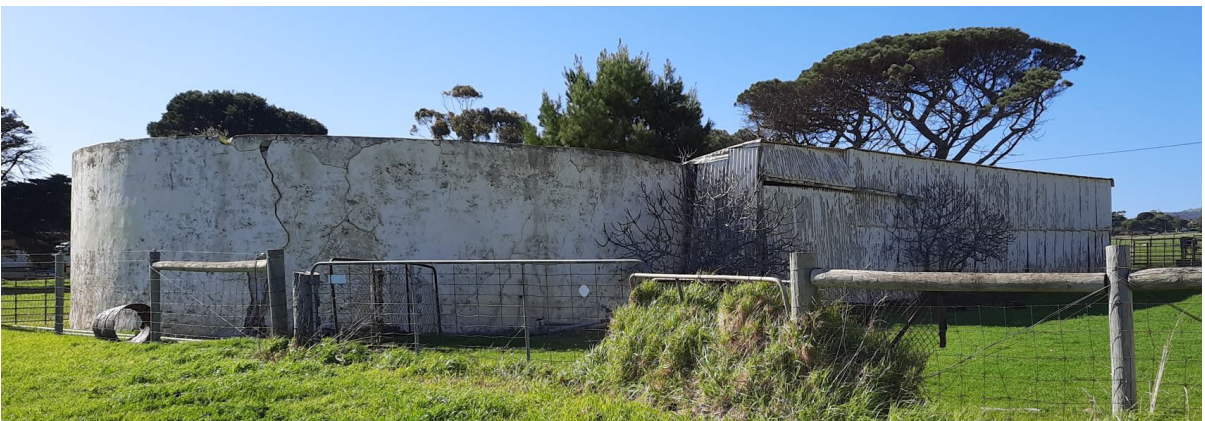
Mid-20 th century rendered concrete water tank and lean-to additions (GGA, 2021)
