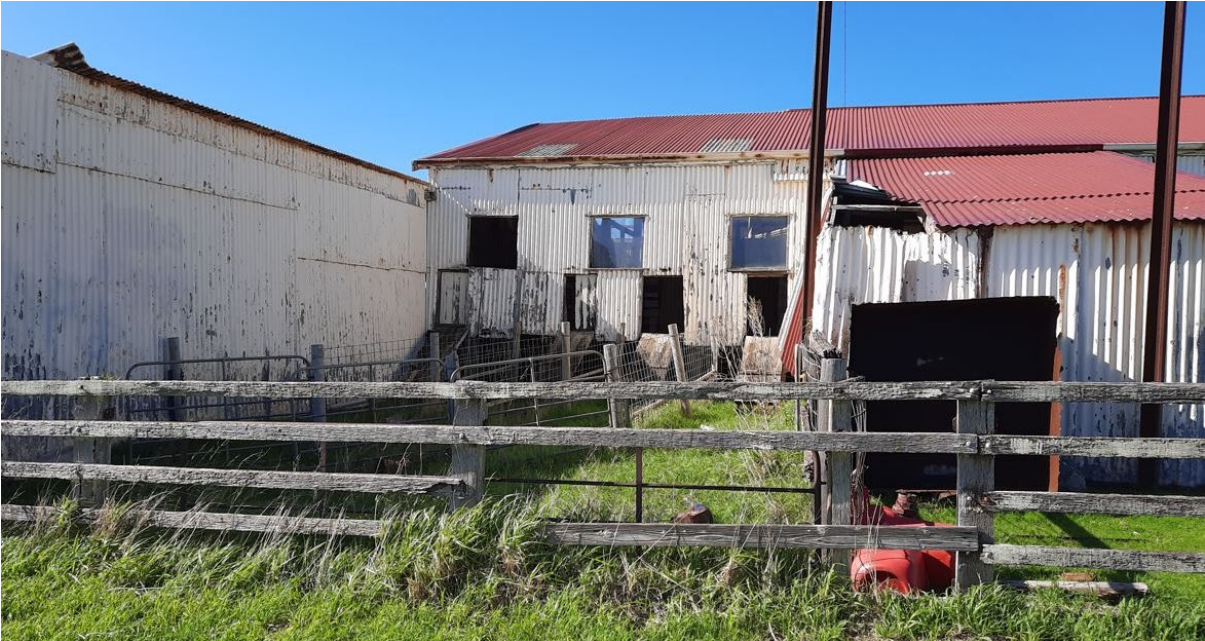
West elevation of primary outbuilding (likely former shearing shed) (GGA, 2021)
