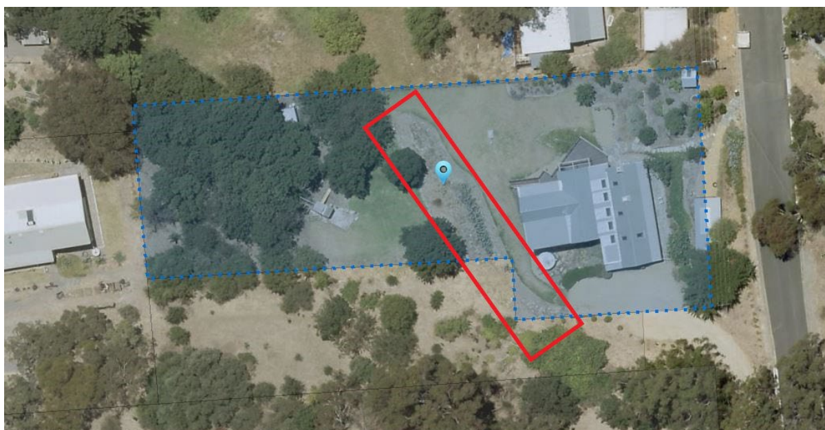
Site of 32 St Matthews Street, Willunga; slate culvert shown within red rectangle (Planning SA SAPPA)
