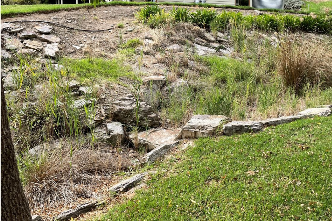
Early masonry fabric to slate culvert at 32 St Matthews Street, Willunga, looking east (GGA, 2022)
