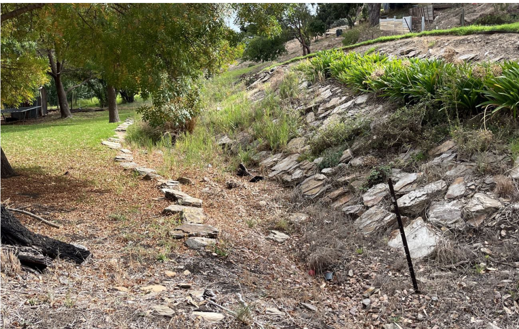
Early masonry fabric to slate culvert at 32 St Matthews Street, Willunga, looking north-west (GGA, 2022) (GGA, 2022)
