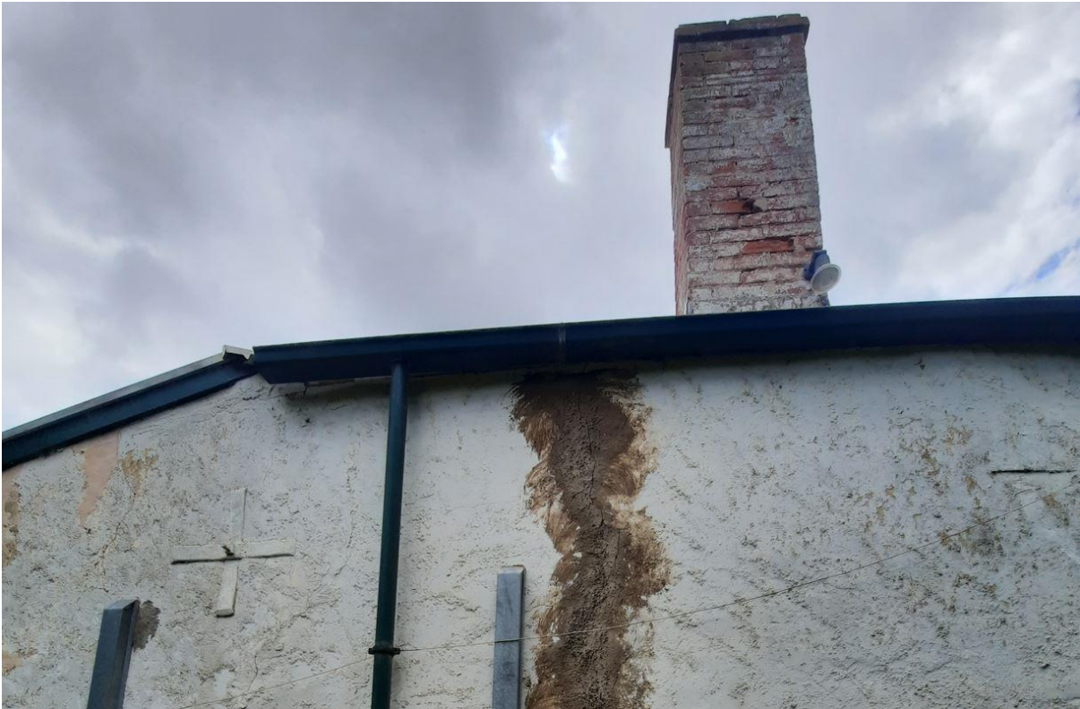
Upper portion of west elevation, with external rendering and early brick chimney (GGA, 2021).
