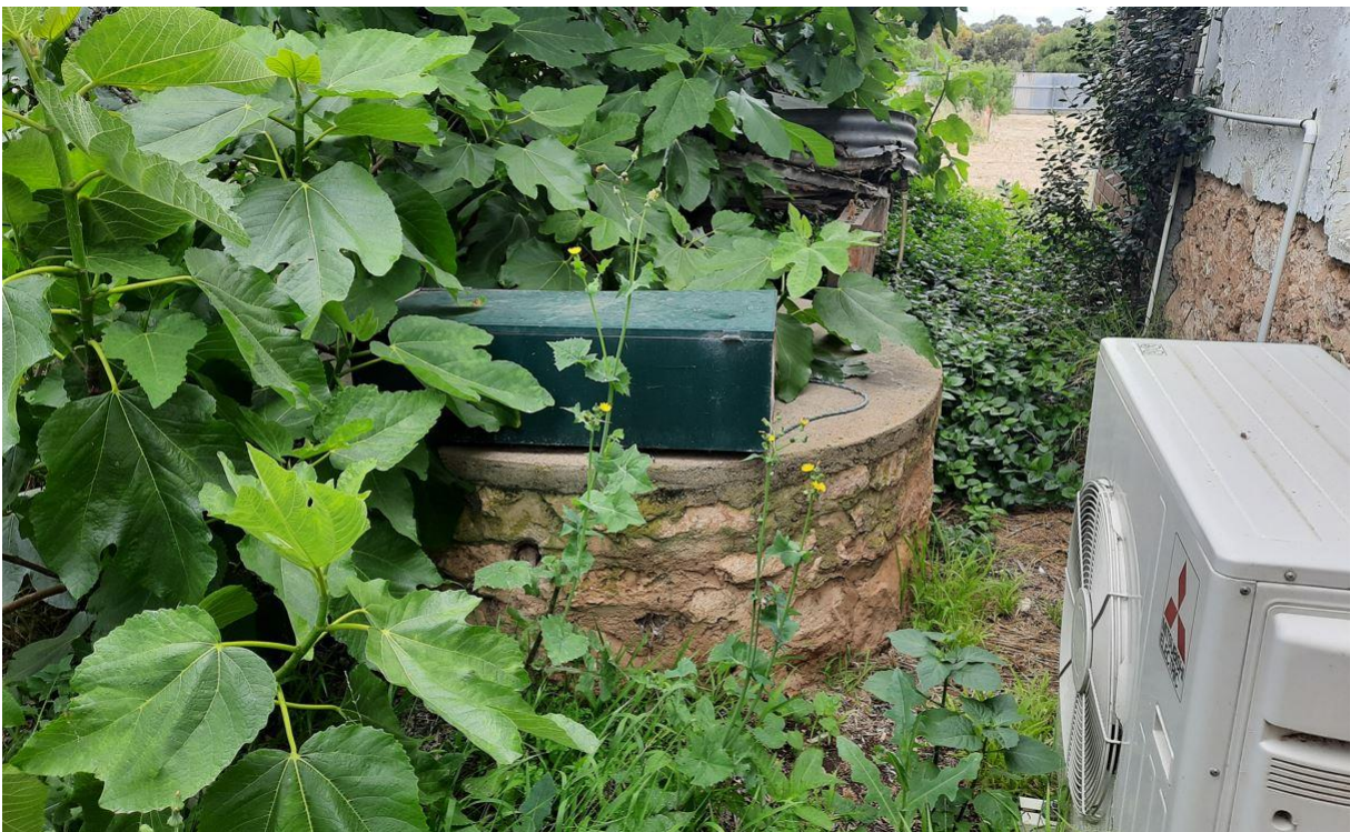
Masonry well with later concrete capping to immediate west of former cottage (GGA, 2021).
