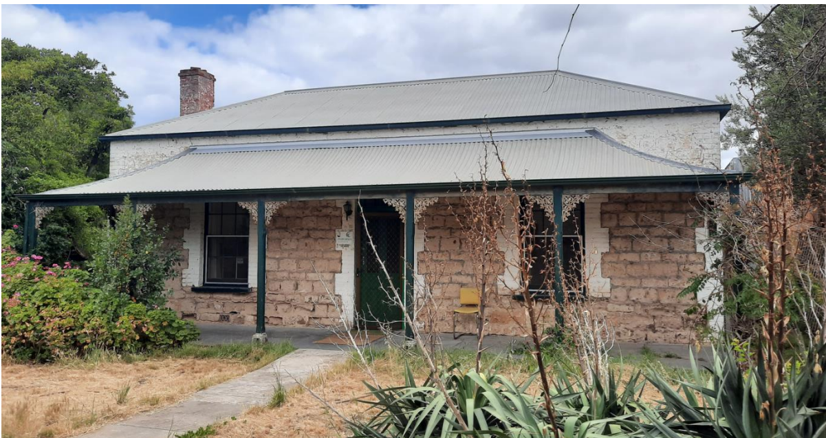
Cottage at 191 Port Road, Aldinga (GGA, 2021)
