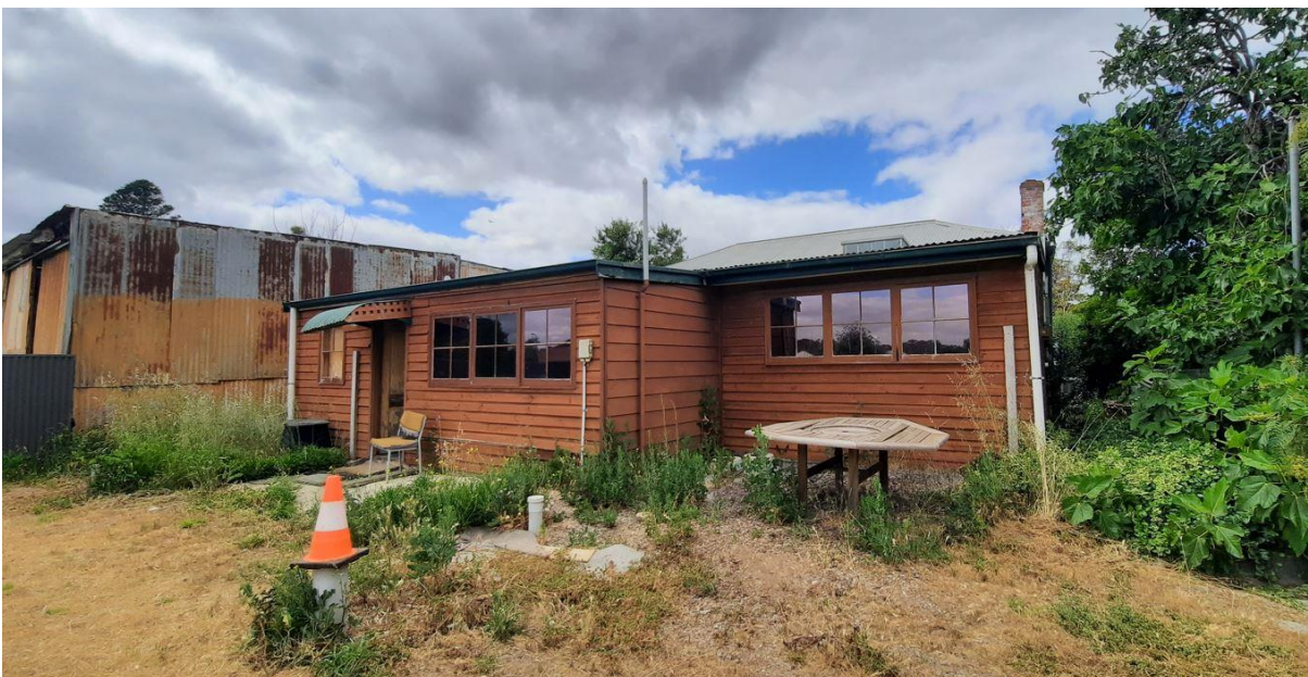
Timber framed and timber clad late 20 th century additions, abutting early lean-to additions to immediate north, viewed looking south. Adjoining sheds appear to date from the mid 20 th century. (GGA, 2021).
