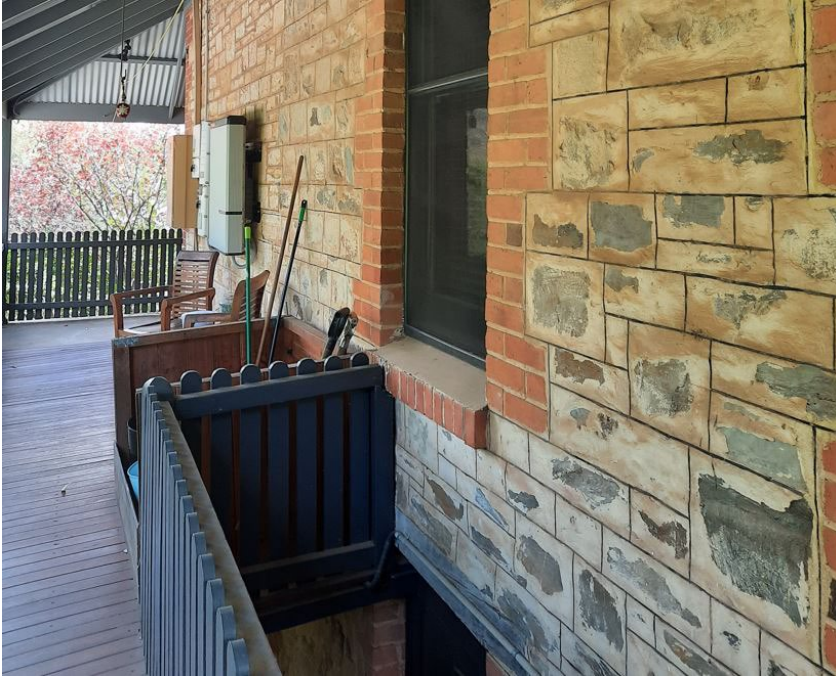
Bluestone fabric associated with the c.1887 cottage with later sandstone fabric to the immediate west, completed by the mid-1910s. Cellar rooms appear to have been completed as part of the c.1887 building (GGA, 2022)
