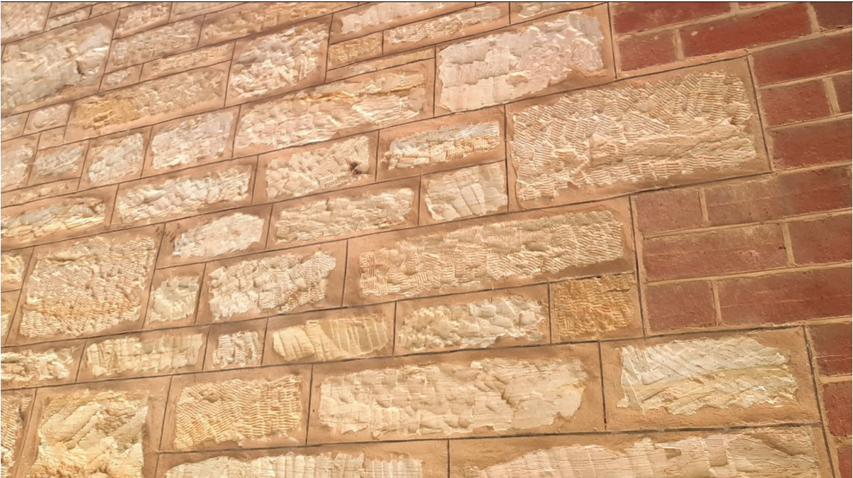
'Chisel-pecking' effect to external sandstone blocks dating to early 20 th century additions to north elevation, a signature of John Weymouth junior's stonework (GGA, 2022).
