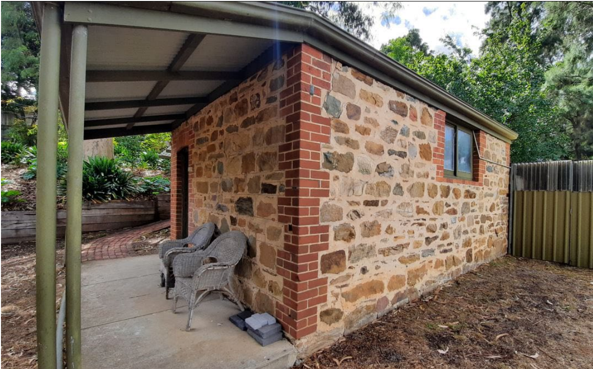
South elevation of the c.1915 bakehouse, showing original fabric to west and south elevations (GGA, 2022).
