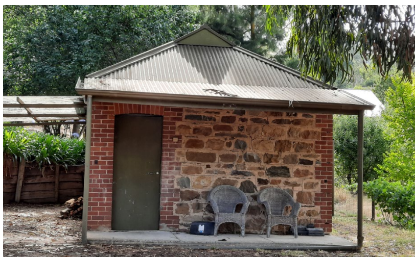
Residence (above) and former bakehouse (below) at 19 Rowlands Hill Road, Coromandel Valley (GGA, 2022)
