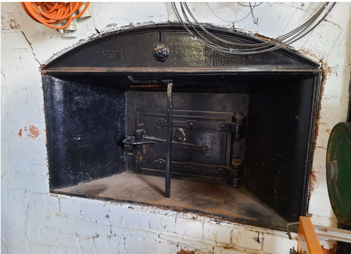
Intact c.1915 cast iron oven elements to internal north wall of former bakehouse (GGA, 2022).
