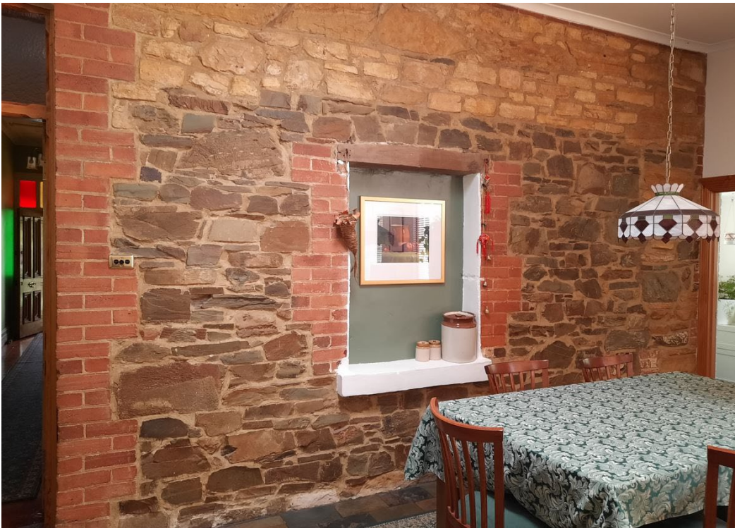
Former external wall comprising c.1887 east elevation, demonstrating various periods of stonework; ie. 1887 bluestone work, later early 20 th century stonework executed in sandstone (GGA, 2022)
