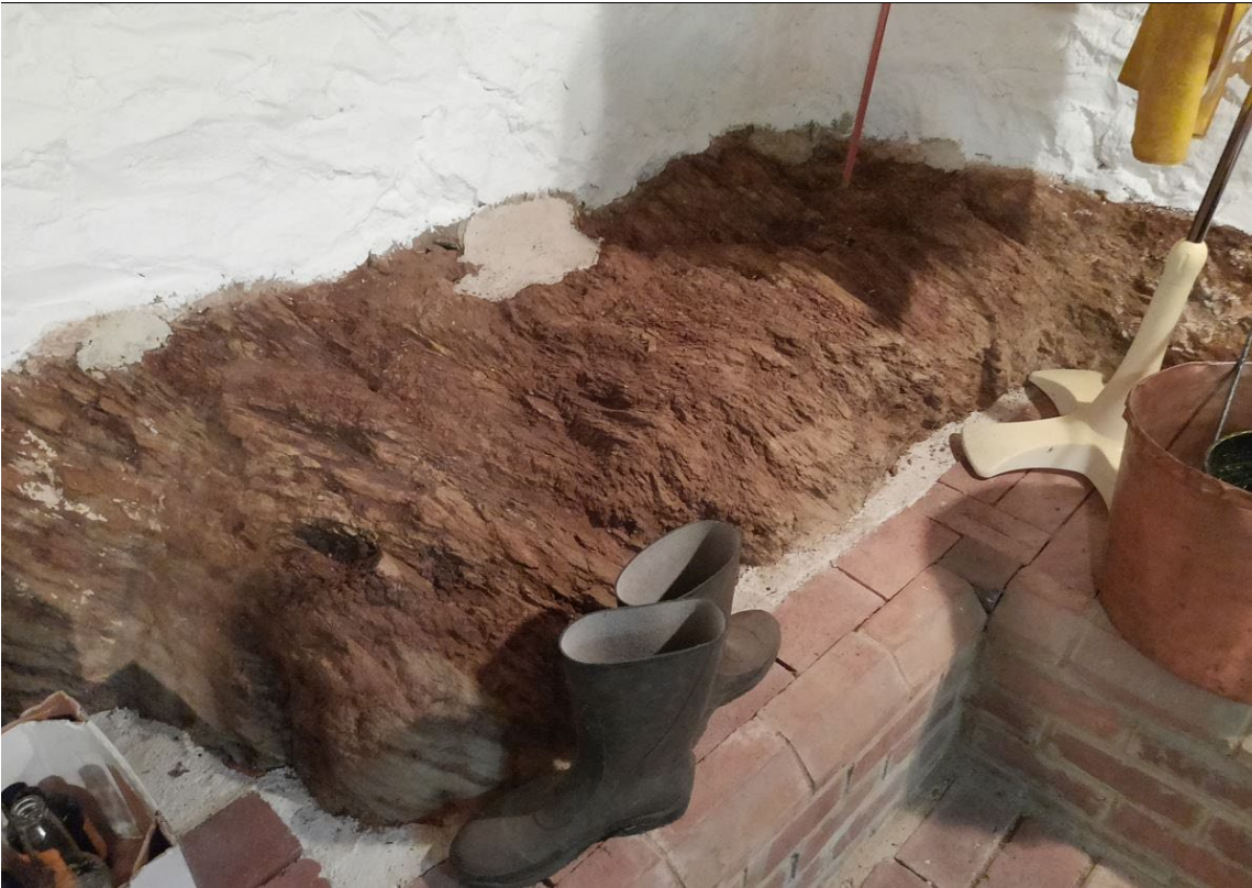
Raw stone foundations to interior of cellar rooms to base of c.1887 building (GGA, 2022).
