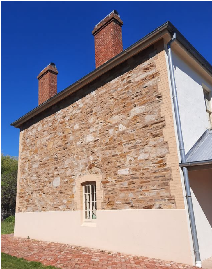
North elevation of 'Ingleburne' – early mid-19 th century photography shows the window was added at a later date (GGA, 2021).
