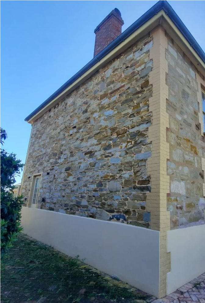
South elevation of 'Ingleburne' (GGA, 2021).
