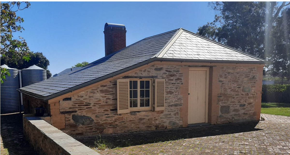
East elevation of 'Ingleburne' former dairy (GGA, 2021).
