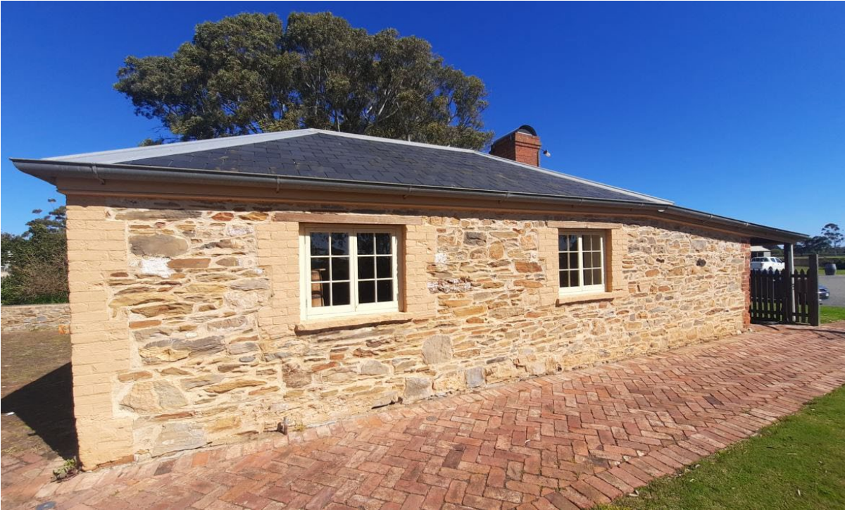
North elevation of 'Ingleburne' former dairy (GGA, 2021).
