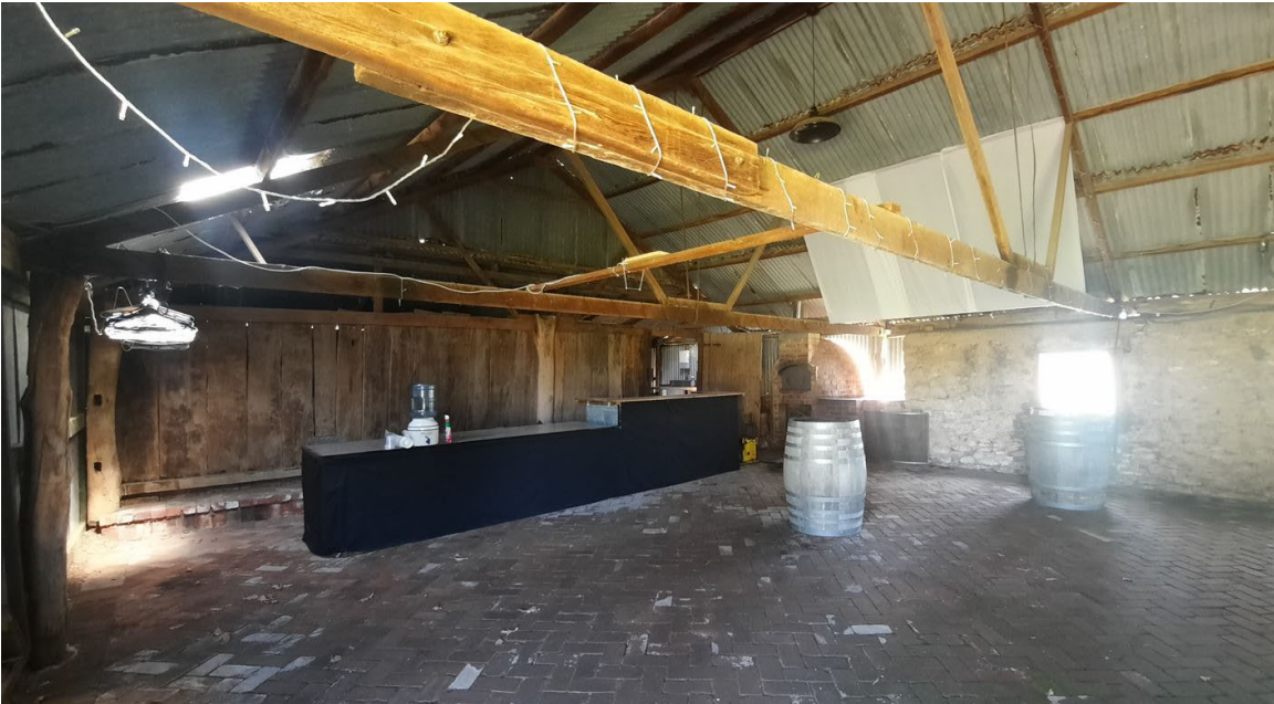
Early timber fittings to early outbuilding (GGA, 2021).
