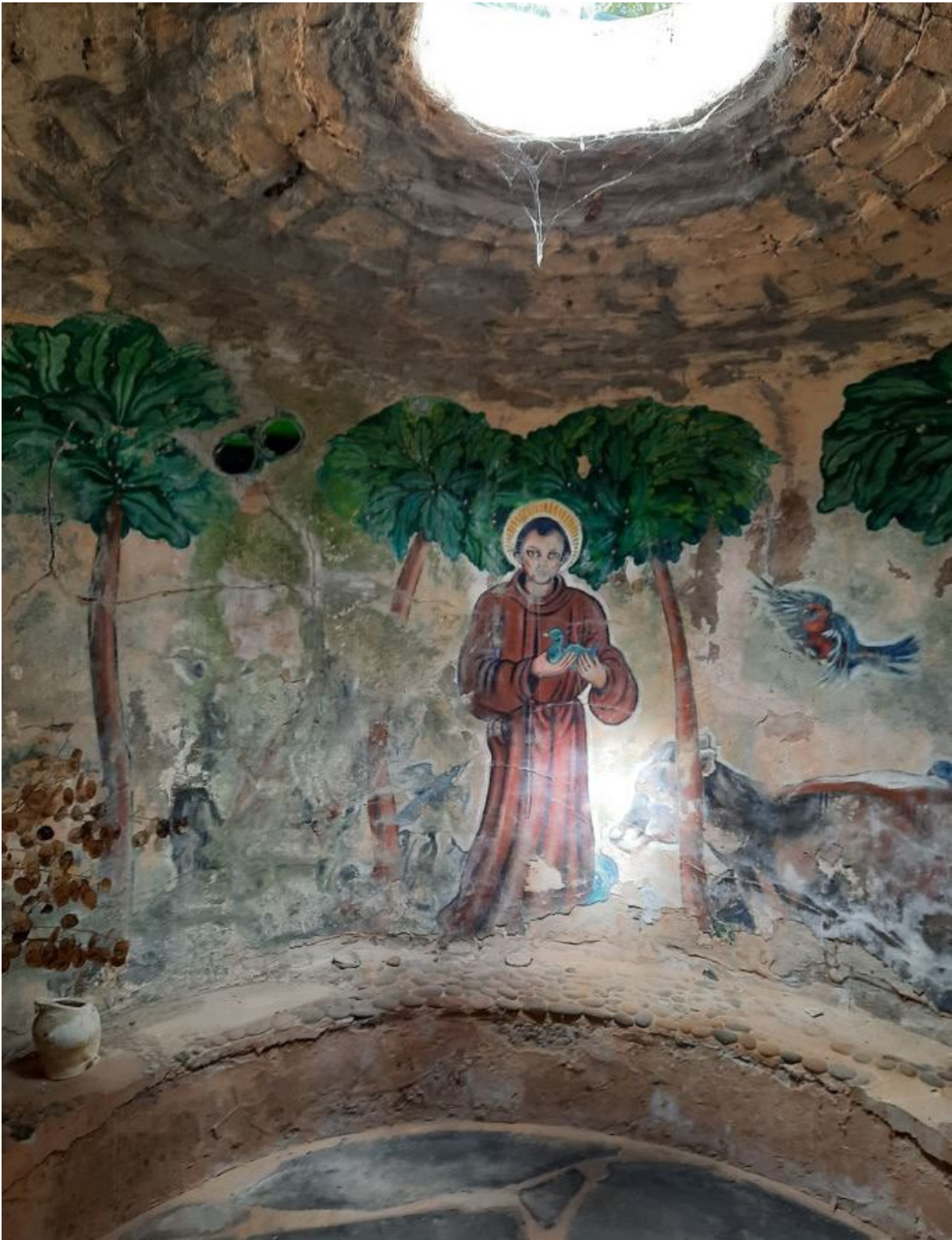
Late 20 th century wall mural to internal walls of former underground tank, appearing to depict St Francis of Assisi. Late 20 th century skylight over brick domed roof. (GGA, 2022).
