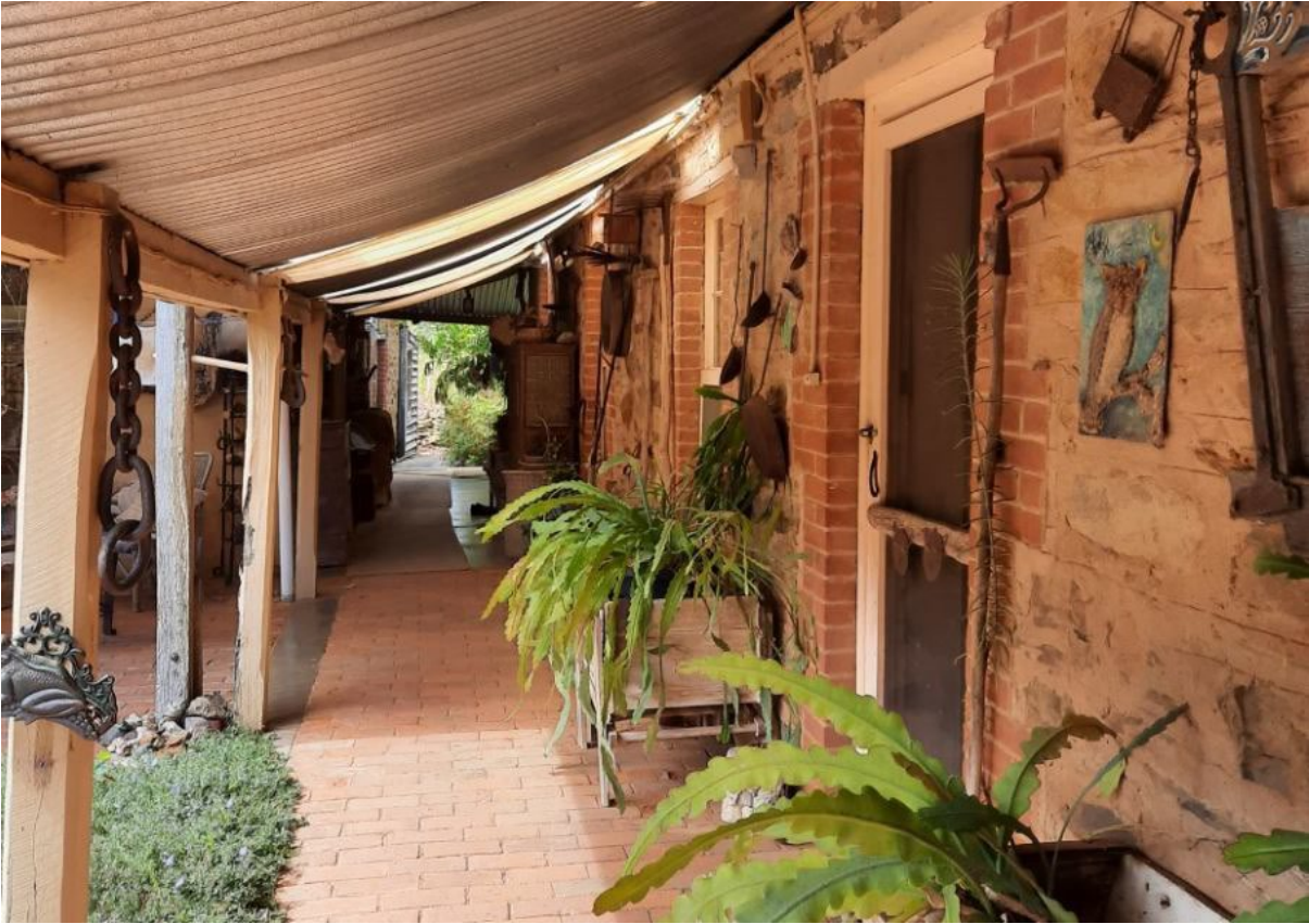
North elevation fabric of the mid-19 th century cottage, looking east (GGA, 2022)
