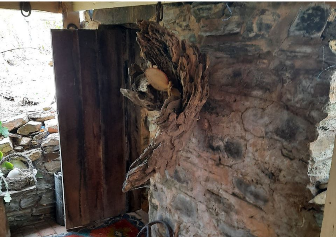
Entrance to former underground tank, timber door likely dating to the late 20 th century, looking east (GGA, 2022)
