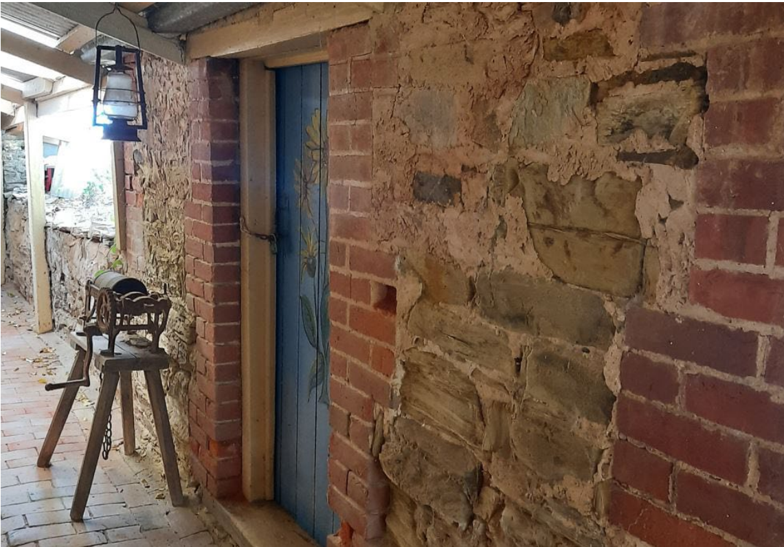
Original timber door and external masonry fabric of the mid-19 th century cool room and associated retaining wall, looking east (GGA, 2022)
