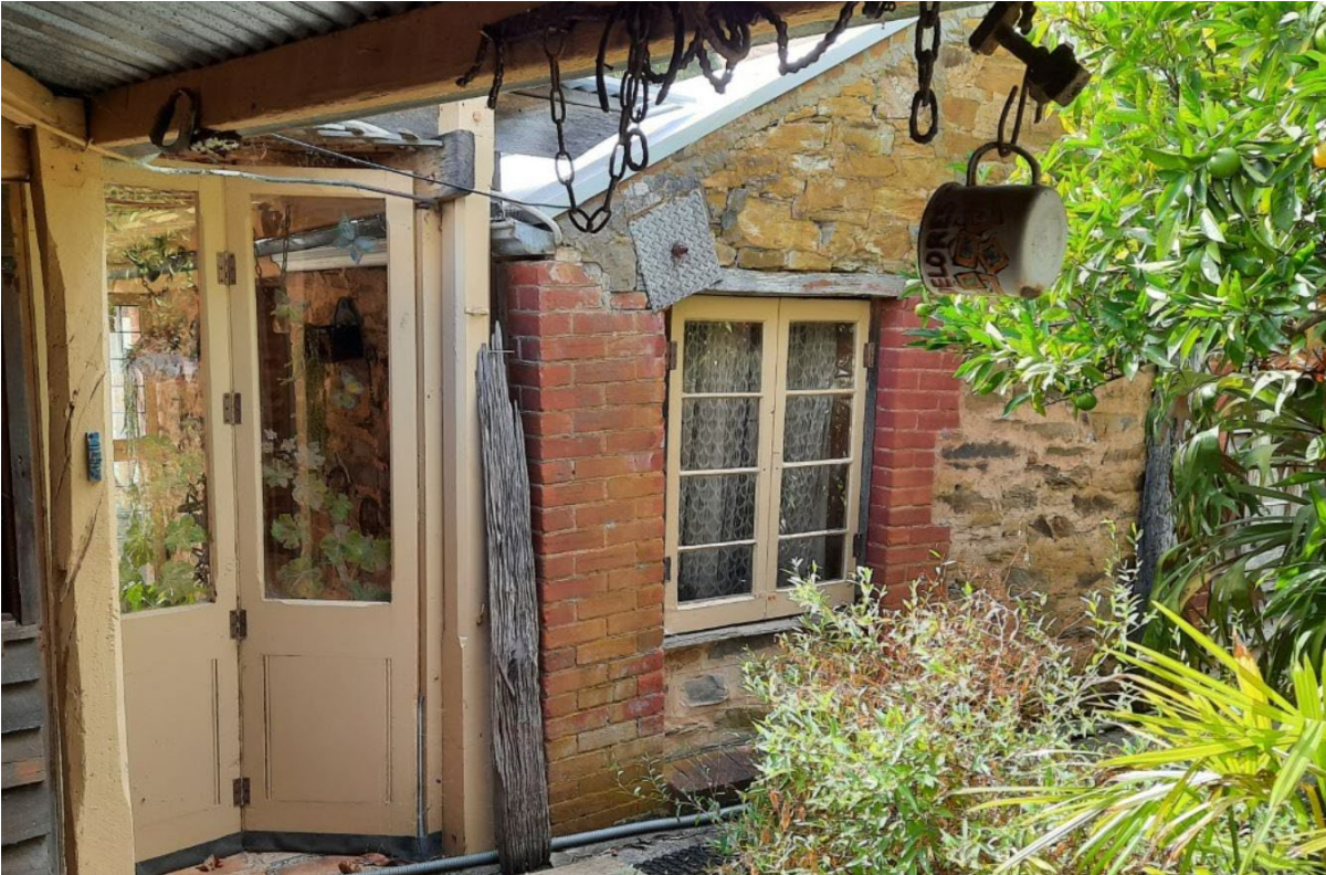
Former outbuilding to the immediate north-east of the cottage, showing original timber windows and masonry fabric with later additions and alterations for residential usage, looking north (GGA, 2022).
