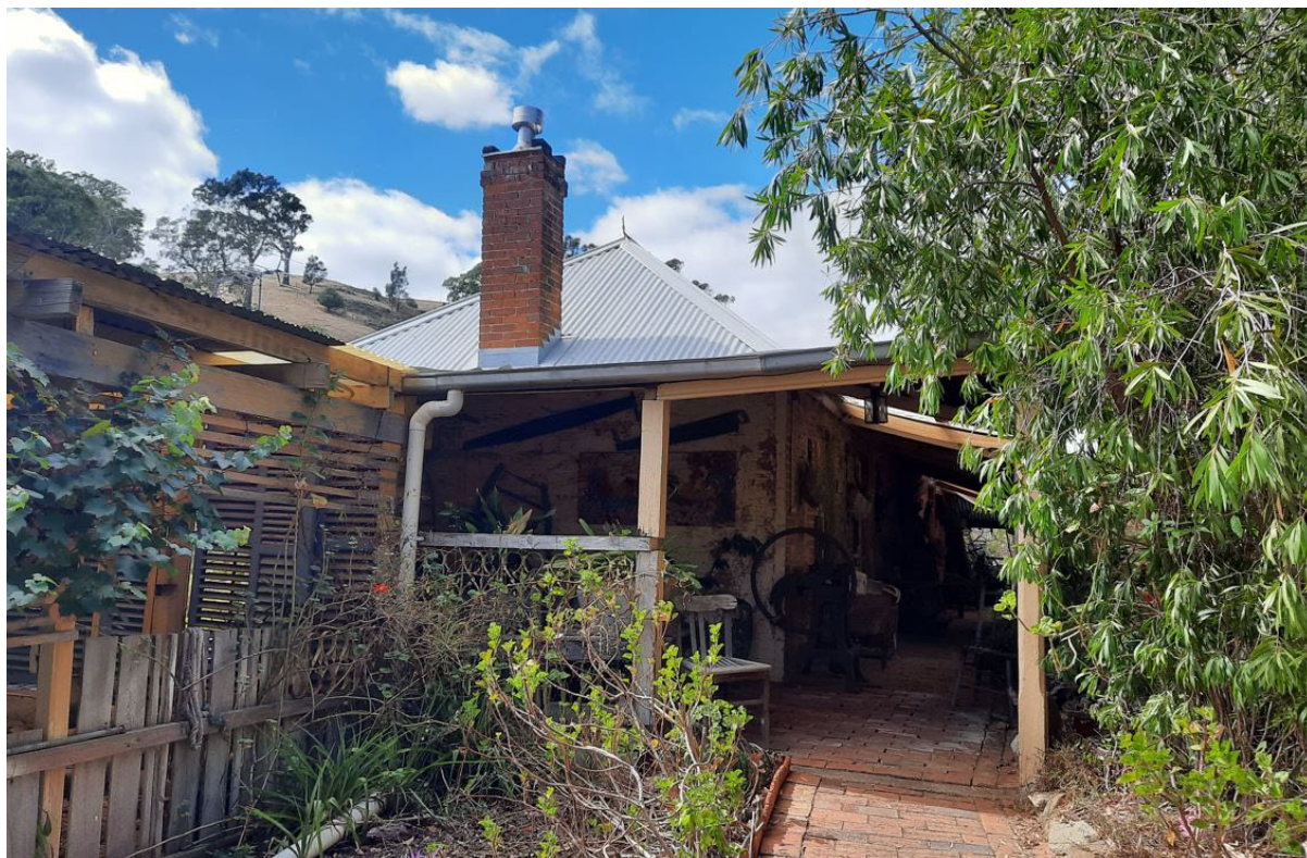
33 Cut Hill Road, Kangarilla (GGA, 2022)
