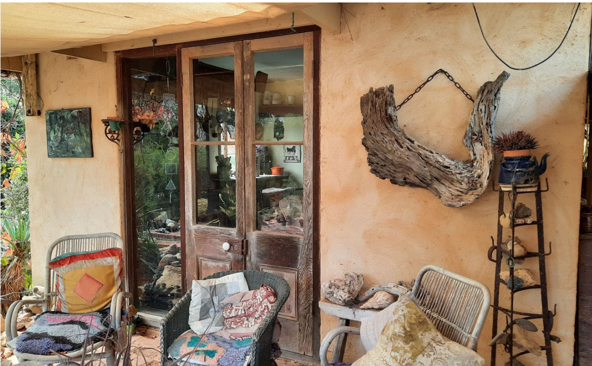
Later 20 th century pise outbuilding, likely used as studio, with timber doors and windows, immediately north of mid-19 th century cottage, looking east (GGA, 2022).
