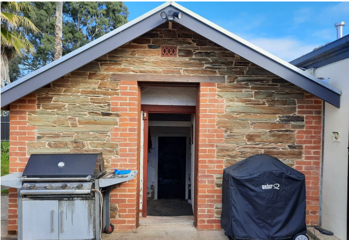
Early semi-excavated cellar with double walls and roofing dating to the mid-19 th century, recent replacement of external corrugated steel roof cladding (GGA, 2021).
