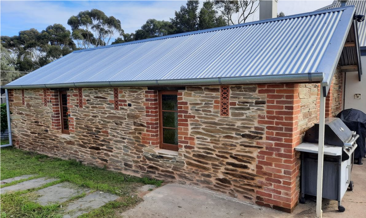
Early semi-excavated cellar with double walls and roofing dating to the mid-19 th century, recent replacement of external corrugated steel roof cladding (GGA, 2021).
