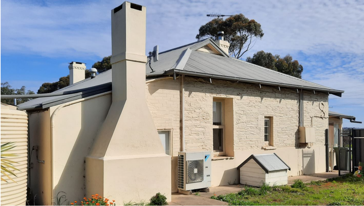
East elevation of former house; early kitchen chimney and an early small window have been retained despite extensive modifications and reconstruction works in c.1930s (GGA, 2021).
