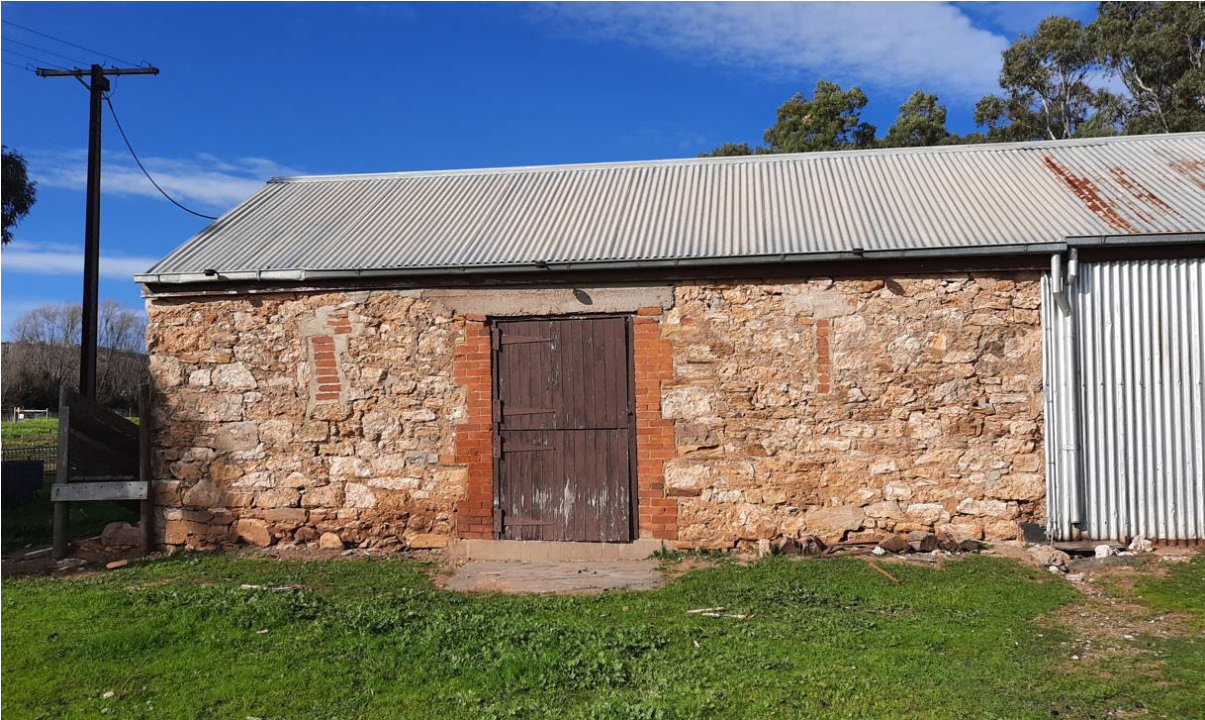
Mid-19 th century masonry and timber-framed farm outbuilding with various areas of early and later replacement corrugated steel cladding; lean-to additions to west elevation retain internal pug walls (GGA, 2021).
