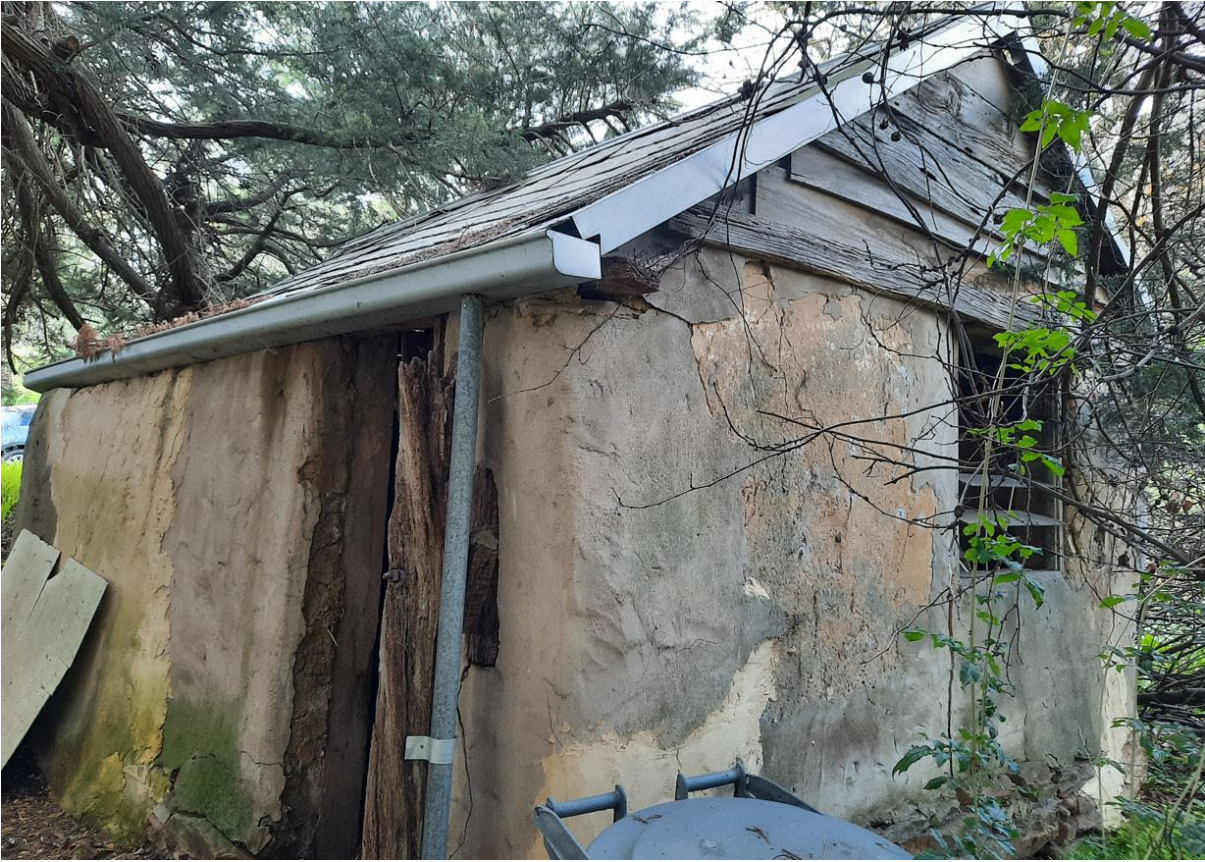
North and west elevations of early pise outbuilding, with external rendering, early timber fittings and various periods of slate roofing (GGA, 2021).
