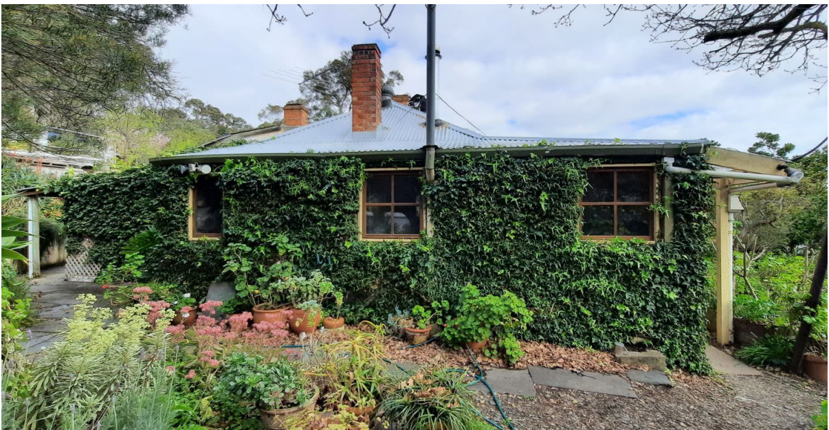
Early 20 th century additions to west elevation of c.1850s cottage (GGA, 2021).
