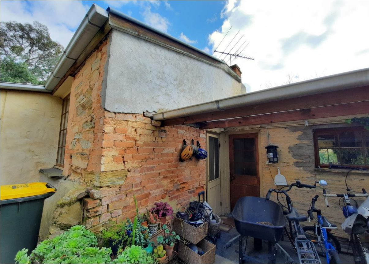
Early masonry to c.1850s lean-to additions and early 20 th century masonry fabric to south elevation (GGA, 2021).
