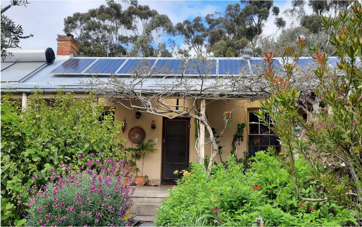
C.1850s original residence, now central portion of dwelling with modified roof and verandah (GGA, 2021).
