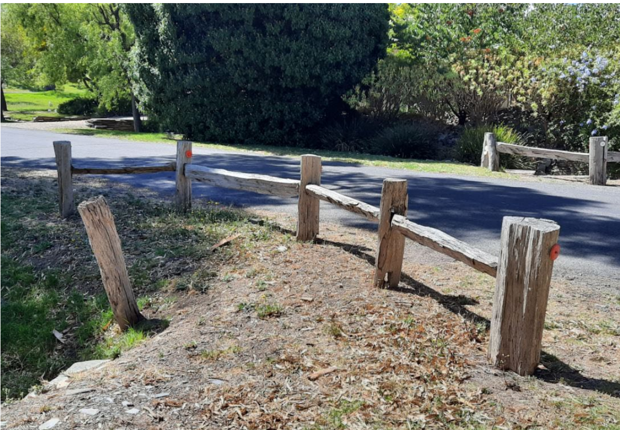
Northern end of culvert with early timber fencuing (GGA, 2022)
