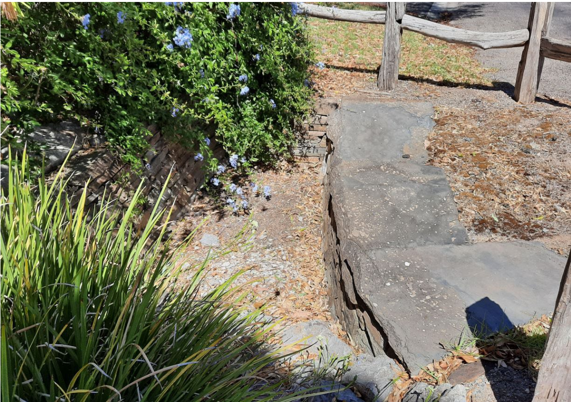
Masonry fabric to the southern end of the St Judes Street culvert (GGA, 2022)
