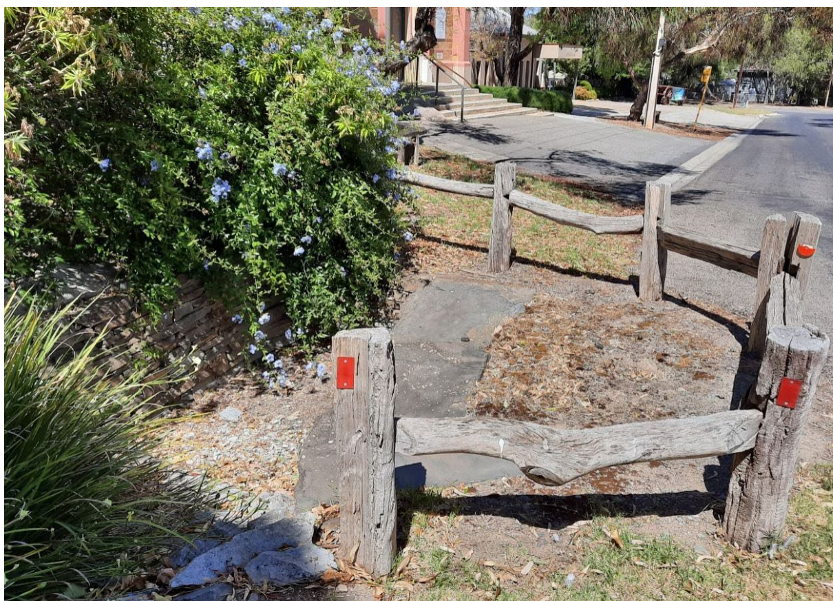
St Judes Street culvert, through which the 'unnamed Willunga creek' disposes into Lot 186 St Andrews Terrace, Willunga (GGA, 2022)
