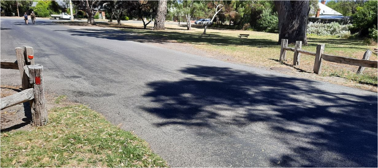
Culvert disposing across St Judes Street from 33 St Andrews Terrace to Lot 186 St Andrews Terrace. Early timber fence posts to both sides of culvert (GGA, 2022)
