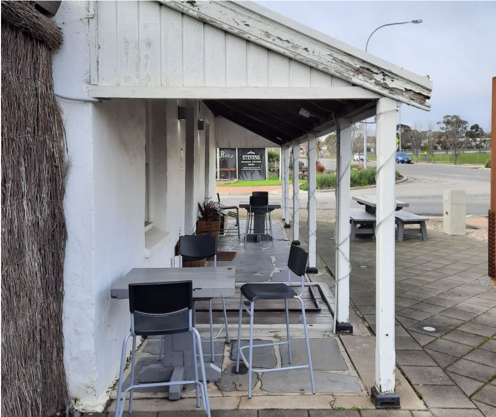
Slate paving and timber hatch entrance to cellar, facing Main Road looking south-east (GGA, 2021)
