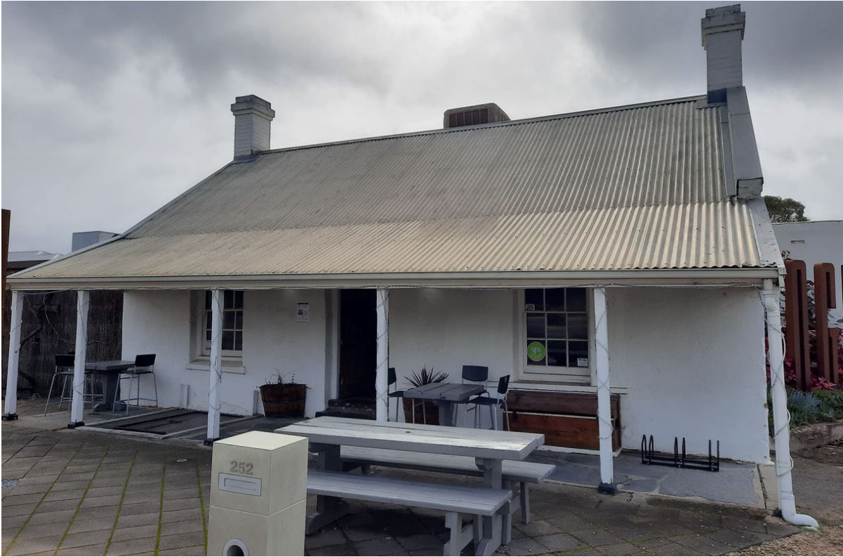
Former cottage at 252 Main Road, McLaren Vale (GGA, 2021)
