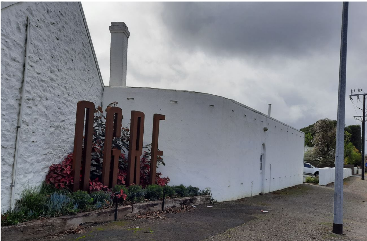
Later 20 th century additions with early masonry chimney, looking east (GGA, 2021)
