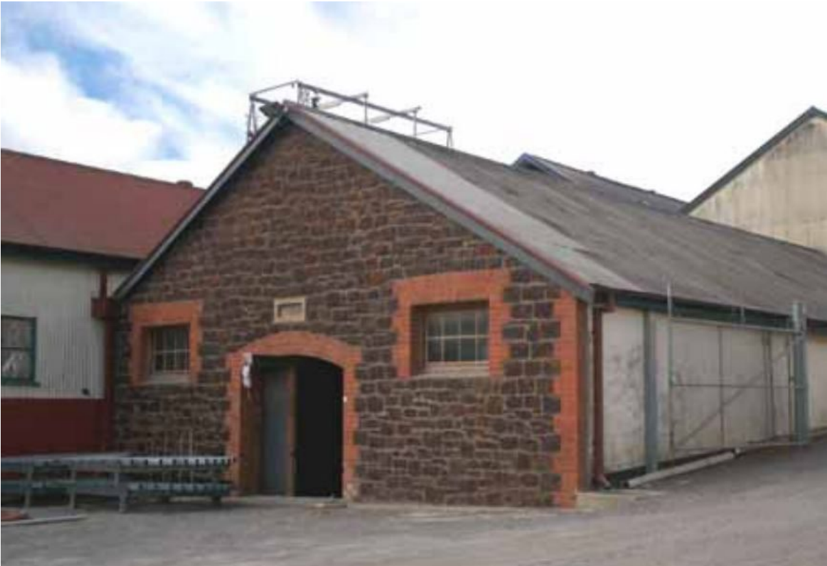
2007 photograph of c.1901 storage cellar at 20 Penfold Way, McLaren Vale (2007 McLaren Vale Township Local Heritage Register).
