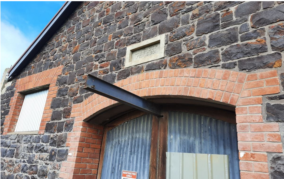
Former entrance to former cellar building, with original c.1901 stone plaque reading "Laid by C. E. P. (Cyril Eustace Pridmore), February 15 th , 1901." (GGA, 2021).
