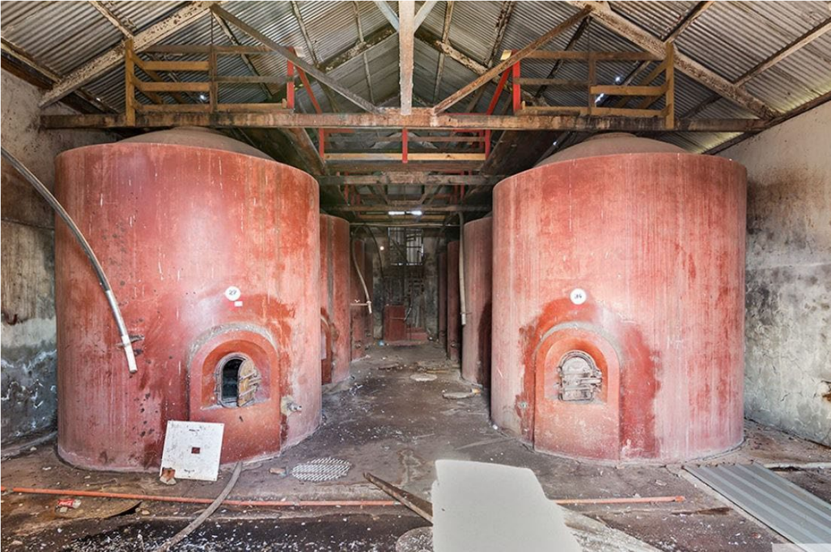
c.2015 photographs of early (c.1901) former vats and boilers to former cellar interior ( https://www.realestate.com.au/property/20-penfold-way-mclaren-vale-sa-5171 , accessed 21/10/2021).
