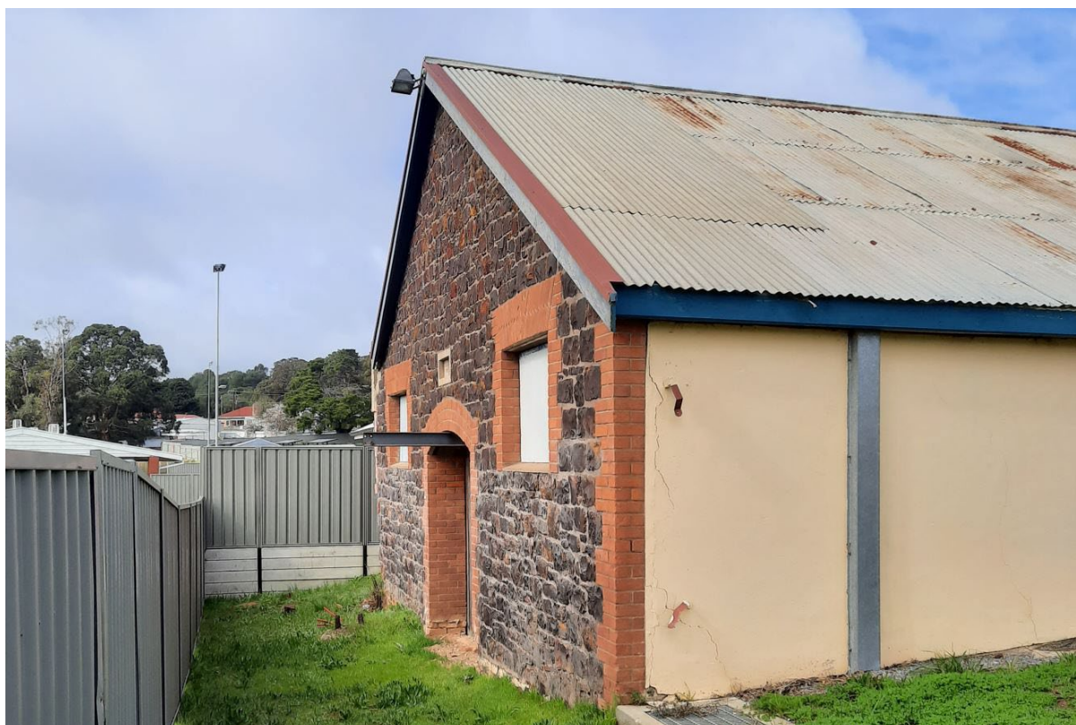
Former storage cellar, 20 Penfold Way, McLaren Vale (GGA, 2021)
