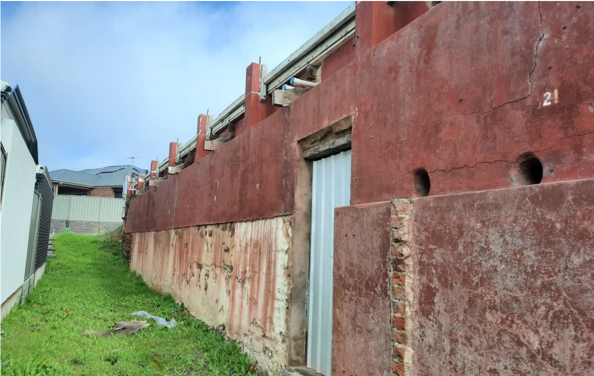
Painted rendered masonry wall to east elevation, formerly an interior wall, showing openings and painted numbers associated with former winery cellar fittings (GGA, 2021).
