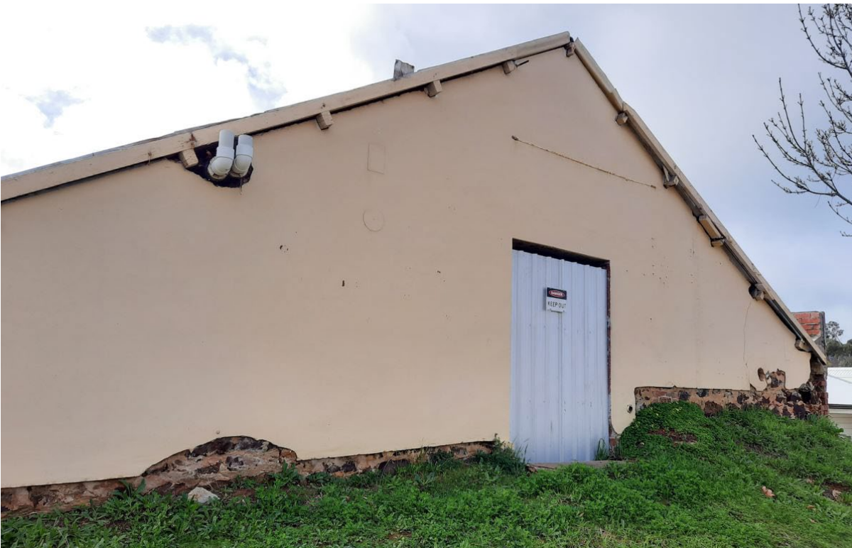
Rendered masonry wall to south elevation (GGA, 2021).
