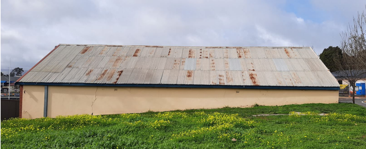
North west elevation of former cellar building at 20 Penfold Drive, McLaren Vale (GGA, 2021).
