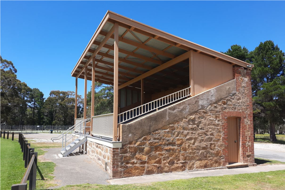
North and east elevations, looking south-west (GGA, 2021).
