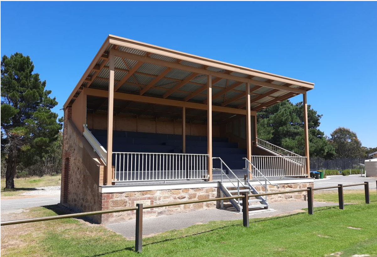
Kangarilla Oval Grandstand, 1988-1992 Kangarilla Road, Kangarilla (GGA, 2021)
