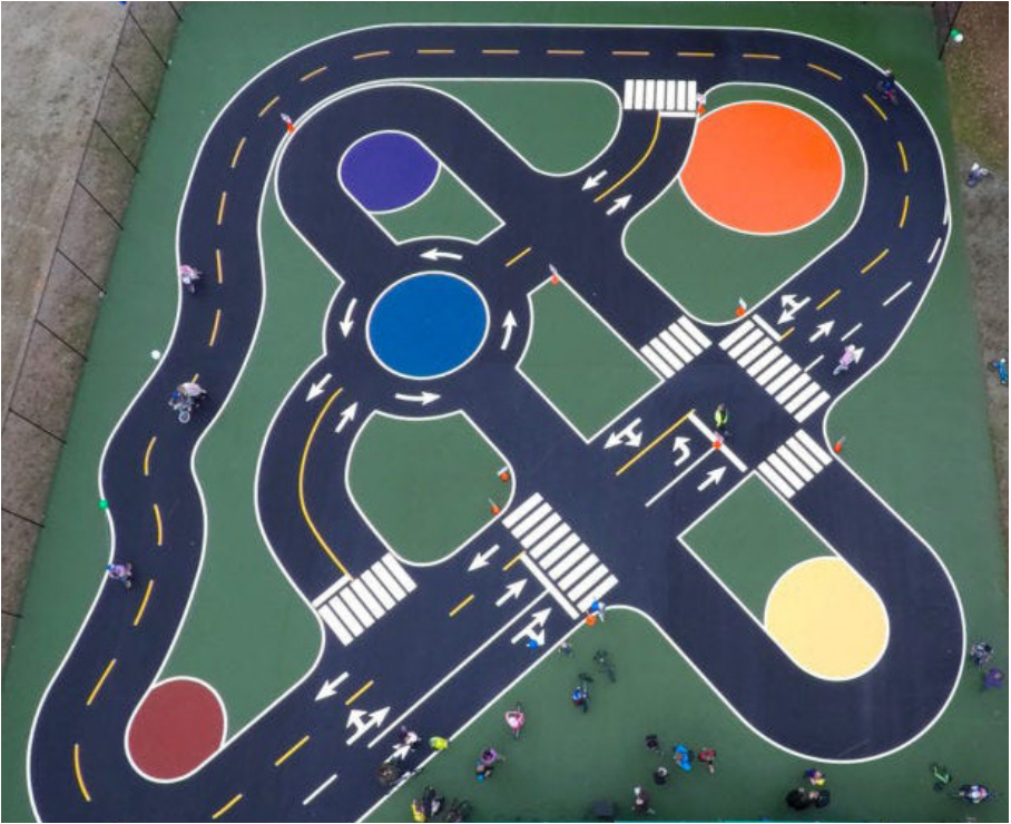
Bike Track Acrylic Surfacing and Linemarking
