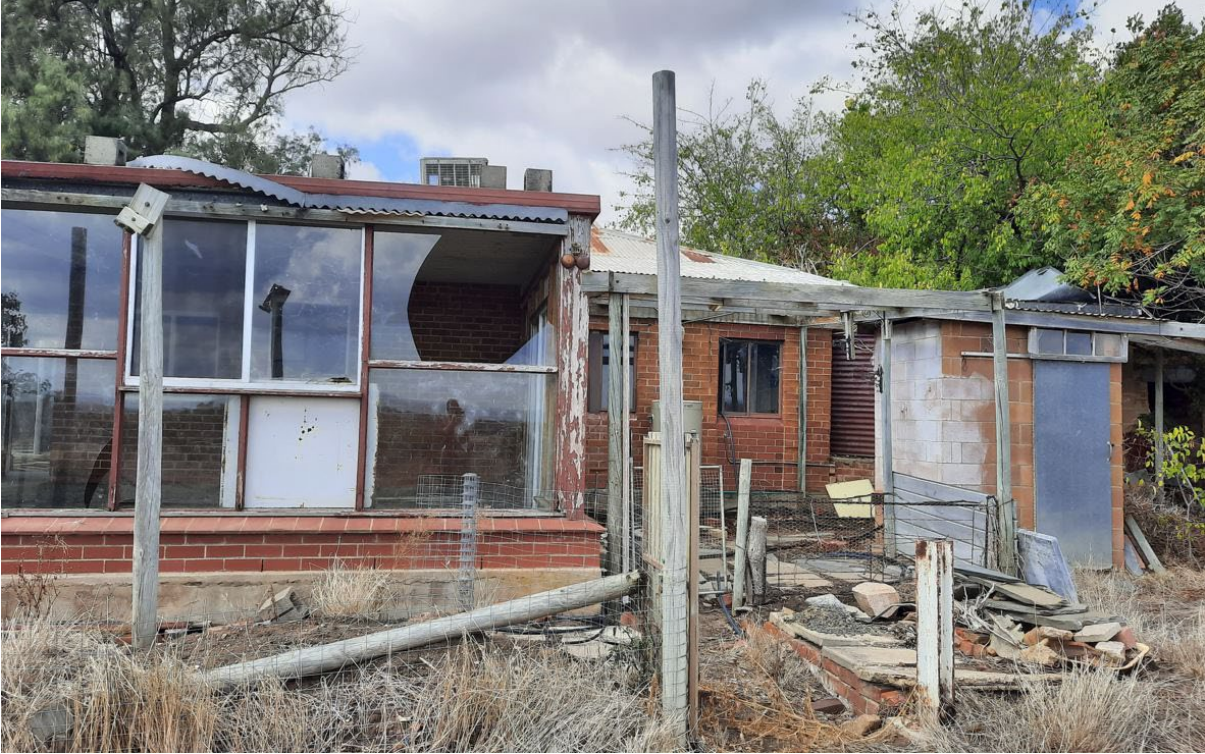
Various later additions to the east elevation, dating from the mid-20 th century onwards (GGA, 2022).
