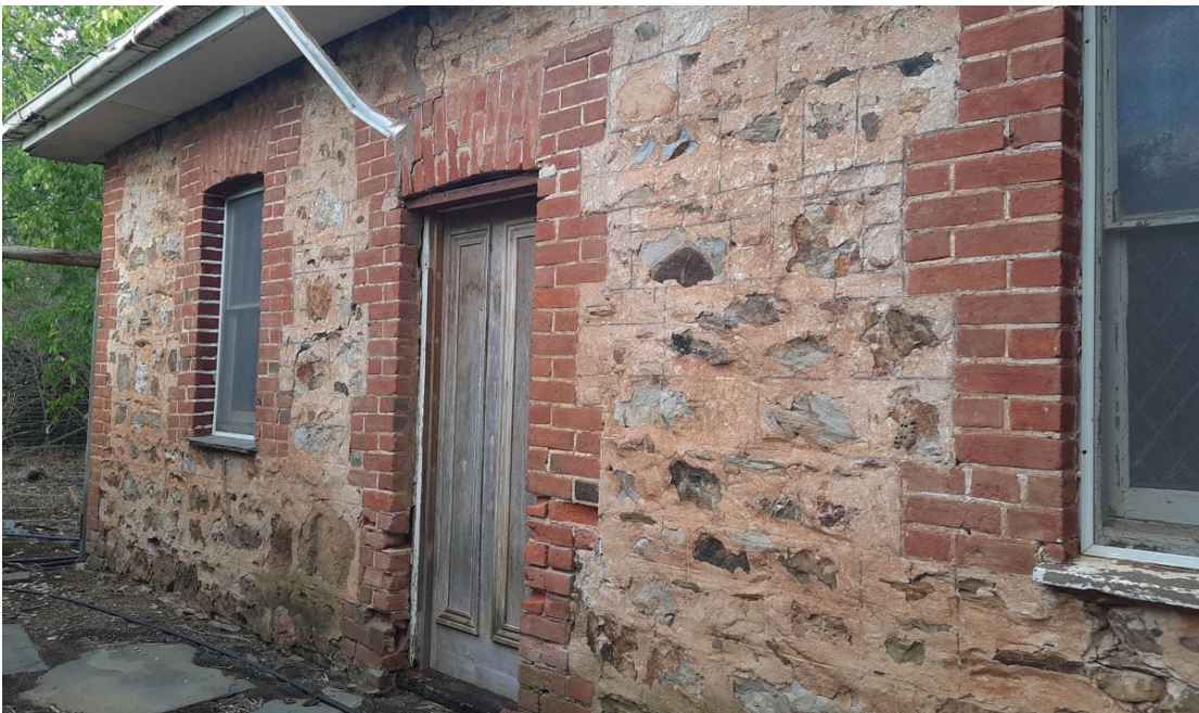
Primary west elevation of 402 Plains Road, Sellicks Hill (GGA, 2022)
