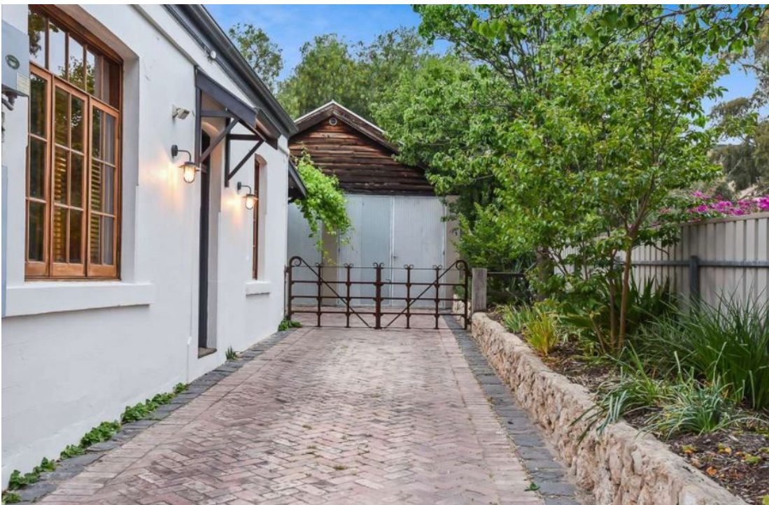
West elevation with external access, looking south ( https://www.realestate.com.au/property/60-patapinda-rd-old-noarlunga-sa-5168 , accessed 15/12/2021).
