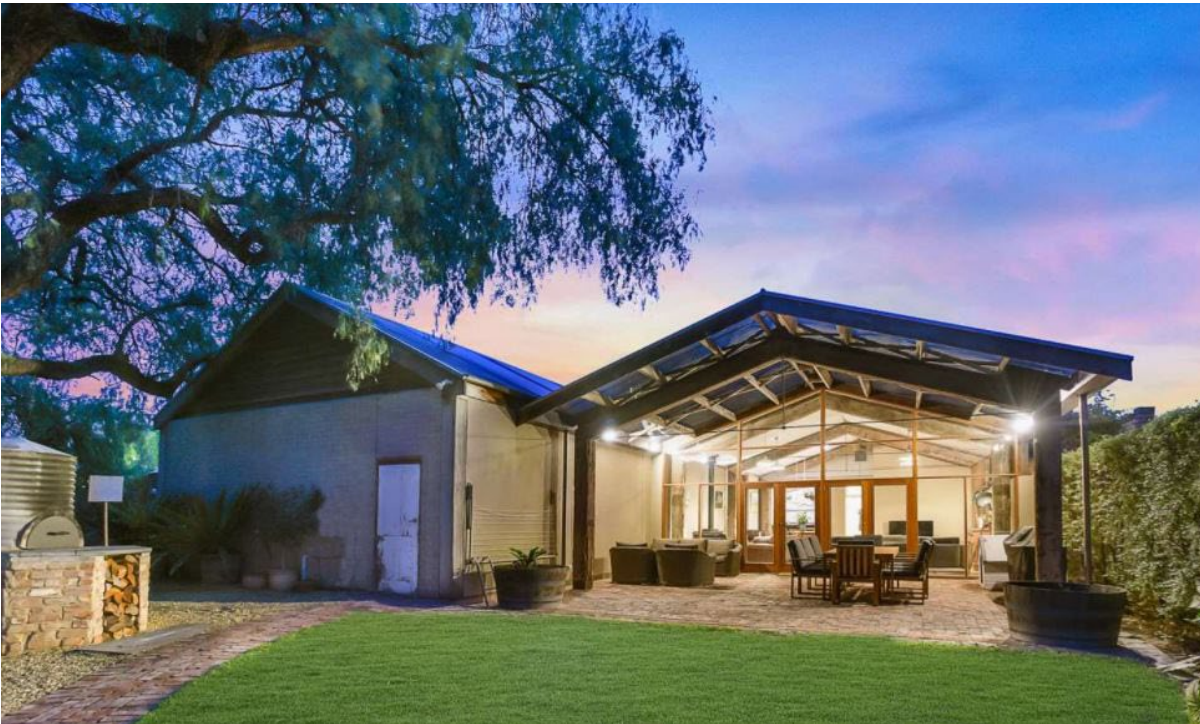
Late 20 th century shed and c.2010s residential additions completed prior to 2019. ( https://www.realestate.com.au/property/60-patapinda-rd-old-noarlunga-sa-5168 , accessed 15/12/2021).
