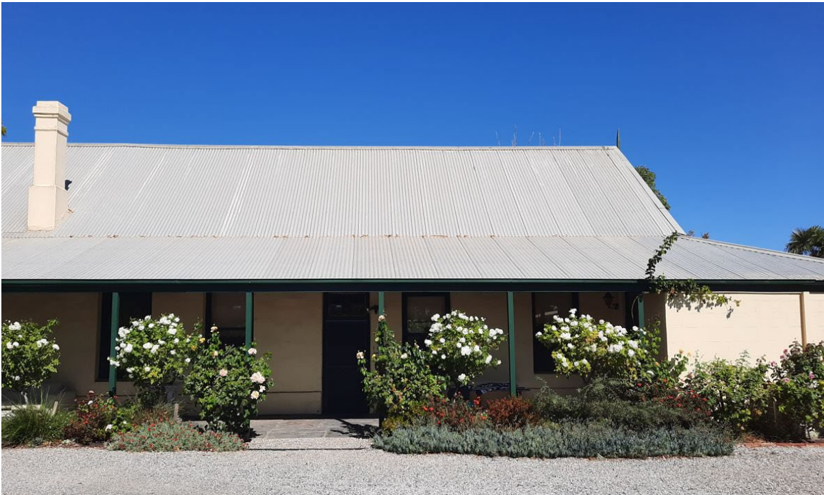
East elevation of 133 Little Road, Whites Valley, showing early fabric to the northern end of the elevation (GGA, 2022)
