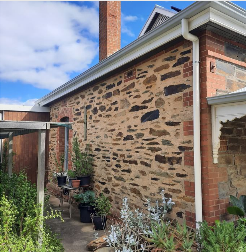
South elevation of 422 Main Road, Coromandel Valley (GGA, 2022)
