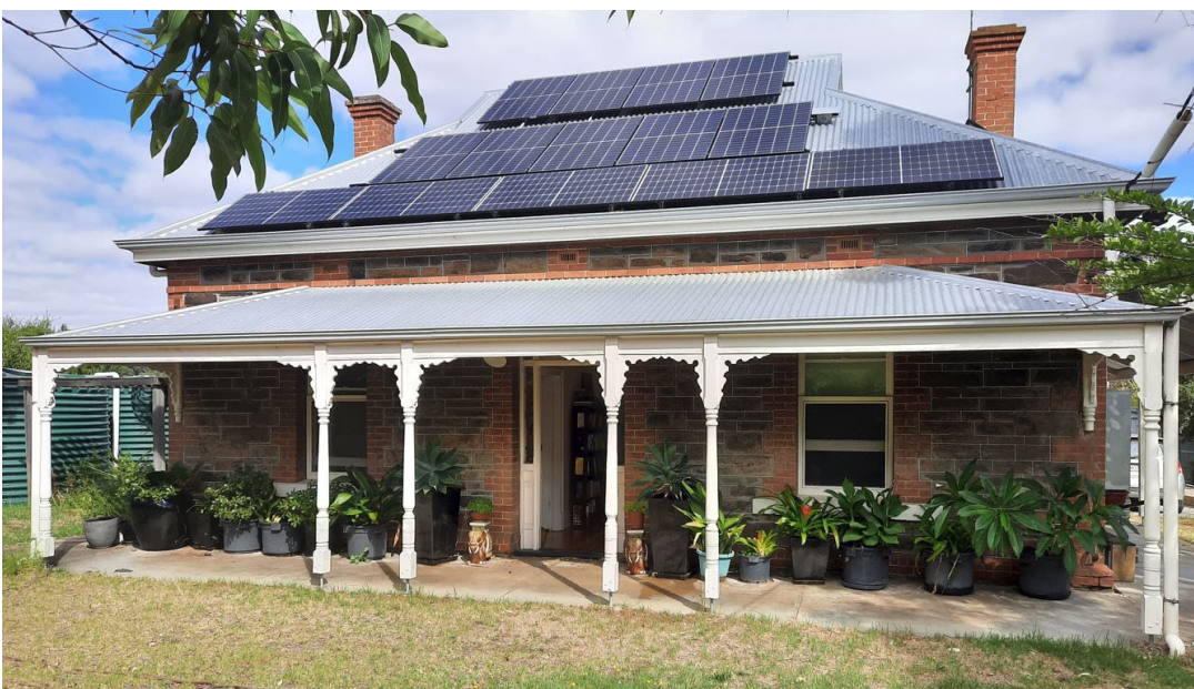
Primary east elevation of 422 Main Road, Coromandel Valley (GGA, 2022)
