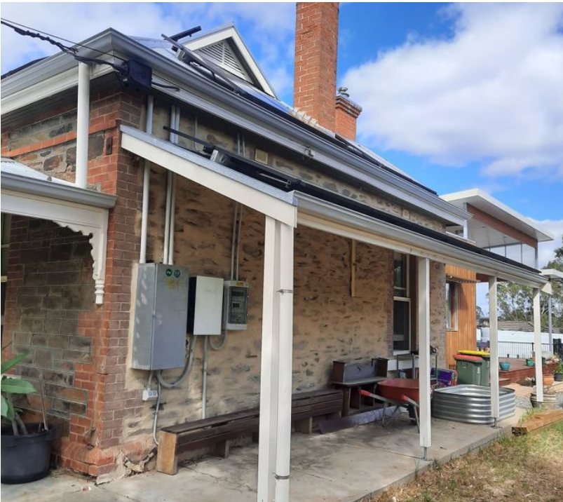
North elevation of 419 Main Road, Coromandel Valley, showing recent additions (GGA, 2022)
