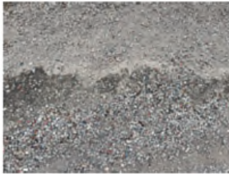
2) back of curved wall.
