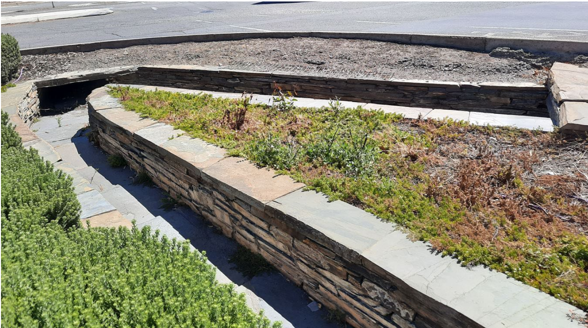
Slate culvert at the five-way intersection of High Street, Willunga; GGA, 2022)
