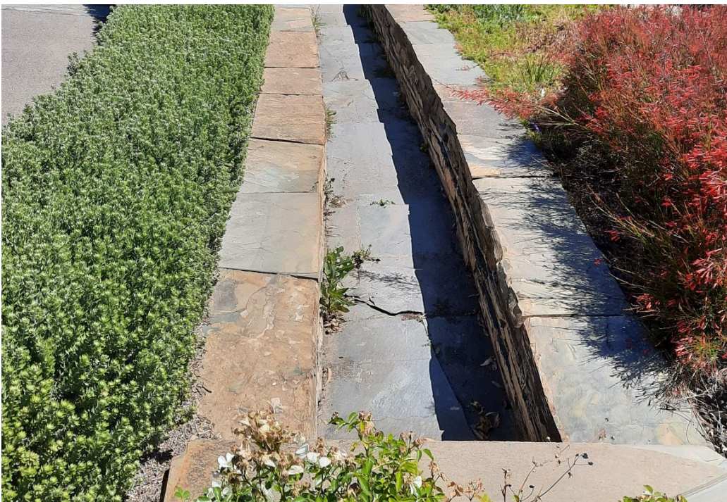
Slate fabric of the culvert dispensing from St Andrews Terrace towards Aldinga Road, looking north (GGA, 2022).
