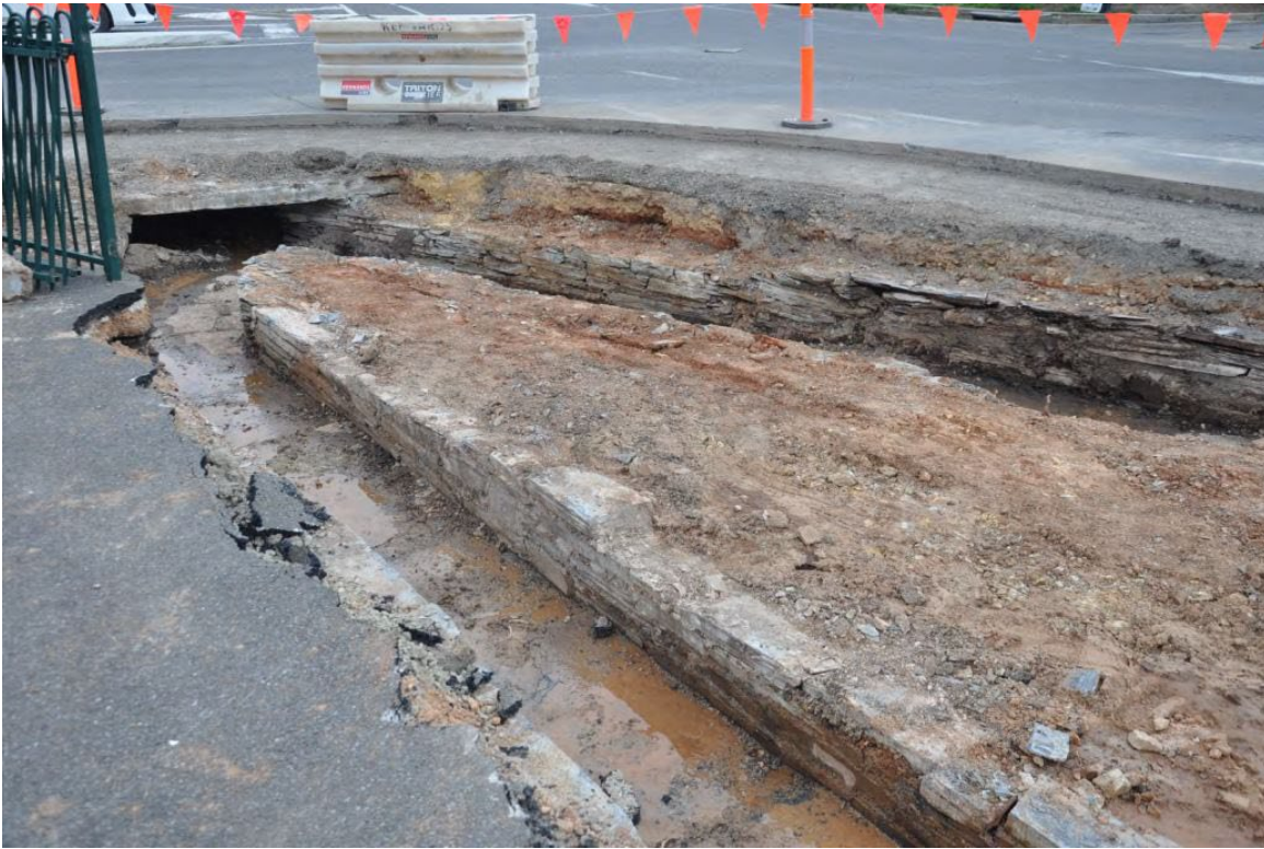
2017 photograph of then recently-excavated slate culverts at High Street five-way intersection, uncovered during the Willunga streetscape project (National Trust of SA, Willunga Branch)
