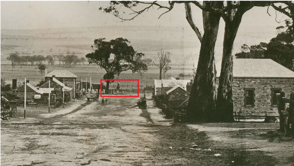
C.1870 photograph of site of five-way intersection slate culvert at the bottom of High Street, Willunga (site shown within red rectangle). Note excavated lines of earth on either side of High Street, indicating completion of recent subterranean drainage culverts at that time. There appears to be a small footbridge over the site of the slate culvert, possibly the 'infant bridge' referred to in the 1865 article. (SLSA B 7192)
