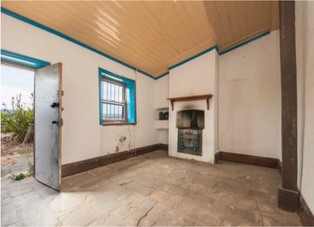
Internal fittings to the lean-to kitchen, including early stove and chimney, matchboard ceiling and slab stone flooring. ( https://www.realestate.com.au/property/1527-1531-main-south-rd-ohalloran-hill-sa-5158 , accessed 15/3/2022).
