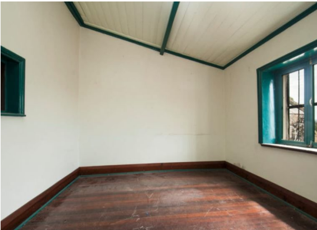
Internal fittings to lean-to room, including matchboard ceiling and early window forms and elements. ( https://www.realestate.com.au/property/1527-1531-main-south-rd-ohalloran-hill-sa-5158 , accessed 15/3/2022).
