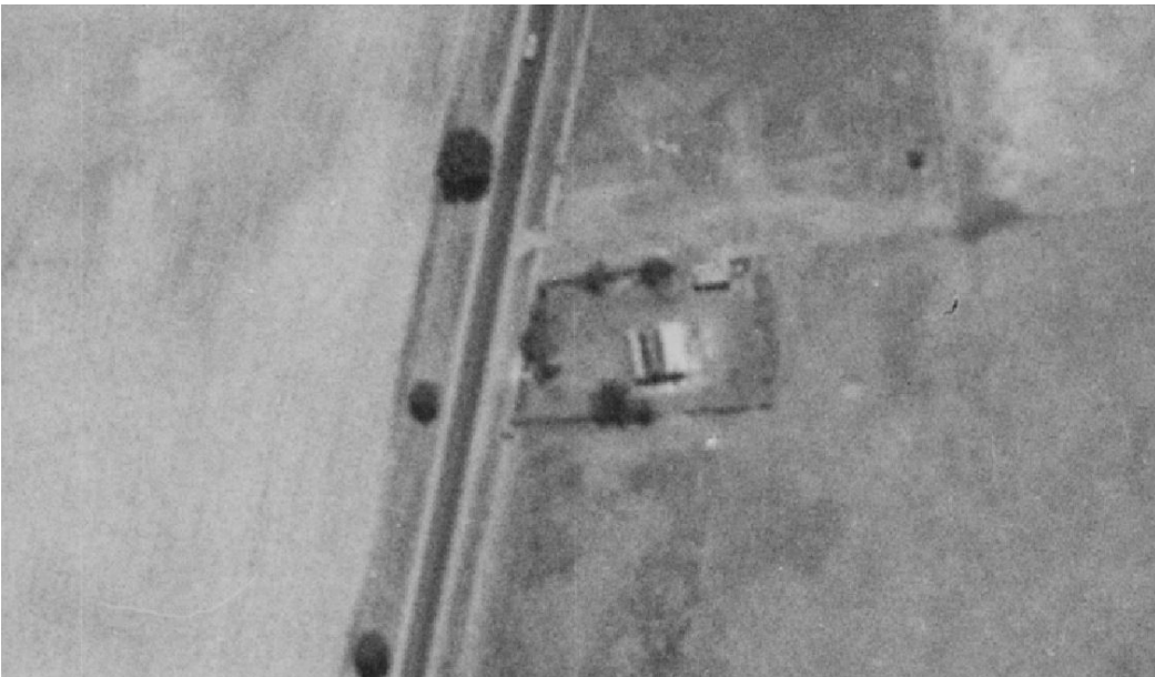
Aerial photo of site of 1527-1531 Main South Road, O'Halloran Hill in 1936 (ICSM Historical Aerial Photography, Film Number MAP1942, Run 4N, Frame 6341, dated 3rd April, 1936. ( https://aerialphotography-geoscience-au.hub.arcgis.com/apps/7f5d281e06be4934b493175fd76d33da/explore , accessed 15/3/2022).
