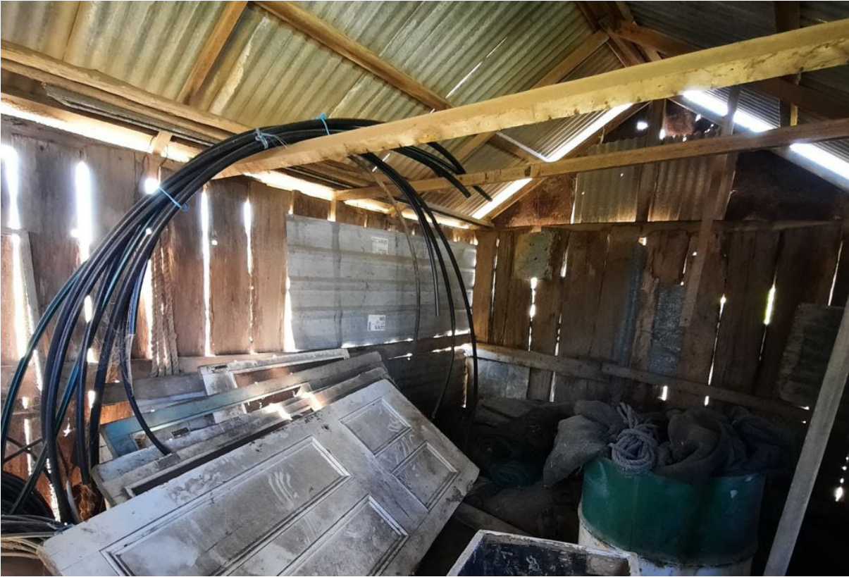
Early slab timber shed interior with later timber structure and corrugated steel cladding (GGA, 2021).
