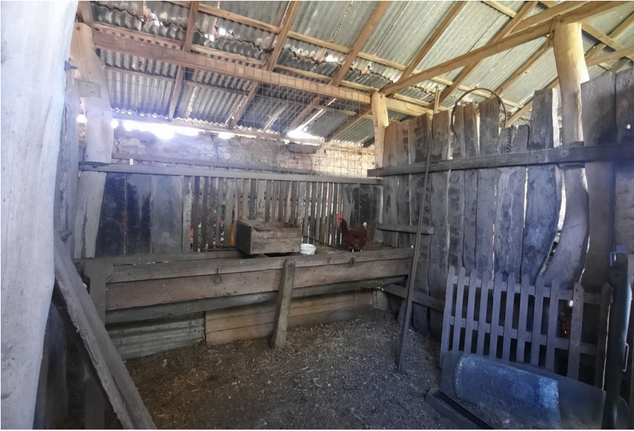
Early slab timber stalls and mangers to stable complex (GGA, 2021).
