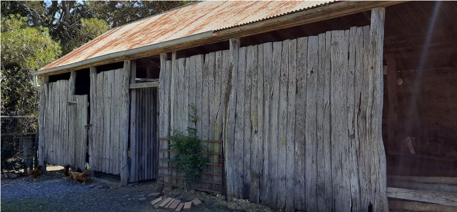
Early external slab timberwork to south elevation of stabling complex (GGA, 2021).
