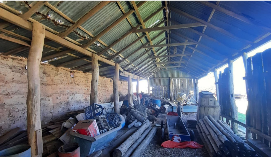
Early masonry construction and slab timberwork to stabling complex (GGA, 2021).
