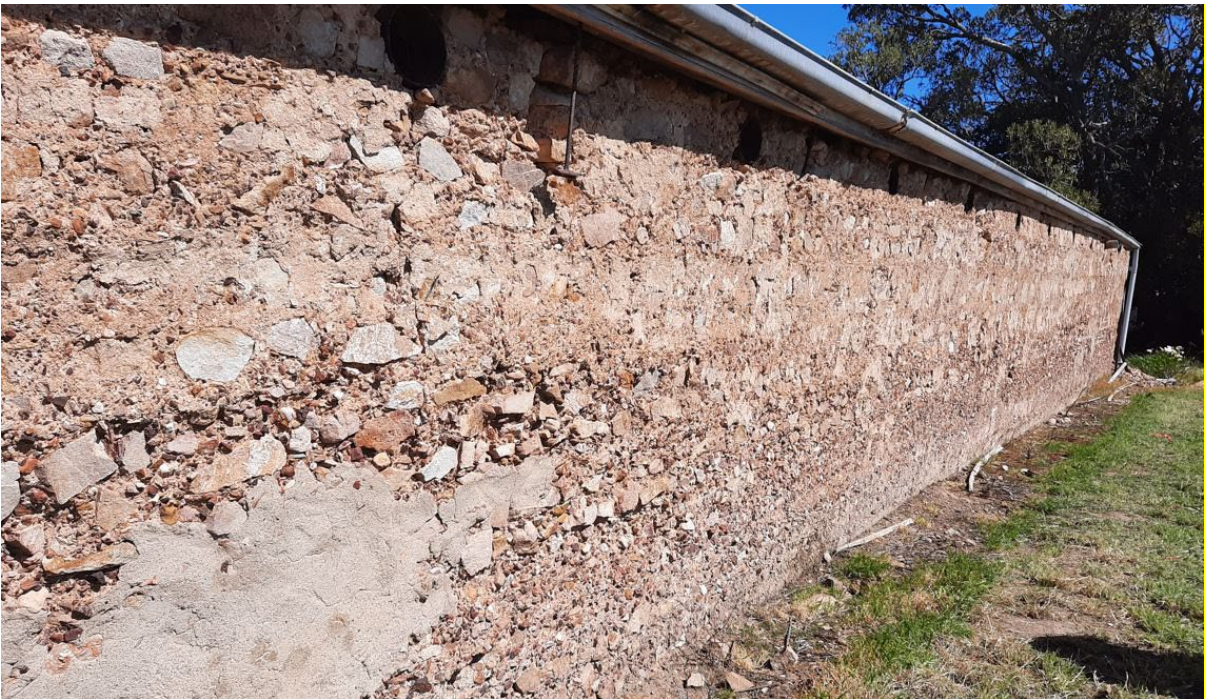
North masonry wall of stabling complex (GGA, 2021).
