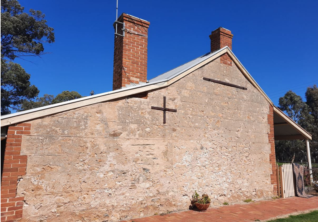
North elevation of c.1850 former farmhouse, including early cast-iron wall plates (GGA, 2021).
