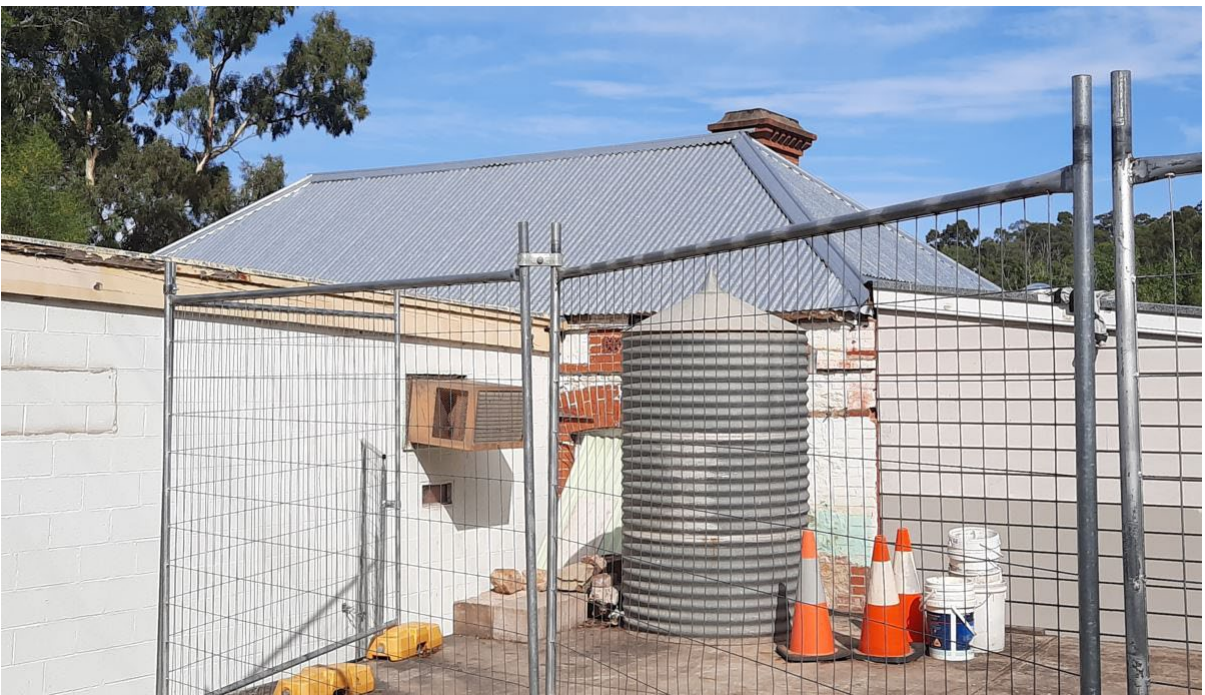
East elevation c.1902 cottage, showing current restoration work, including re-roofing with corrugated steel and external masonry repairs (GGA, 2022)
