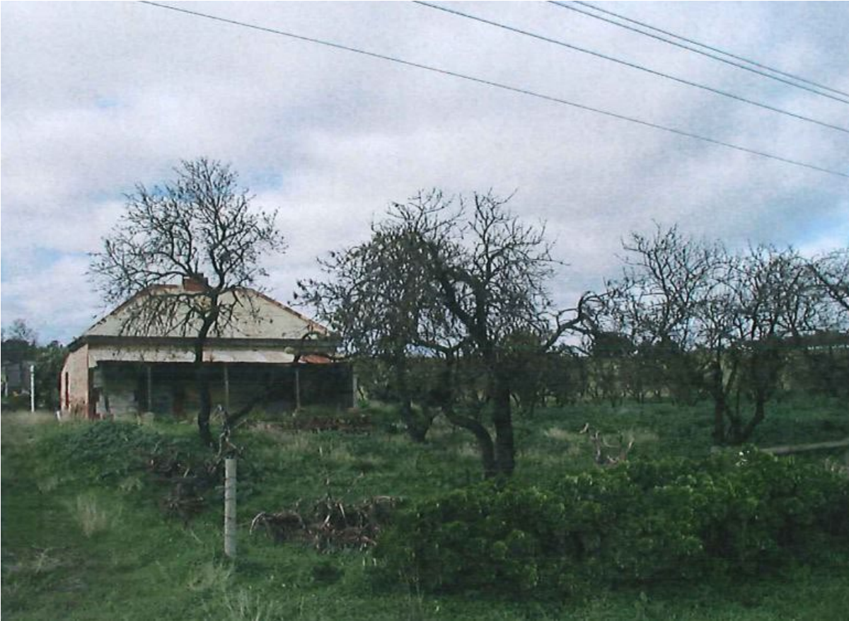
North west elevation of former farmhouse in 2003, then in dilapidated condition (2003 Noarlunga Local Heritage Register)
