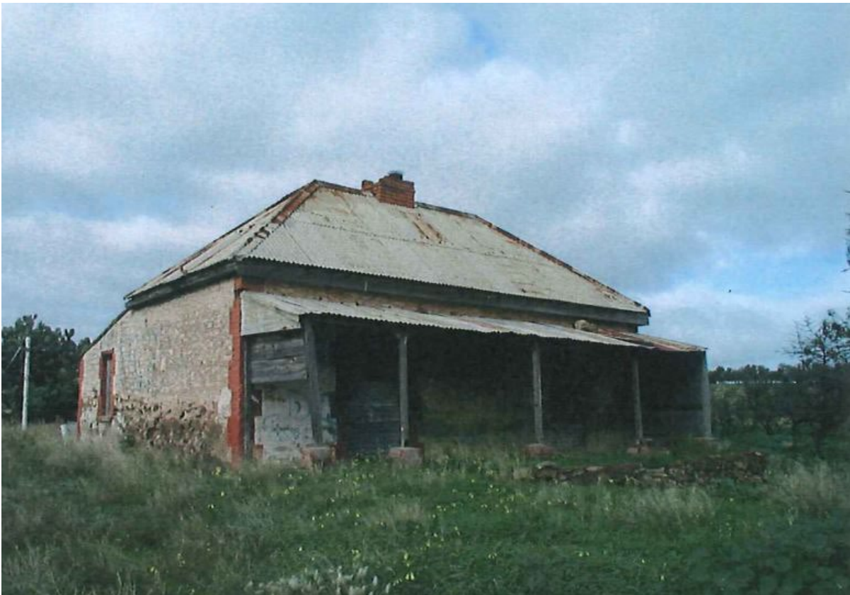
North west elevation of former farmhouse in 2003, then in dilapidated condition (2003 Noarlunga Local Heritage Register)
