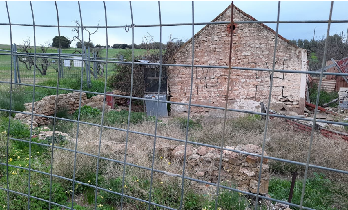
East elevation of early outbuilding with courtyard retaining wall and boundary fencing (GGA, 2021).
