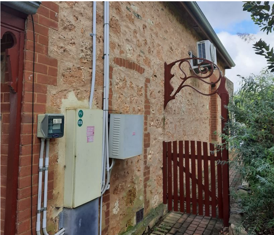
Early stonework and brickwork to south wall of c.1912 residence; it is possible that elements of a late-19 th century residence formerly associated with the late 19 th century chaff mill were incorporated into the c.1912 building, as this wall suggests. (GGA, 2022)
