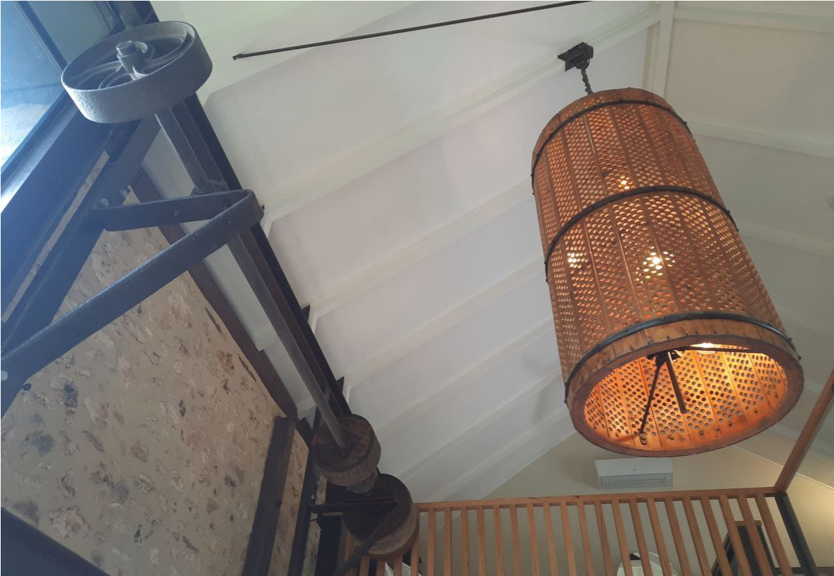
Early industrial fabric relating to the chaff mill's function, retained and incorporated into the c.2014 reconstruction works (GGA, 2022)
