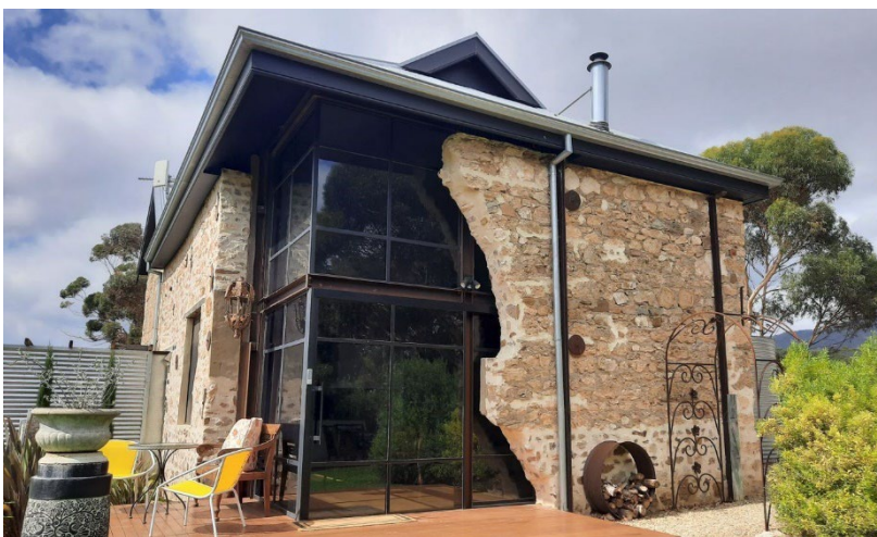
Residence (above) and former chaff mill (below) at 371 Plains Road, Sellicks Hill (GGA, 2022)
