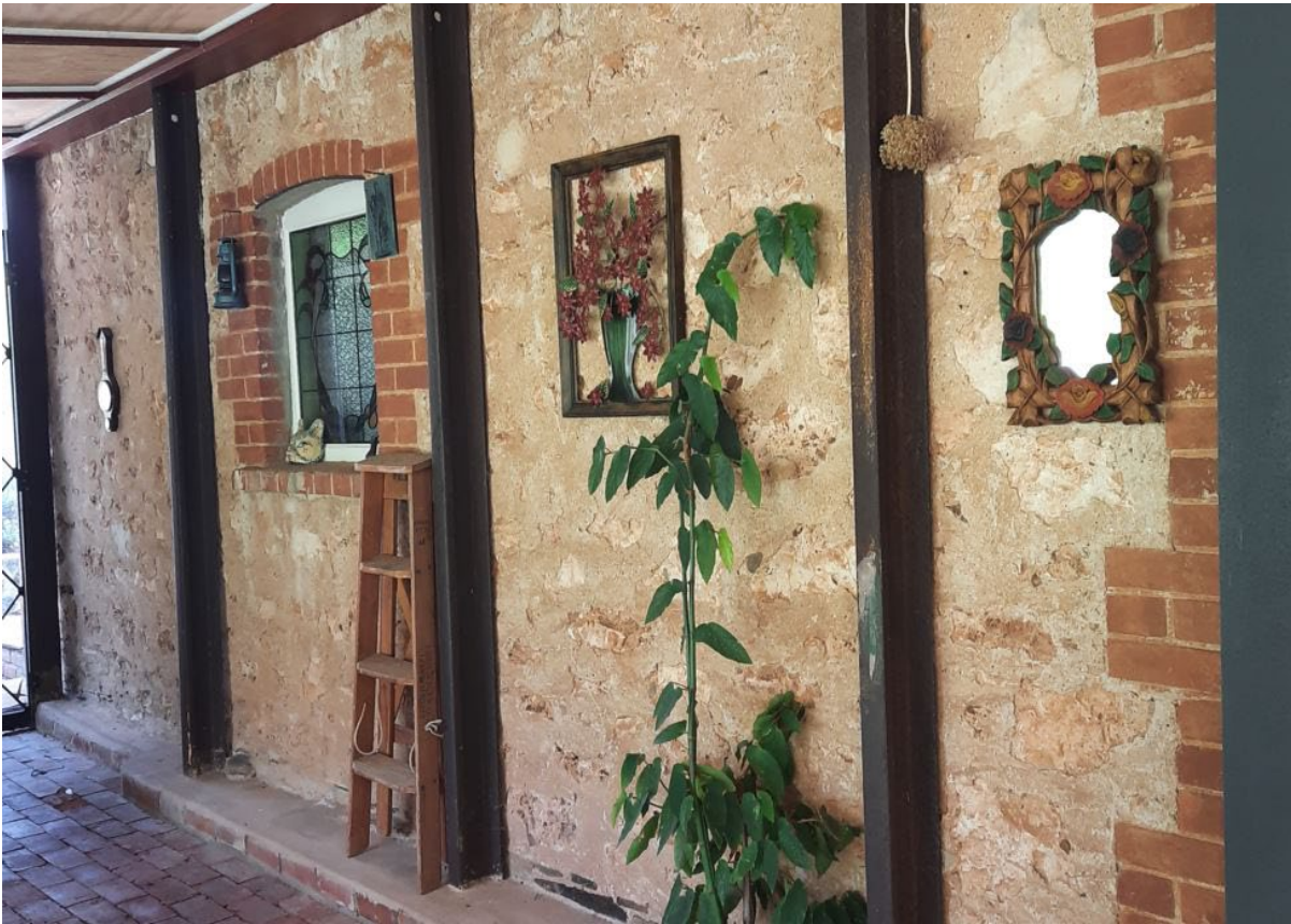
Masonry fabric associated with the 'lean-to' additions to the west elevation, (GGA, 2022)
