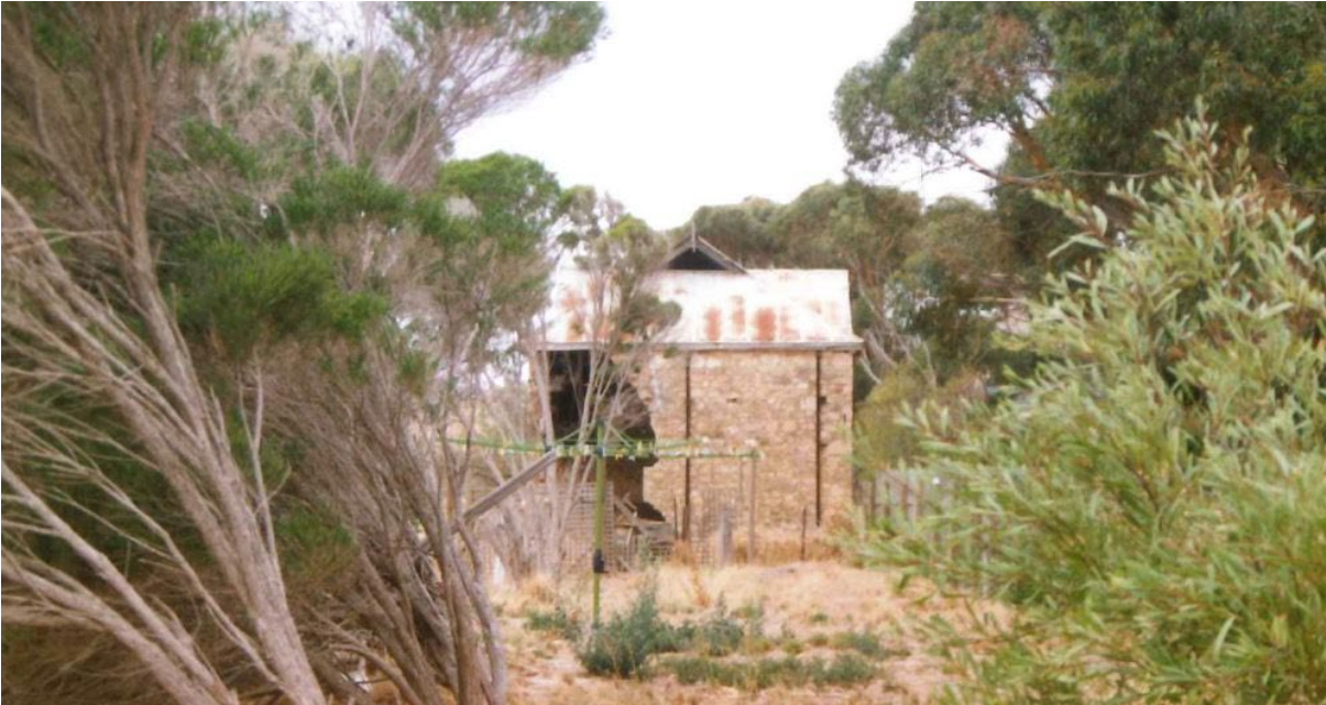
Former chaff mill at 371 Plains Road, Sellicks Hill, (McDougall & Vines, 1997, Willunga District Heritage Survey, p. 210).
