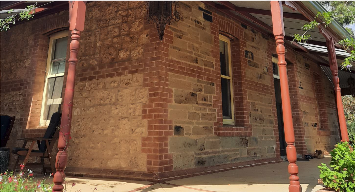
Differing stonework to c.1912 residence; it is possible that elements of a late-19 th century residence formerly associated with the late 19 th century chaff mill were incorporated into the c.1912 building (GGA, 2022)
