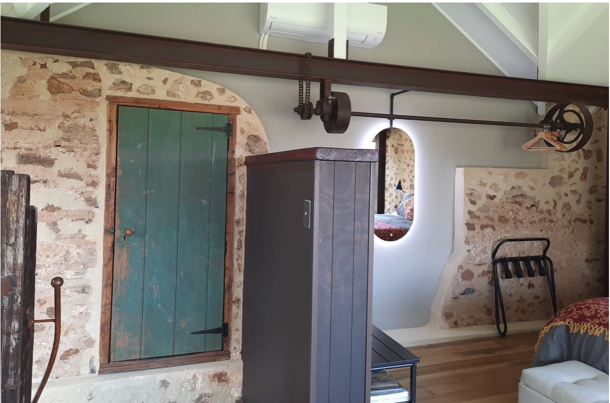
Early masonry and timber fabric to former chaff mill, now with later reconstructed elements dating to c.2014 (GGA, 2022)
