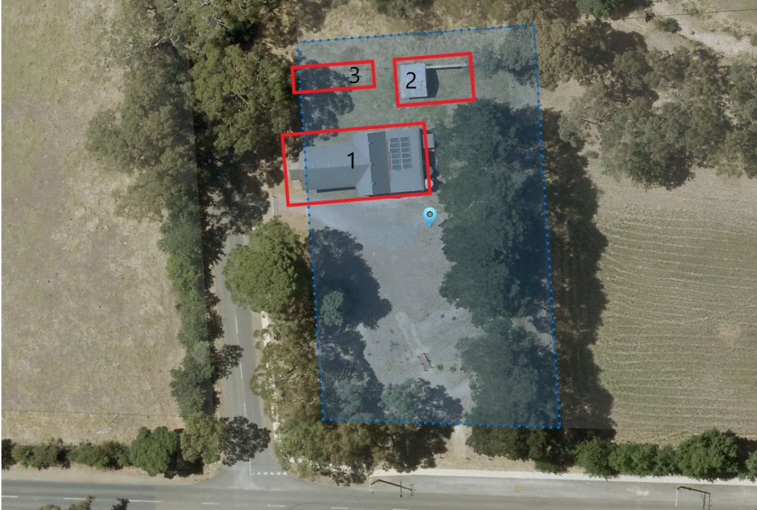
Site of heritage elements at 1 McLaren Flat Road, Kangarilla; (1) chapel (2) outbuilding and hitching wall; (3) relocated early gravestones (Planning SA SAPPa)
