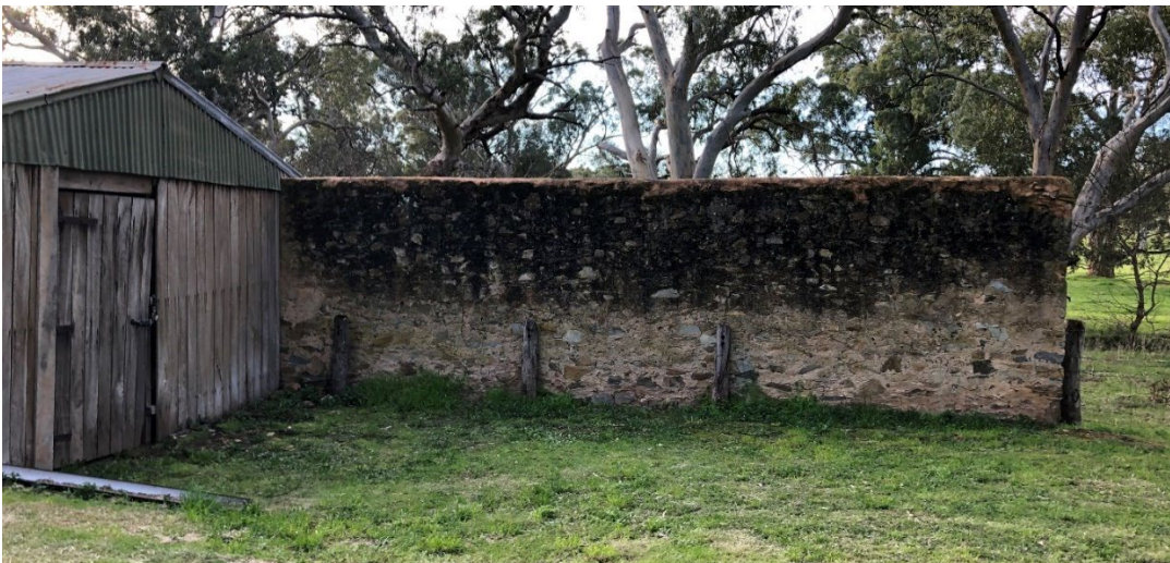
Outbuilding wall at 1 McLaren Flat Road, Kangarilla (GGA, 2021)
