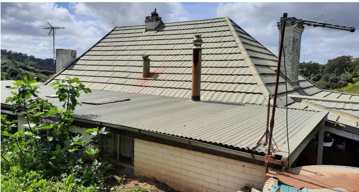
West elevation, including c. mid-20 th century masonry additions. Original slate tiling (evident in image SLSA B 35564 removed with replacement aluminium tiling; original roof structure appears to be intact (GGA, 2021).
