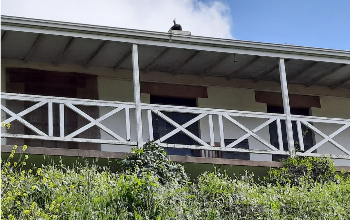
C.1850 original door and window openings, possibly retaining early fittings (GGA, 2021).
