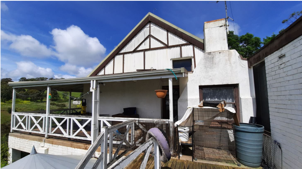
North elevation of 24 Chalk Hill Road; reconstructed north gable roof with c. mid-20 th century masonry verandah and timber framed covered verandah roof after 1983; original form of masonry chimney now rendered. (GGA, 2021).
