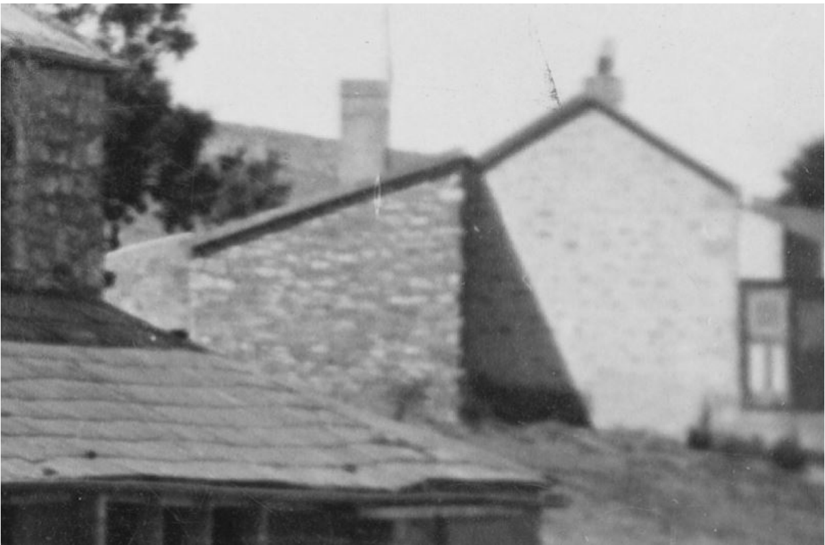
West elevation of former Harbour Master's cottage in 1933 (SLSA, B 8885).
