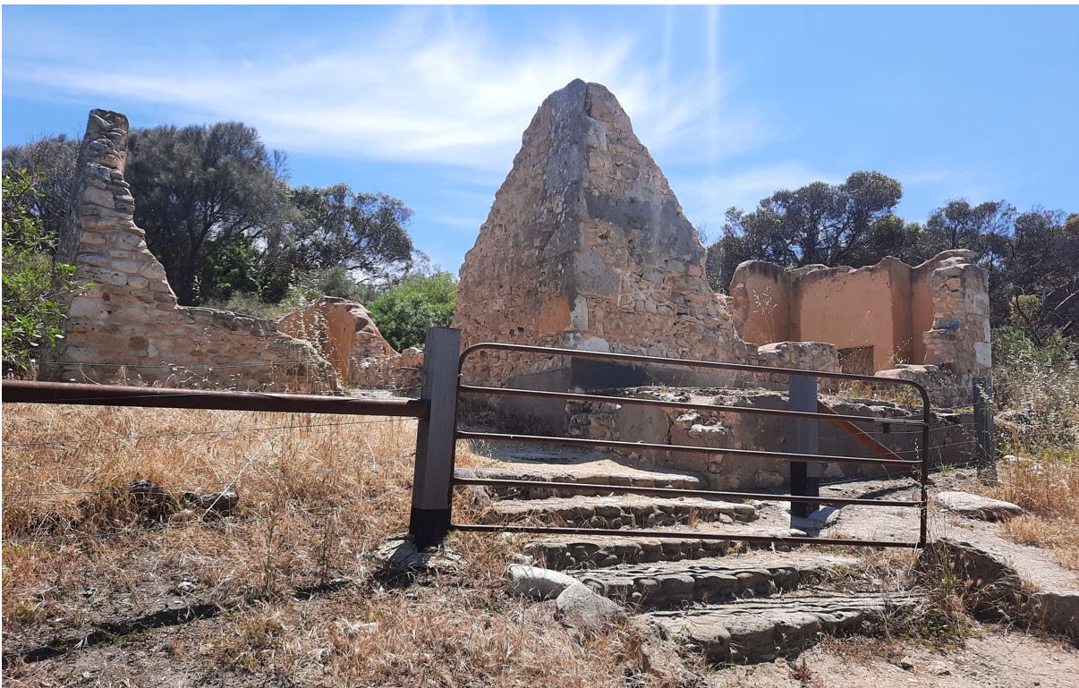
Former Harbour Master's Cottage ruins, Lot 22 Water Street, Port Willunga looking north (GGA, 2021)
