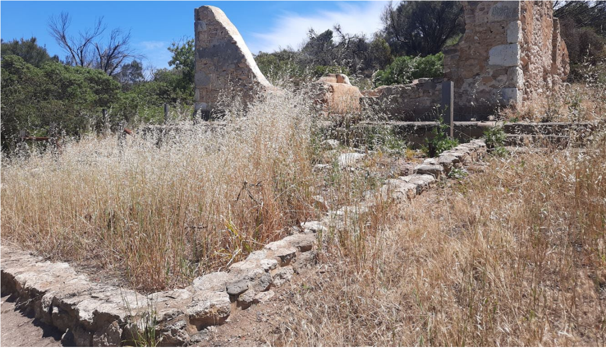
Former Harbor Master's cottage ruins, looking north; freestone retaining walls and verandah plinth to immediate south of former cottage (GGA, 2021).
