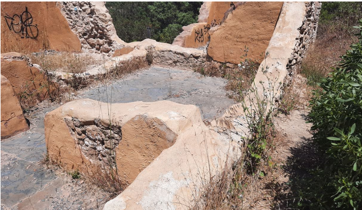
Former Harbour Master's cottage ruins, looking south-west; original slate paved flooring to various former rooms (GGA, 2021).
