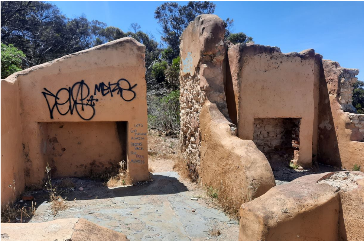
Former Harbour Master's cottage ruins, looking east; former fireplace surrounds with later painted render (GGA, 2021).
