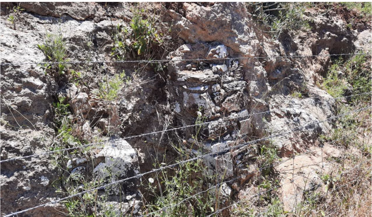
Constructed retaining wall element to Old Sellicks Hill Road, possibly dating to the initial 1850s construction period (GGA, 2022)
