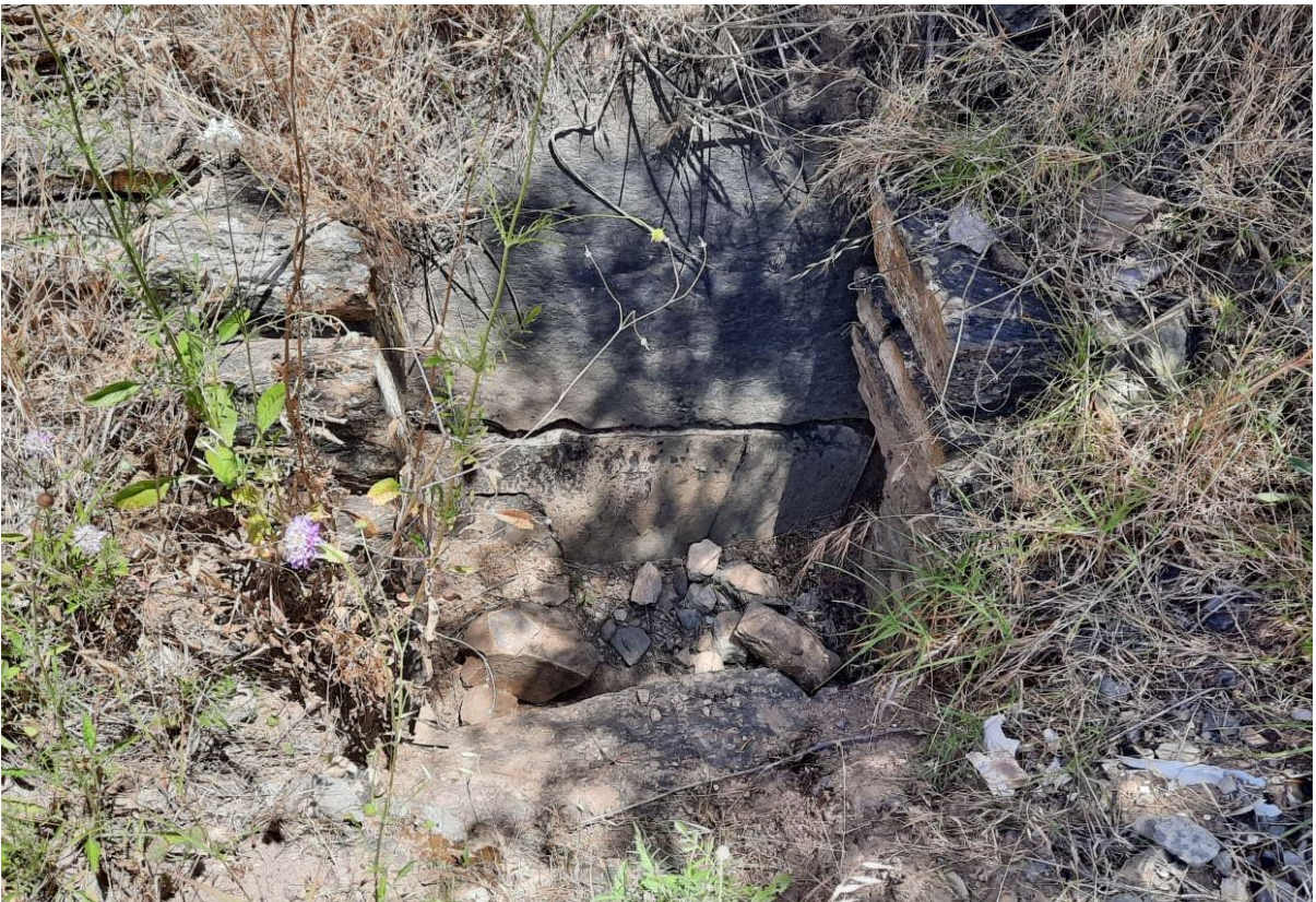
Slate culvert running beneath Old Sellicks Hill Road (GGA, 2022).
