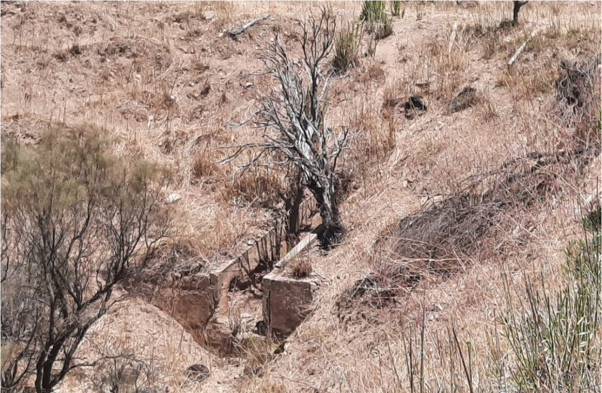
Masonry fabric associated with early culvert under corner of Old Sellicks Hill Road, some later concrete fabric (GGA, 2022)
