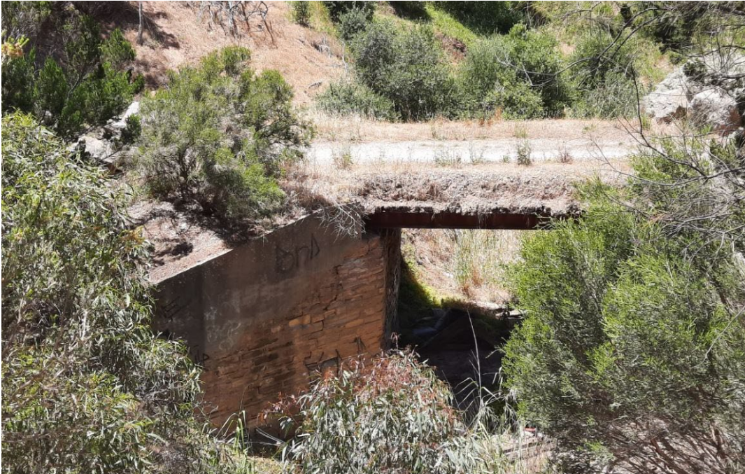
Masonry fabric and steel girders of Pedler's Creek Bridge, Old Sellicks Hill Road, looking east (GGA, 2022)
