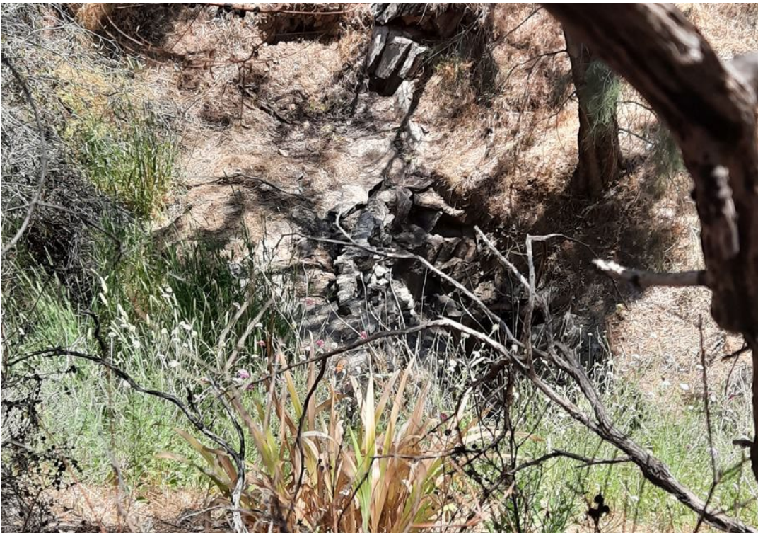
Masonry fabric of old slate weir immediately north-west of Pedler's Creek Bridge, looking south (GGA, 2022)
