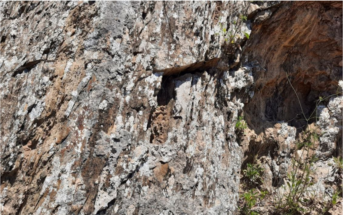
Excavations to Old Sellicks Hill Road, gouged hole in stone possibly relates to dynamite insertion (GGA, 2022).
