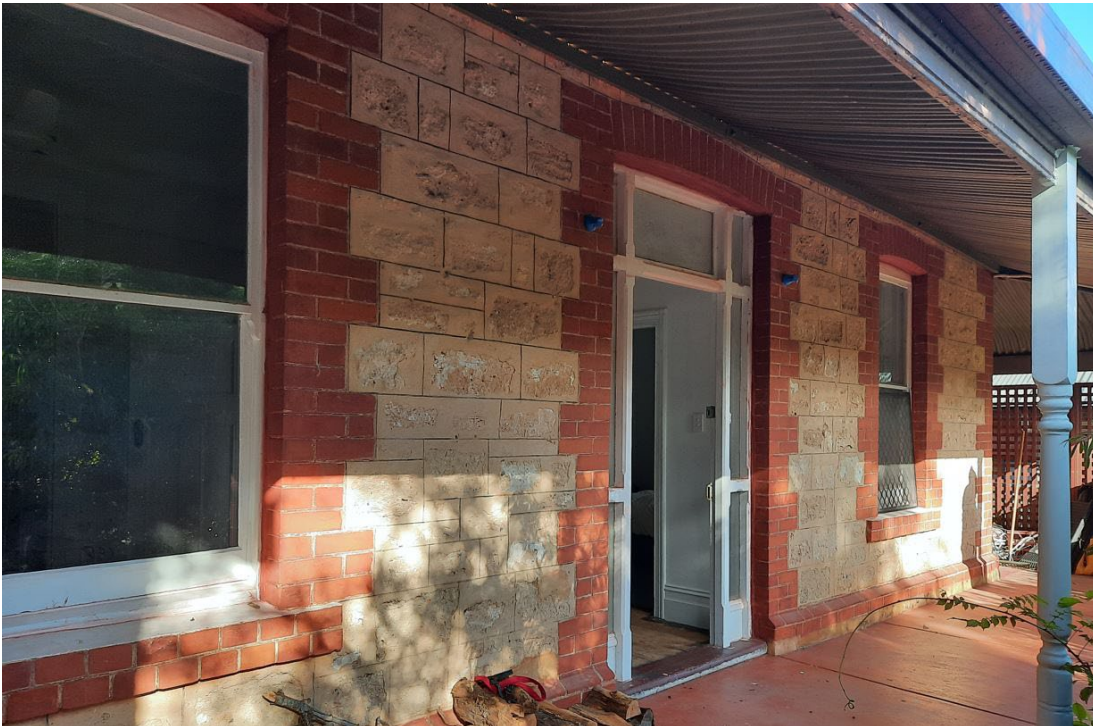
Primary façade of the c.1915 portion of 4 Oval Road, Old Reynella (GGA, 2022).
