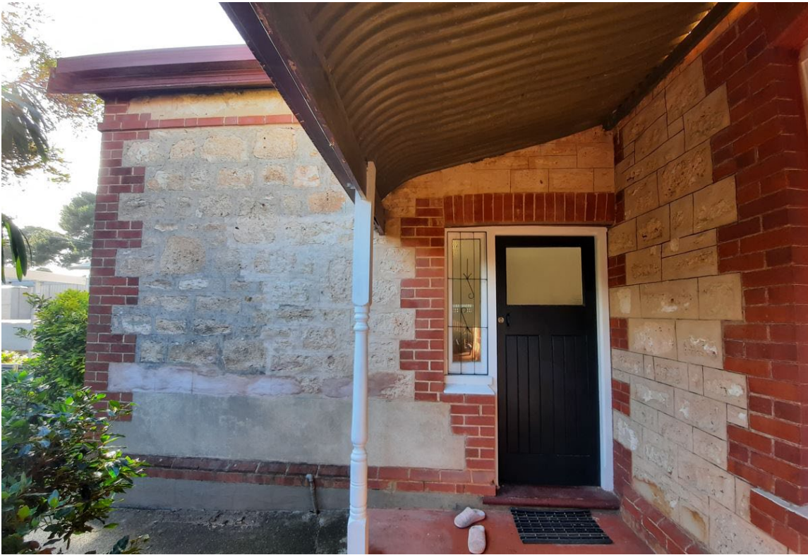
Joint between 1915 building and c.mid-1920s additions, looking east (GGA, 2022).
