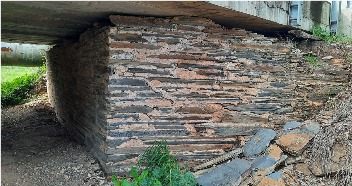
Southern slate abutment at Almond Grove Road, Whites Valley (GGA, 2021).
