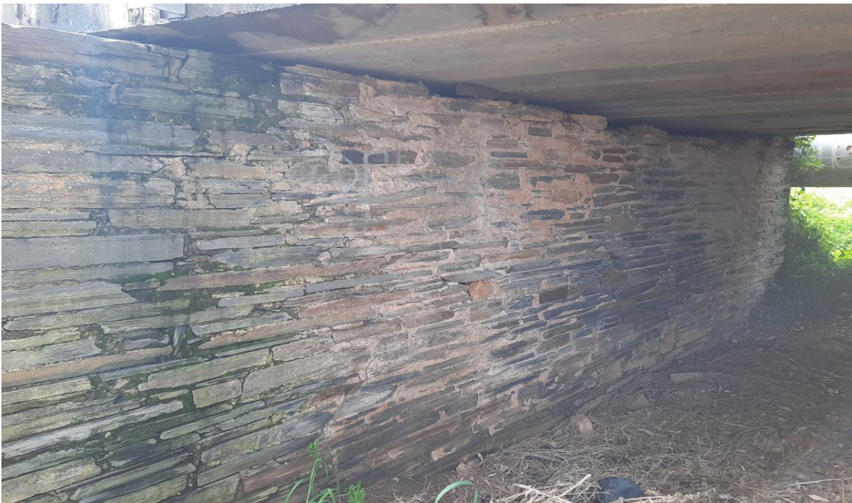
Northern slate abutment at Almond Grove Road, Whites Valley (GGA, 2021).
