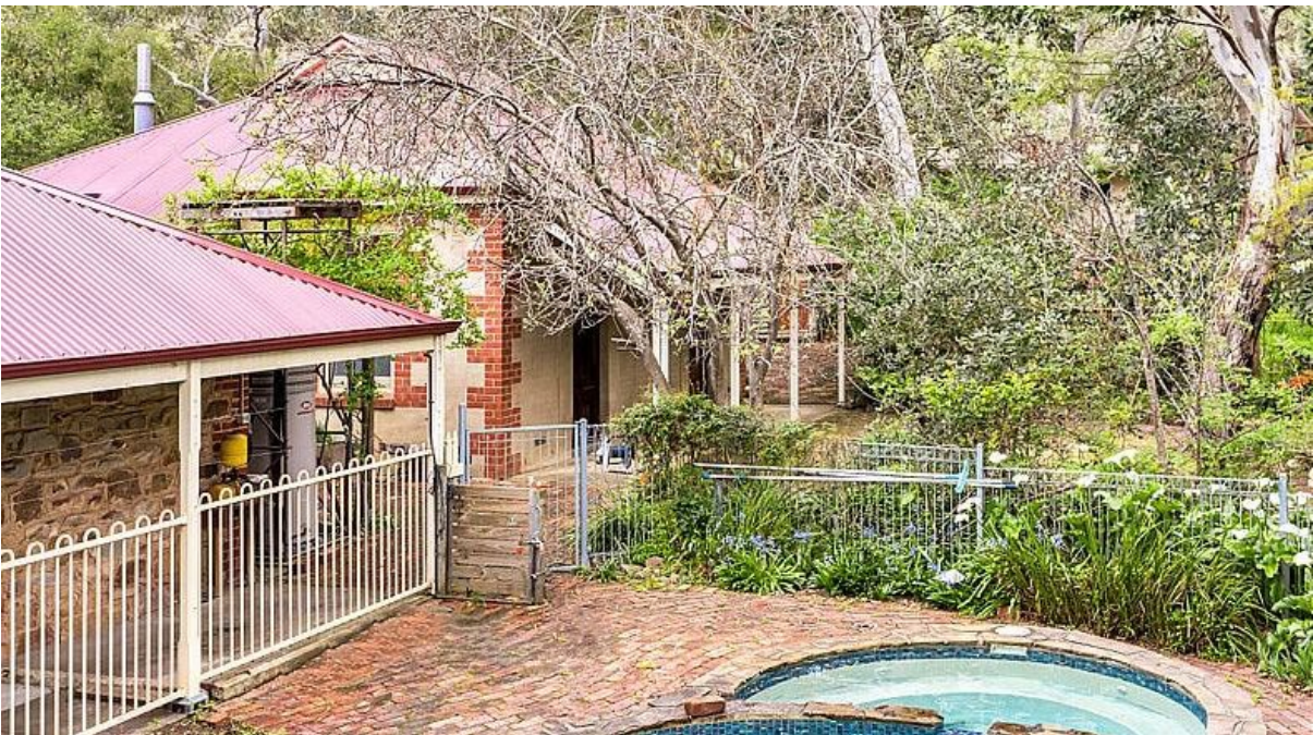
Later additions joining early fabric of c.1898 residence to the east elevation ( https://www.realestate.com.au/property/419-main-rd-coromandel-valley-sa-5051 , accessed 7/4/2022)
