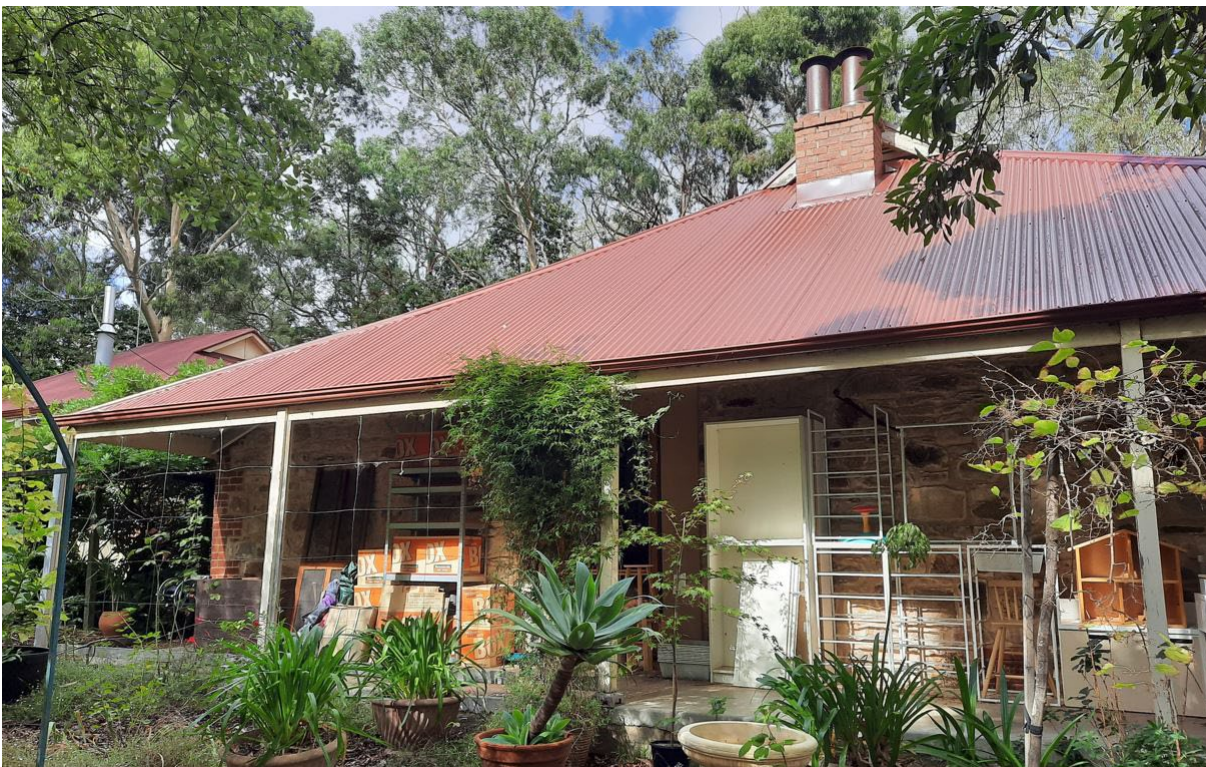
North elevation of 419 Main Road, Coromandel Valley (GGA, 2022)
