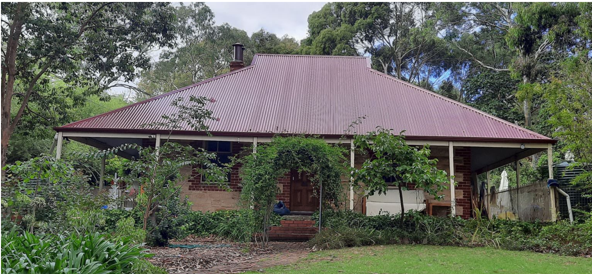
Primary west elevation of 419 Main Road, Coromandel Valley (GGA, 2022)
