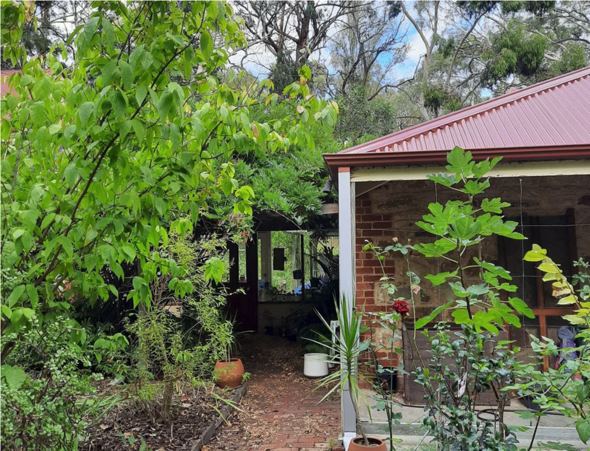
Later additions joining early fabric of c.1898 residence to the east elevation (GGA, 2022)
