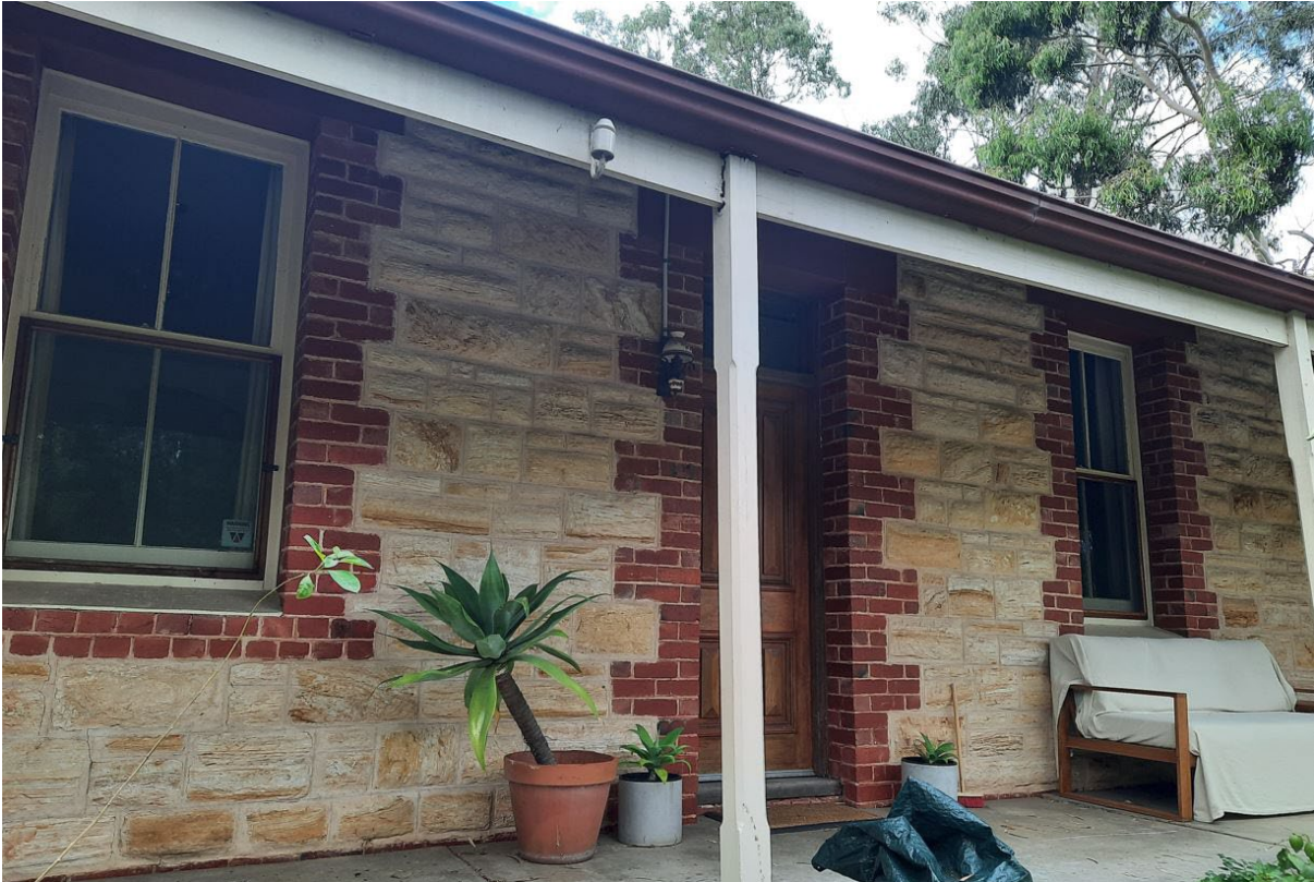
Primary west elevation of 419 Main Road, Coromandel Valley, showing historic fabric of early timber door and windows (GGA, 2022)
