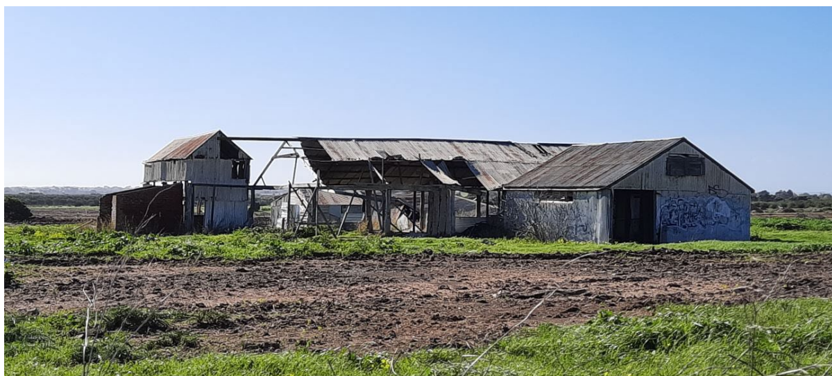
Barn/shed ruins at Allot. 353, Sec. 610 Rogers Road, Sellicks Hill (GGA, 2021)
