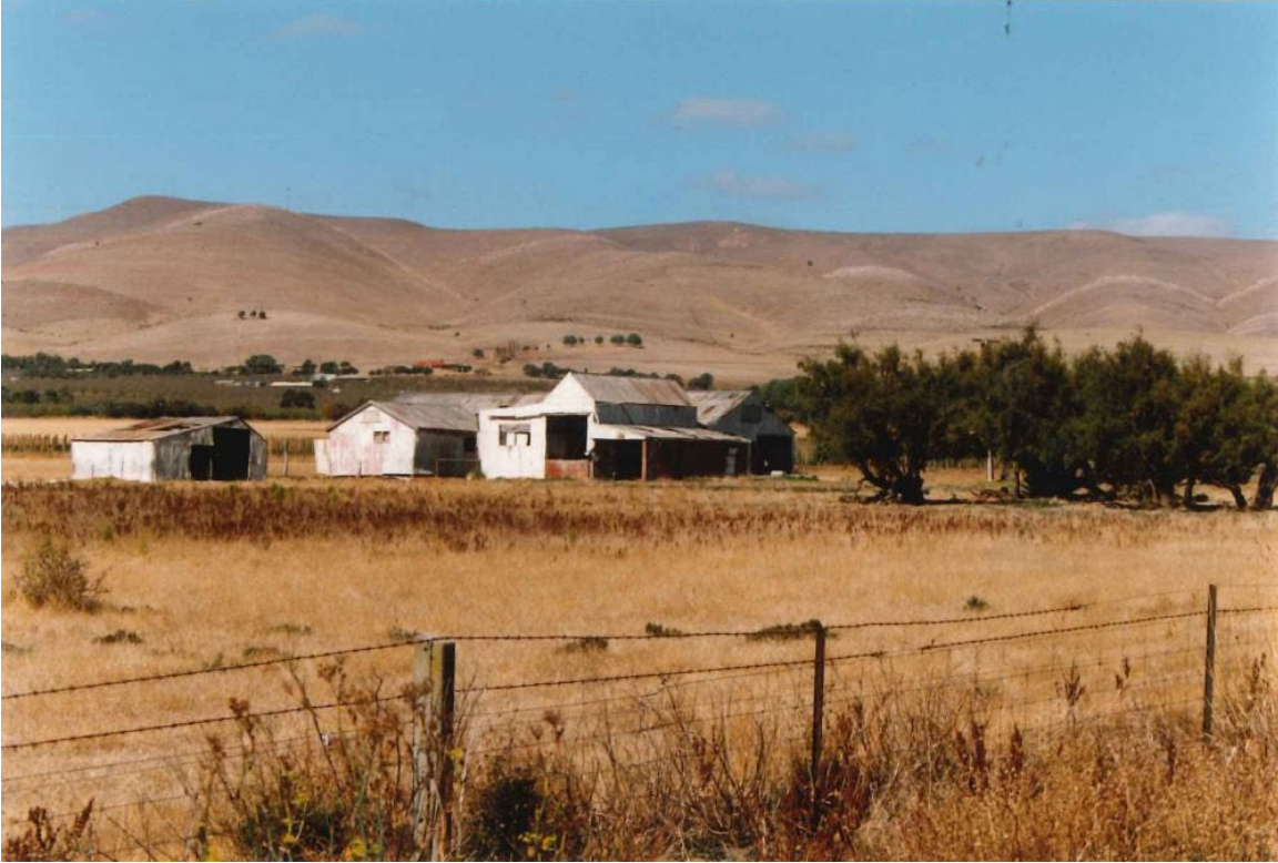
Barn/sheds at Lot 353, Section 610 Rogers Road, Sellicks Hill in 1997, extensive deterioration has occurred since then ( Willunga District Heritage Survey )
