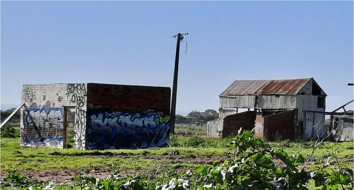
Extensive graffiti to ruined masonry outbuildings (GGA, 2021)
