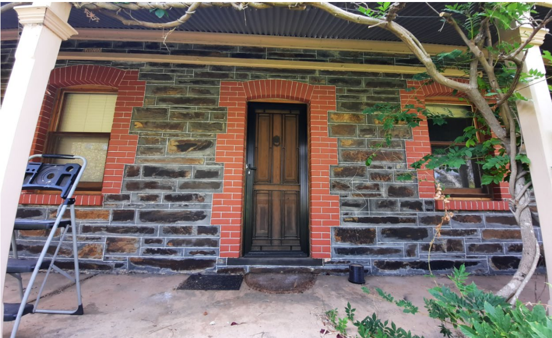
Primary west elevation of the mid-19 th century cottage at 17 Rowlands Hill Road; the matching bluestone to later additions could suggest this elevation was reconstructed at a later date (GGA, 2022)
