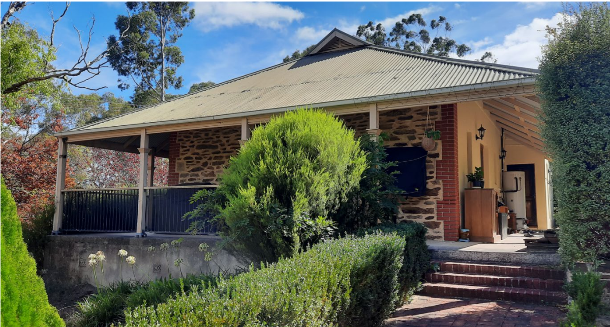
South elevation of c.late-19 th century additions looking north (GGA, 2022)
