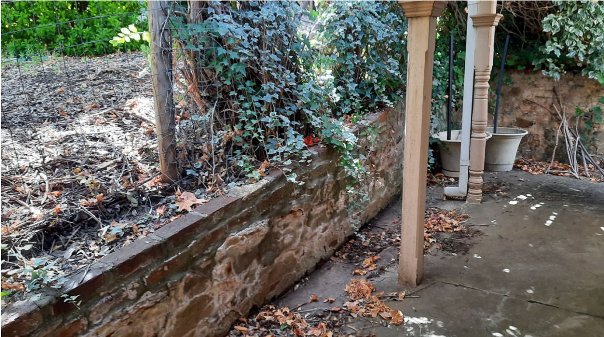
Extensive early retaining walls to the north-east of the mid-19 th century residence (GGA, 2022).
