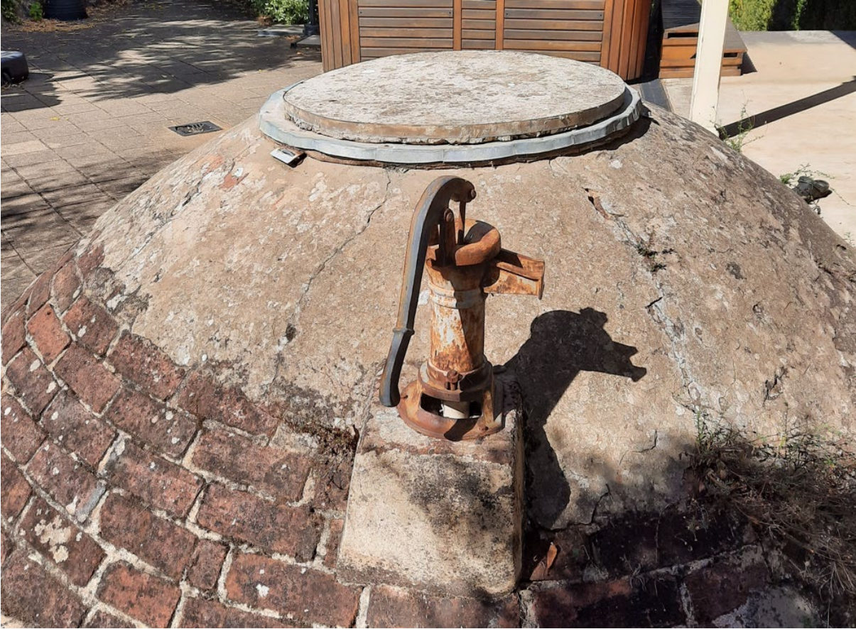
19 th century brick underground tank with original pump still intact, located to the rear gardens immediately east of the residence (GGA, 2022).
