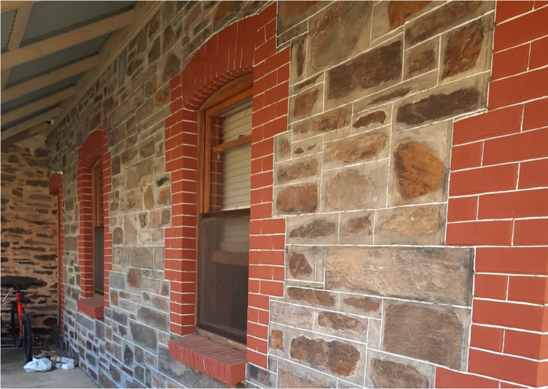
Later 19 th century additions immediately south of c.mid-19 th century cottage looking north; these additions appear to have undergone extensive alterations during the 20 th century, particularly to the eastern portion of the building (GGA, 2022)
