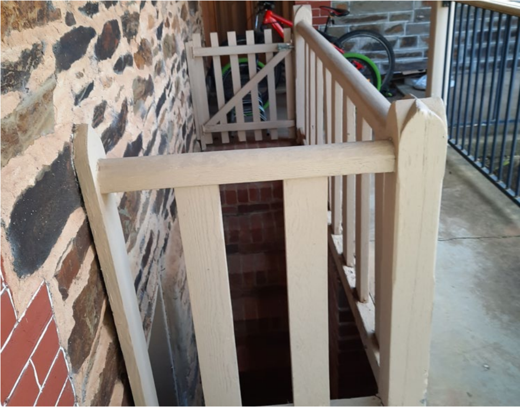
Brick stairs to the original cellars to the base of the c.mid-19 th century residence, looking east (GGA, 2022)
