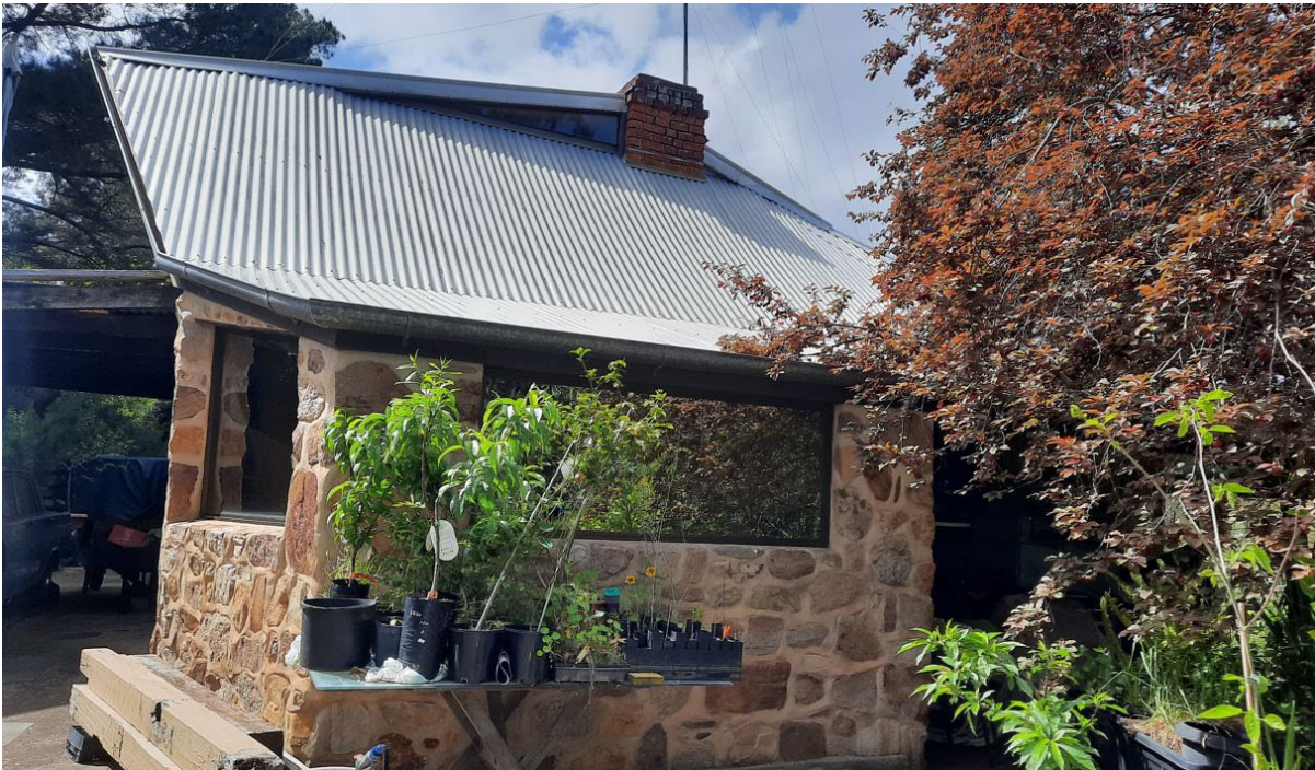
Late 20 th century additions to north elevation, retaining early brick chimney stack. (GGA, 2021).
