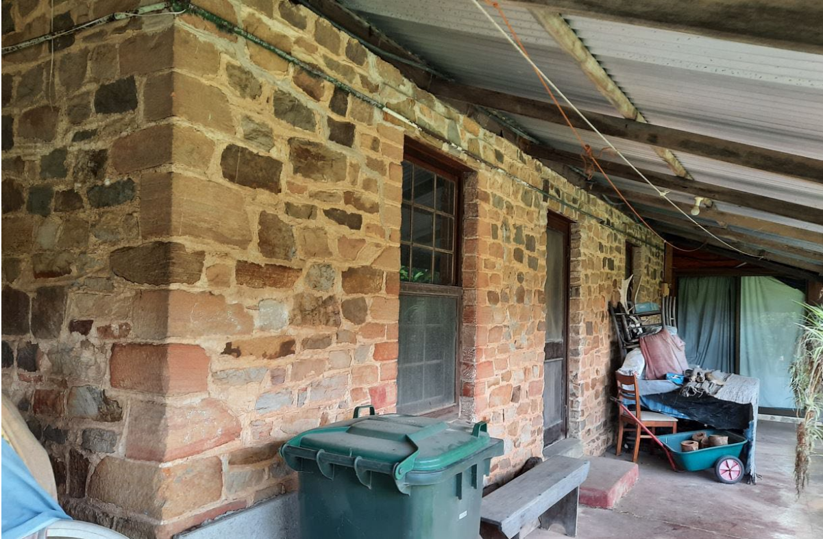
Early c.1850s masonry with original door and window openings, possibly early fittings (GGA, 2021).
