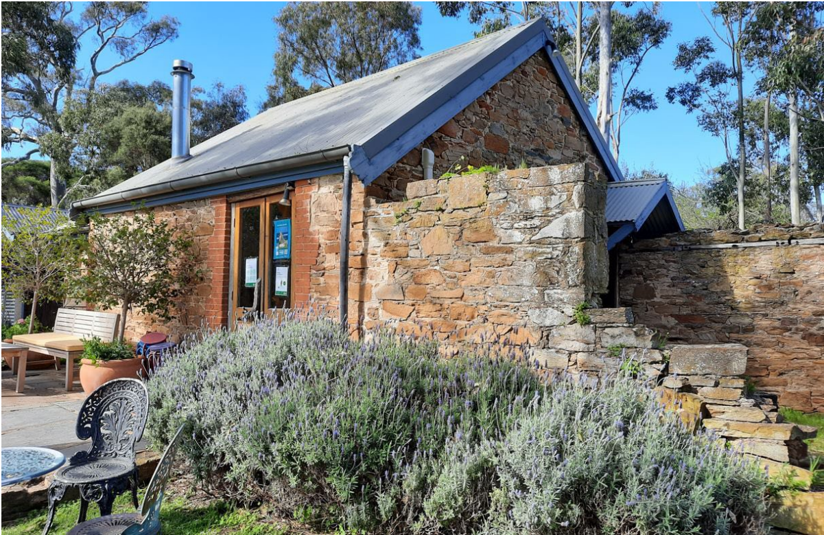
North elevation and ruinous walls of mid-19 th century outbuilding immediately east of former farmhouse with later corrugated steel roofing, chimney and timber-framed doors (GGA, 2021)
