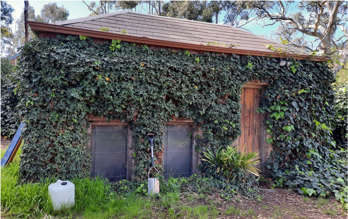
West elevation of split-level former dairy (GGA, 2021)
