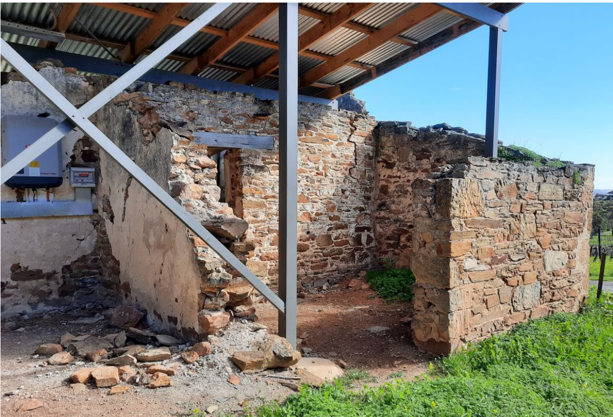
Surviving timber lintels and internal door and window openings to ruinous masonry outbuilding walls (GGA, 2021)
