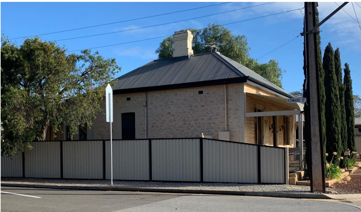
East elevation of 14 Malpas Street, Old Noarlunga (GGA, 2021)
